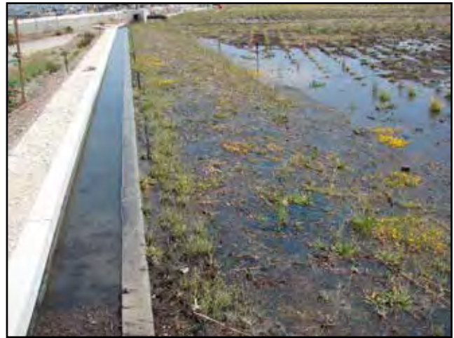
Stormwater Retention Basin
