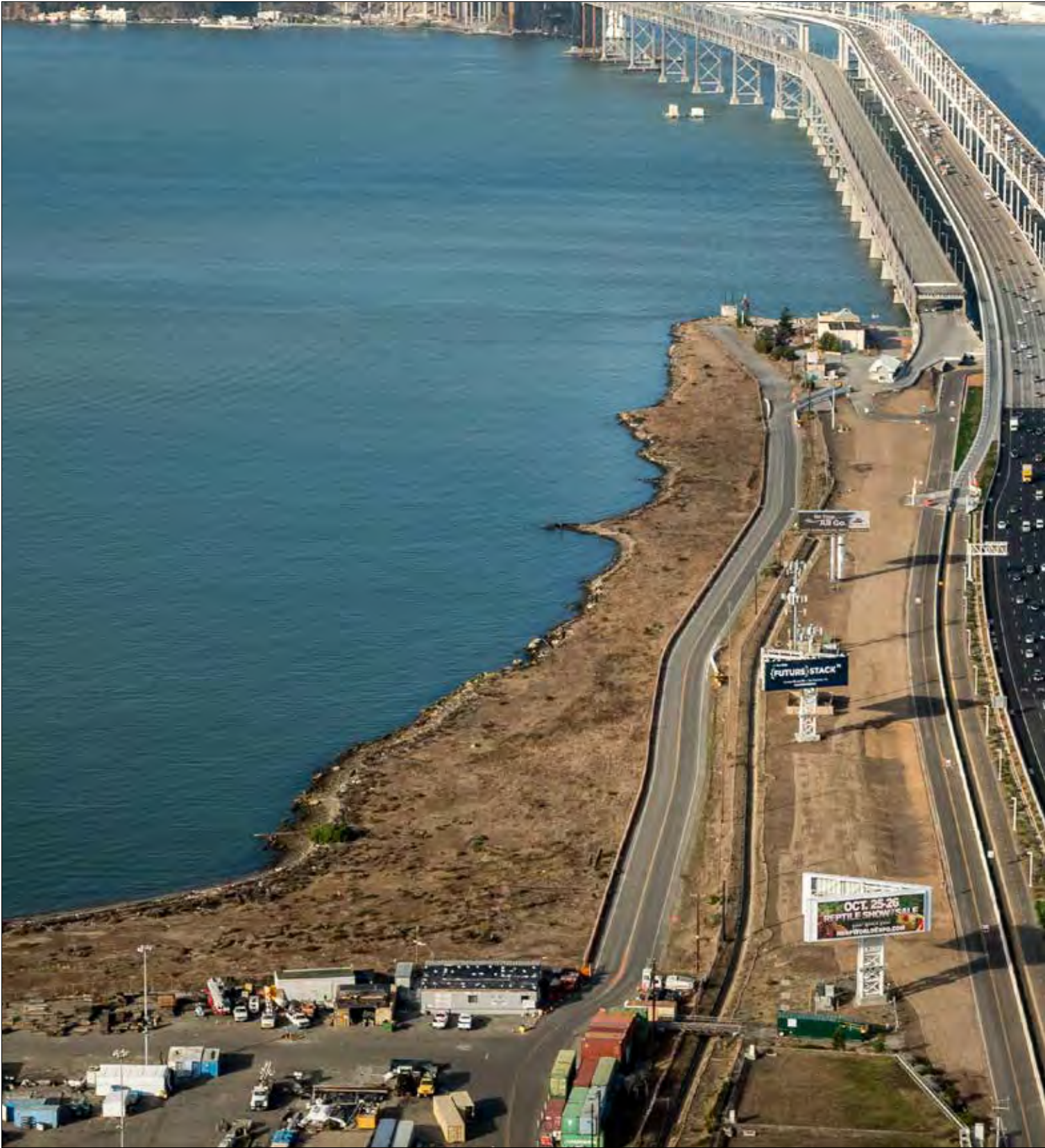
Aerial View of Oakland Touchdown Construction
