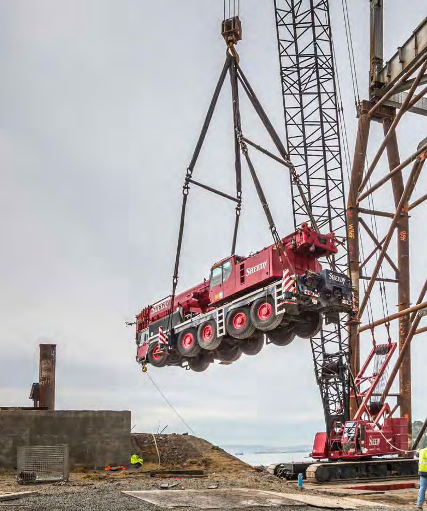
Lowering the Crane from the Dismantling Project
