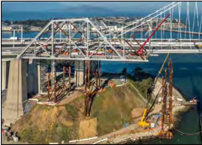
Superstructure Dismantling Progress
