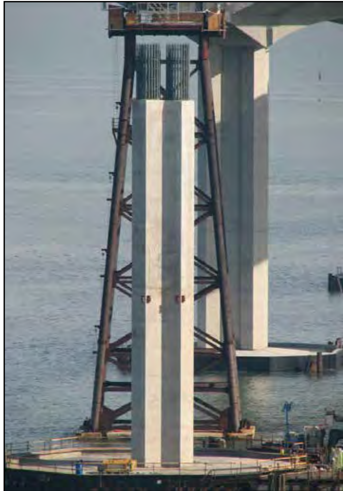
SAS Marine E2 and the Skyway Westbound Foundation and Columns
