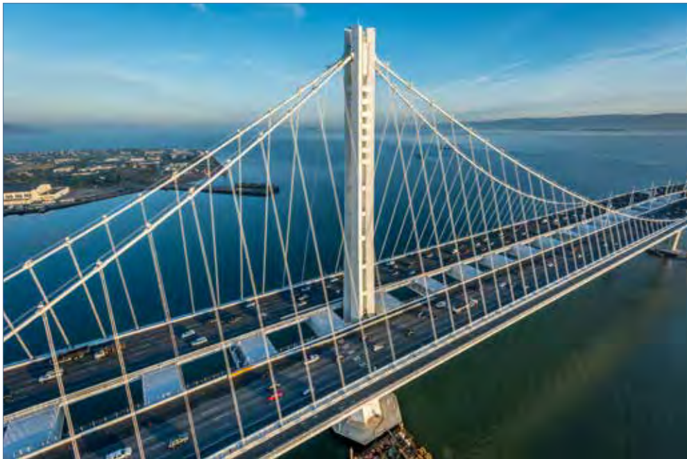
The Self-Anchored Suspension Bridge Span
