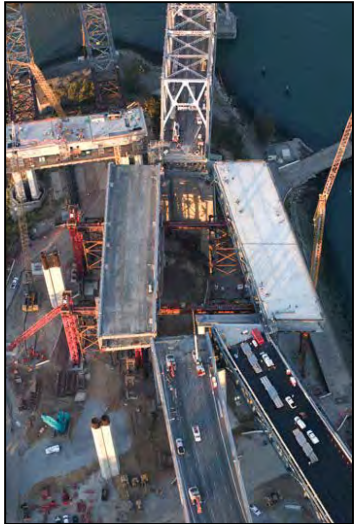
YBID East Tie-In Rolled in on Labor Day Weekend 2009
