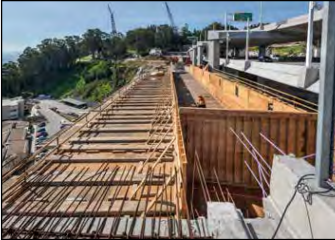
Self-Anchored Suspension Bridge Bike Path Construction
