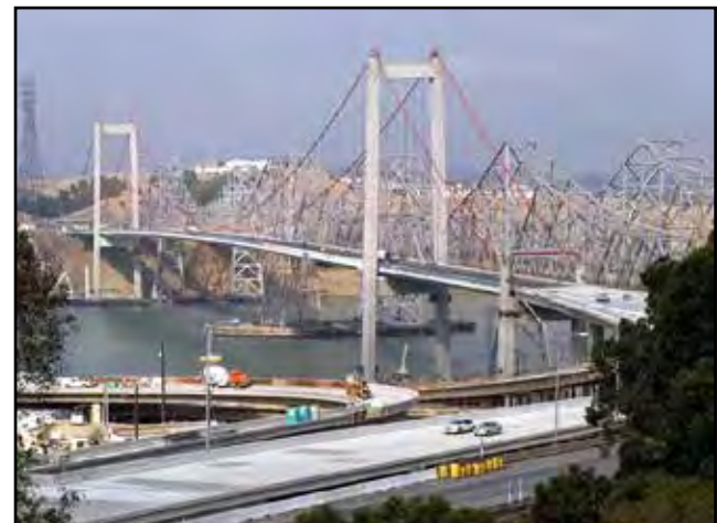
New Alfred Zampa Memorial (Carquinez) Bridge Soon after Opening to Traffic, with Crockett Interchange Still under Construction
