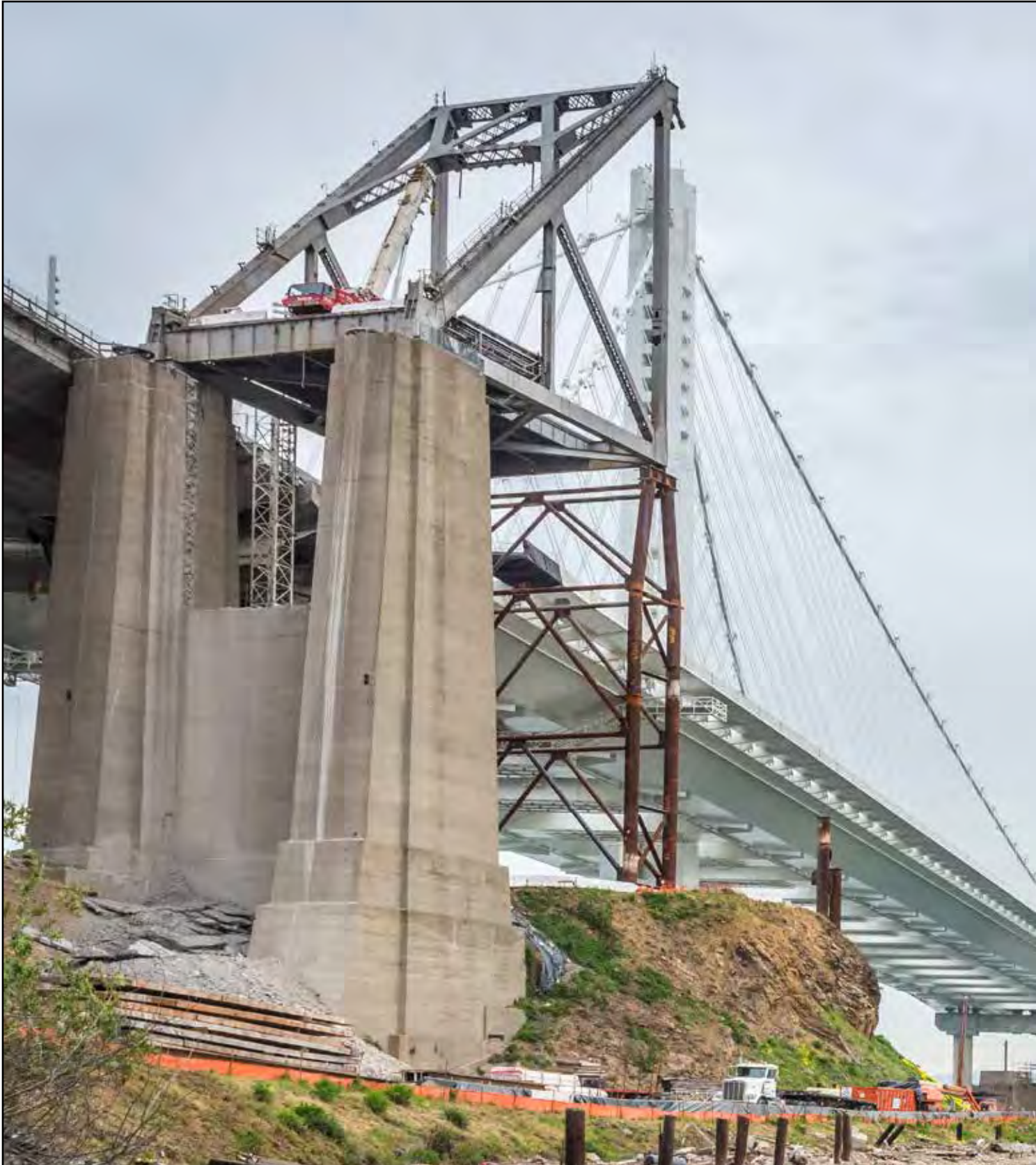
Yerba Buena Island Transition Structures Demolition Progress
