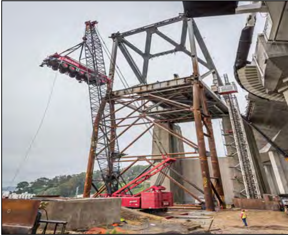
Lowering of Crane from Old San Francisco-Oakland Bay Bridge
