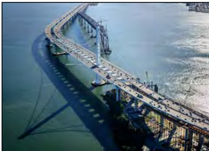
Superstructure Dismantling Progress
