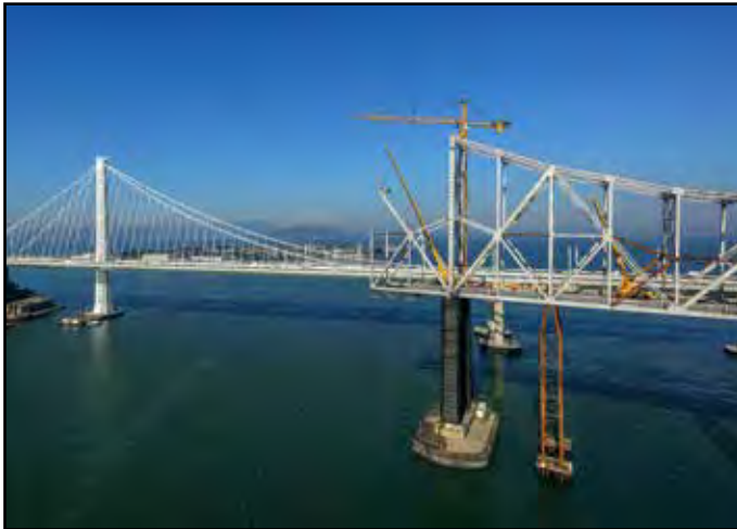
Superstructure Dismantling Progress
