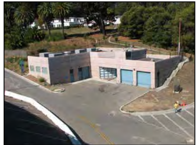
New YBI Electrical Substation
