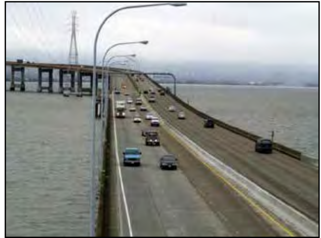
High-Rise Section of San Mateo-Hayward Bridge
