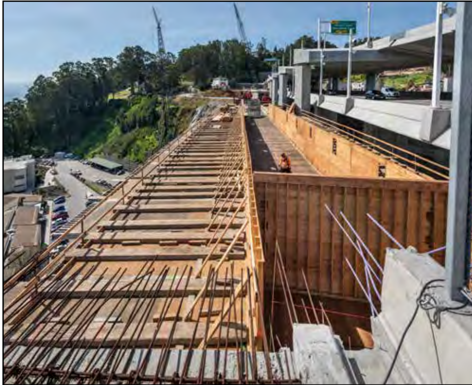
Bike Path Construction Progress
