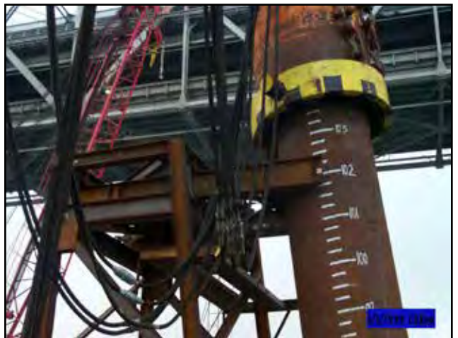
Battered Pile Installation Demonstration
