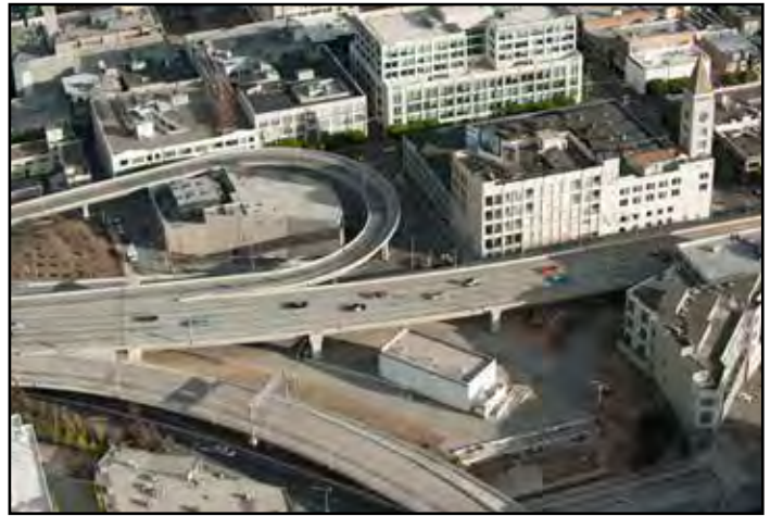
The San Francisco-Oakland Bay Bridge West Approach Overview
