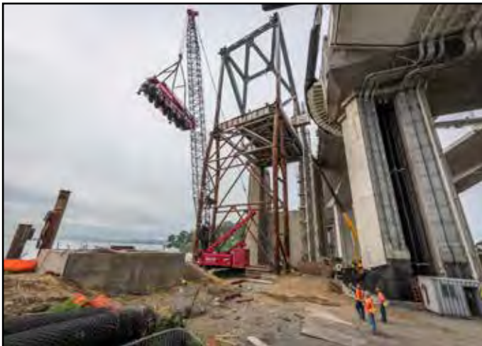
Self-Anchored Suspension Bridge Lowering Crane
