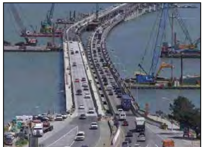
New Richmond-San Rafael Bridge West Approach Trestle under Construction
