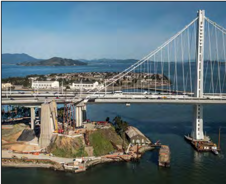
Aerial View of Dismantling Progress
