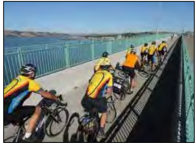
Benicia-Martinez Bridge Bicycle/Pedestrian Path
