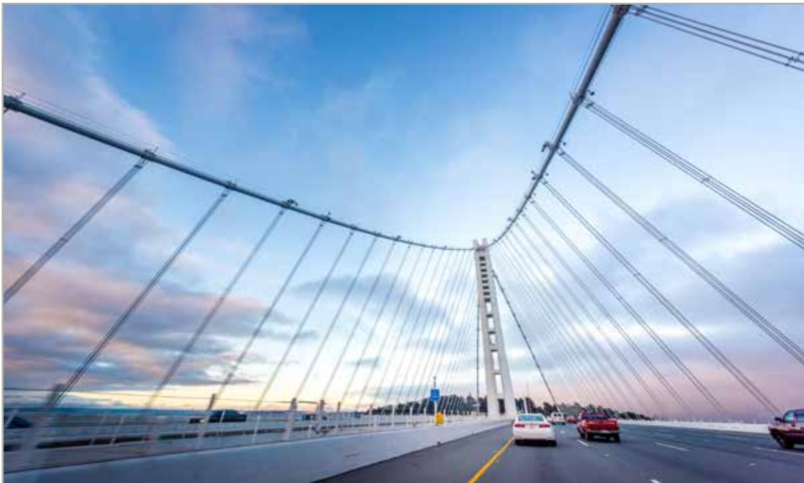
Self-Anchored Suspension Bridge Superstructure
