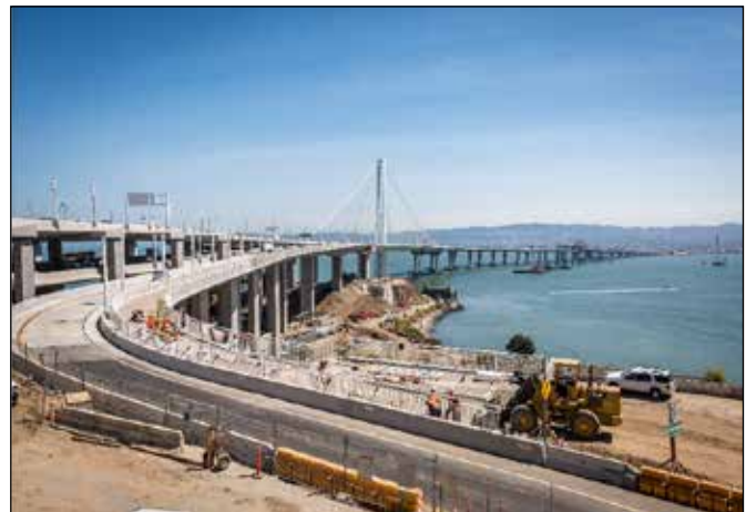
On-ramp and Bicycle/Pedestrian Pathway Progress
