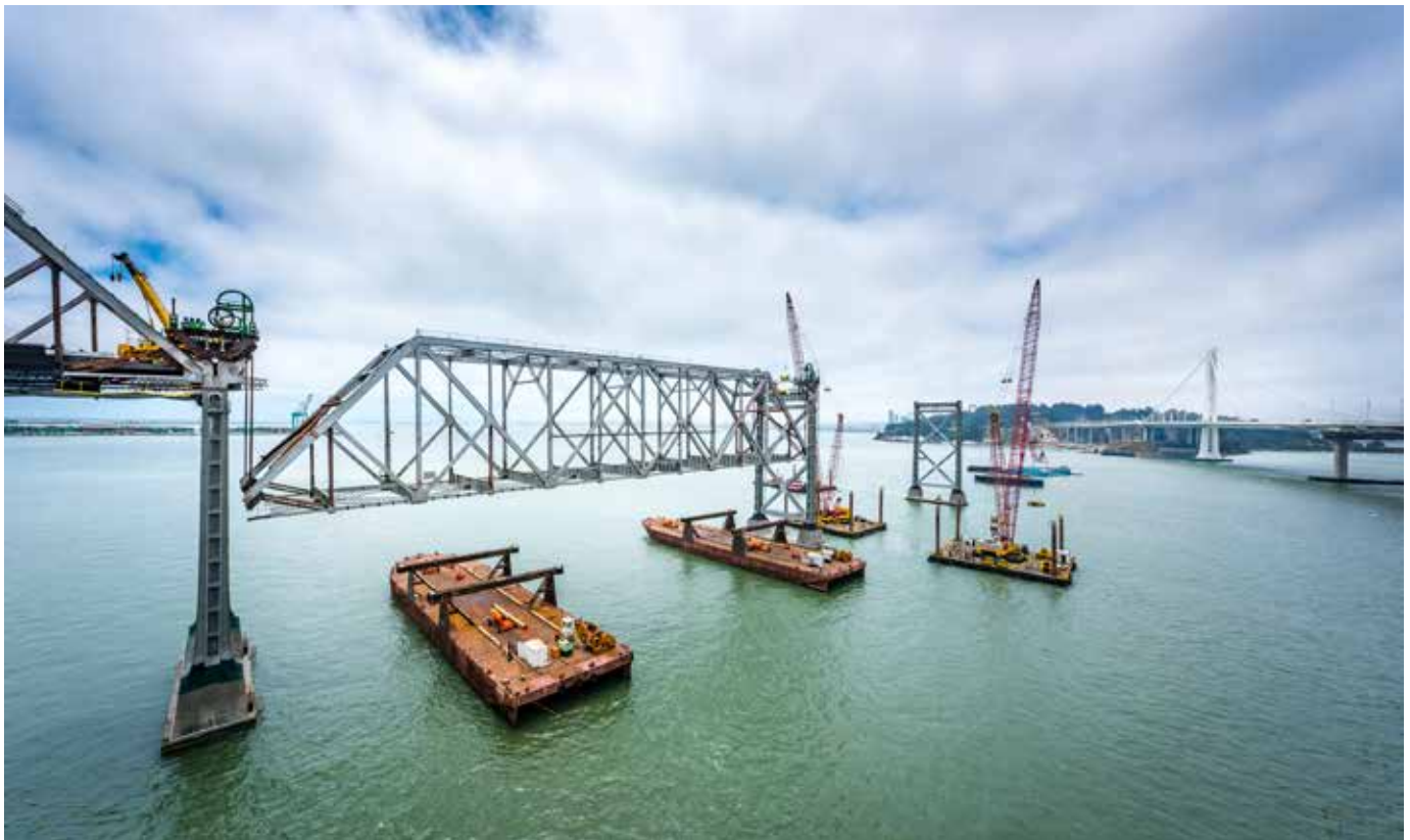
Dismantling Progress of the Former Superstructure
