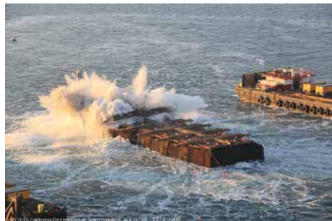
Pier E3 During Implosion
