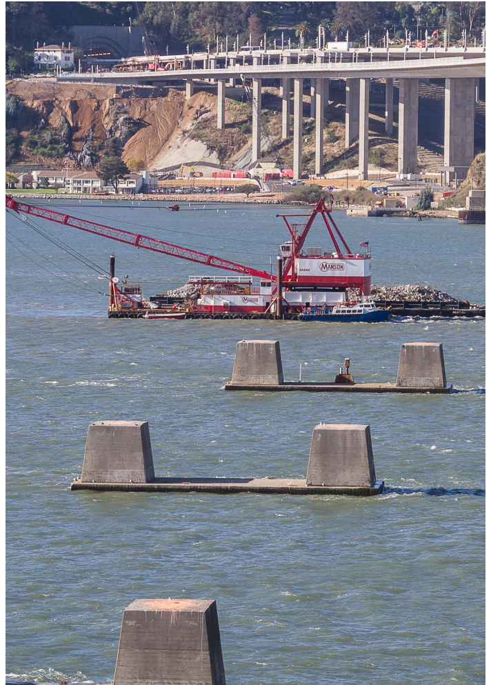
Marine foundation demolition.
