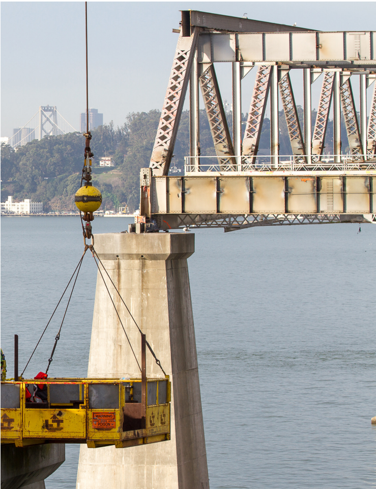
Demolition work on the original truss bridge.
