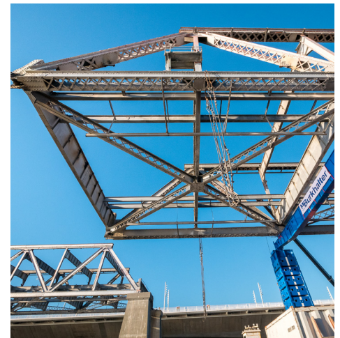
Lowering of 288' truss sections.
