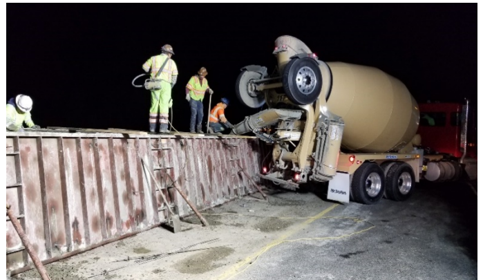
Barrier Rail Replacement I-880
