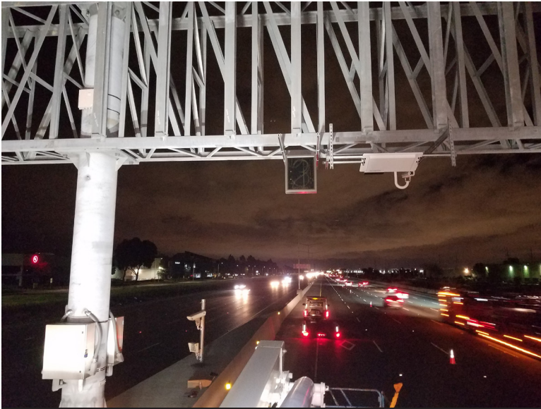
Installing toll system equipment including numeric enforcement beacons on I-880 gantries
