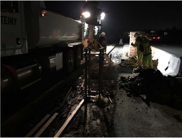
Electrical crews boring in the median barrier.
