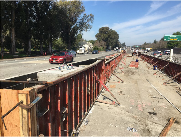
Preparing median barrier replacement for a concrete pour.
