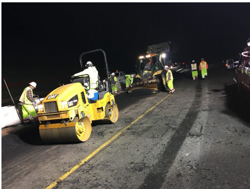
Construction crews pave a section of I-680.
