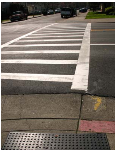
A crosswalk improved with an ADA truncated dome strip near the Mastick Senior Center.
