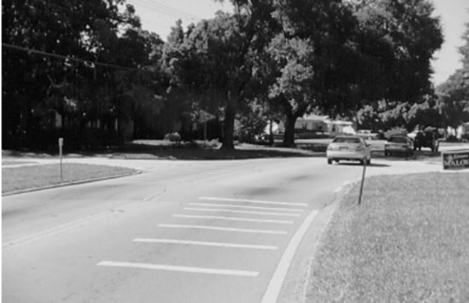
Figure A3-7 Transverse Marking
