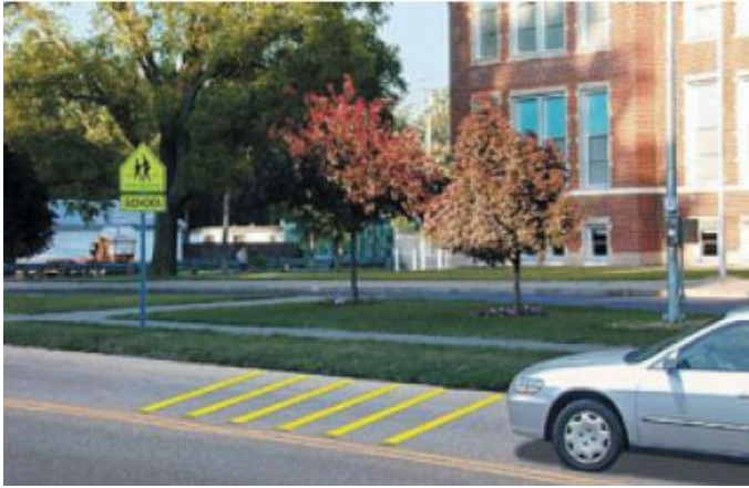
Figure A3-6 Rumble Strips
