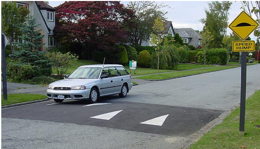
Figure A3-9 Concrete Speed Humps
