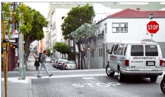
Figure 16. Raised crosswalk implemented at Minna and 7th streets is similar to the treatments recommended here.
