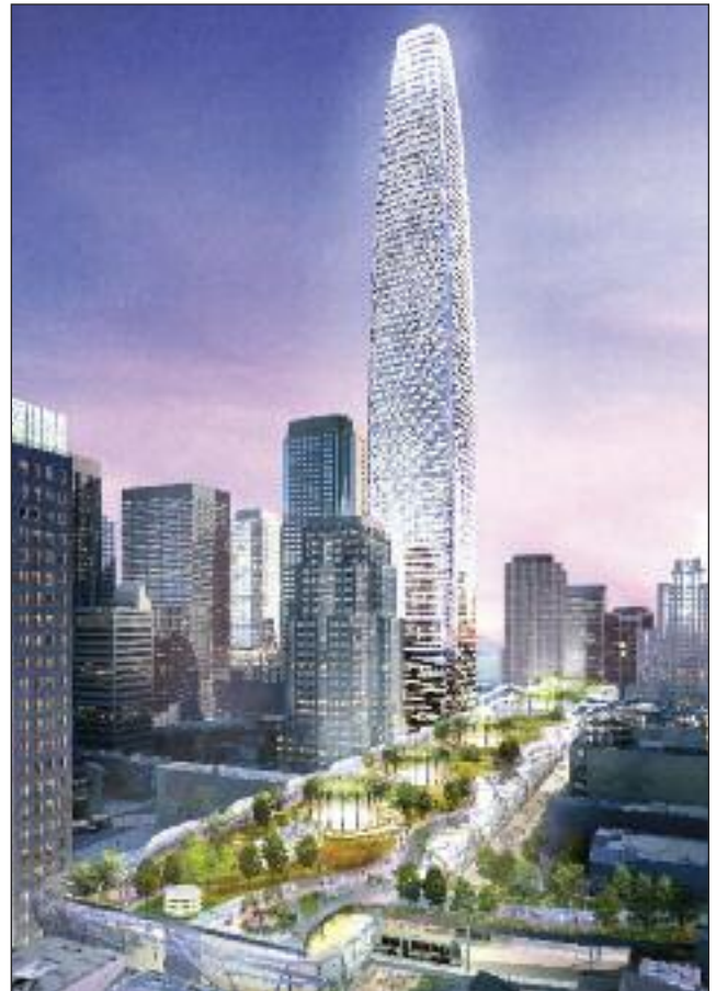
Rooftop garden at the new Transbay Transit Center in San Francisco
