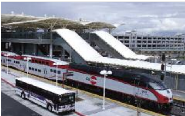
The existing multimodal BART/Caltrain station in Millbrae
