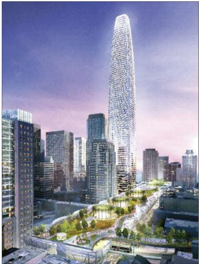
New Transbay Transit Center in San Francisco
