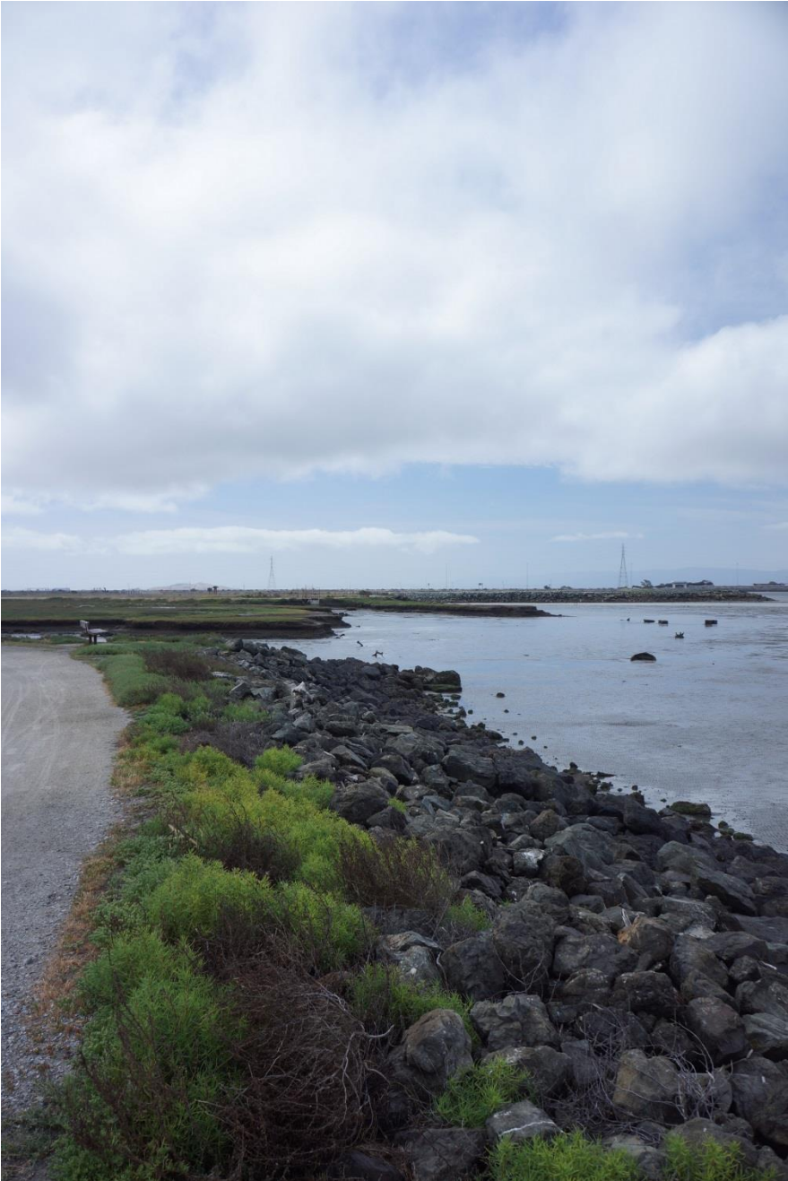
Hayward Focus Area – Shoreline Protection (Hayward Marsh looking South)
