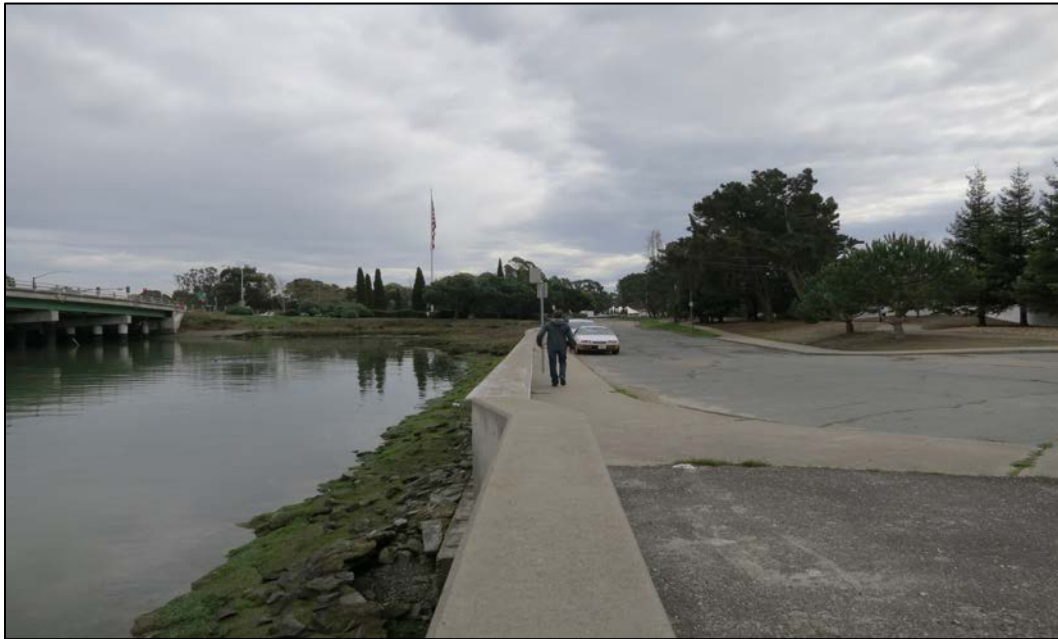
Figure 5. Site B - Veterans Court Seawall
