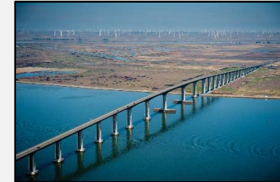
Antioch Bridge Opened 1926 Replaced 1978
