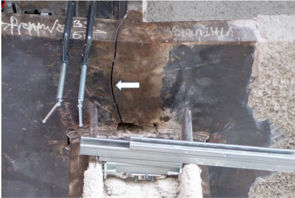
Figure 12 – North Girder – South Half - View Looking North (Photo: TJPA)
