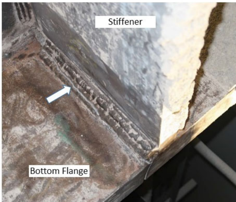
Figure 13 – North Girder – South Half - View Looking Northeast (Photo: TJPA)
