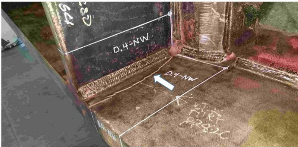
Figure 11 – North Girder – North Half – View Looking Southeast (Photo: TJPA)
