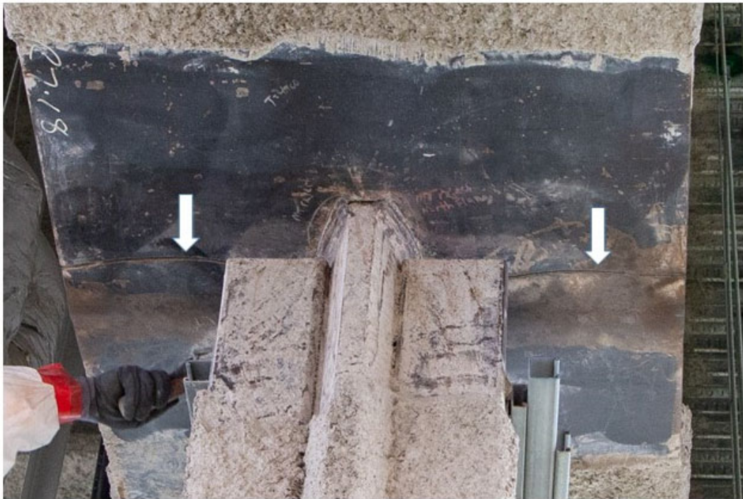
Figure 9 – North Girder - View Looking East (Photo: TJPA)
