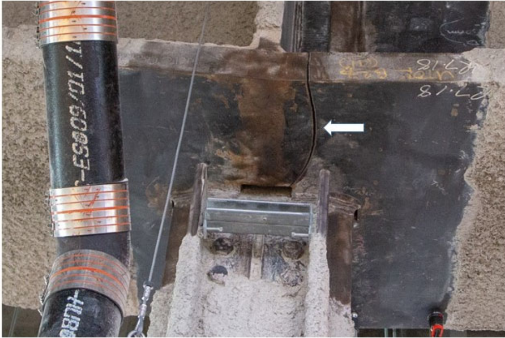
Figure 10 – North Girder – North Half - View Looking South (Photo: TJPA)
