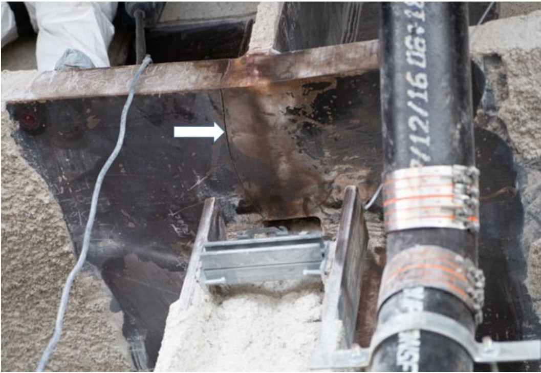
Figure 14 – South Girder – South Half - View Looking North (Photo: TJPA)
