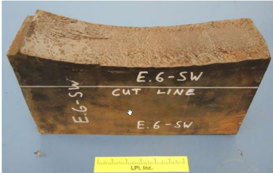
Figure 18 – Fracture Surface – South Half of South Girder (Photo: LPI Report)
