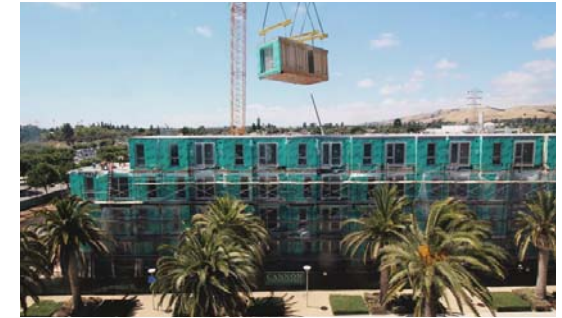
Union City; Modular Construction of Union Flats*
