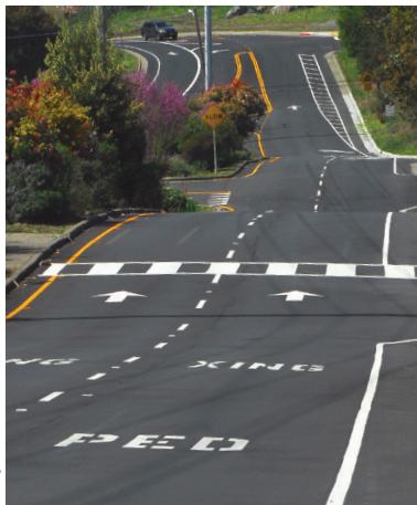
El Cerrito streets have had a major makeover, funded in part by revenues from a voter-approved sales tax.
