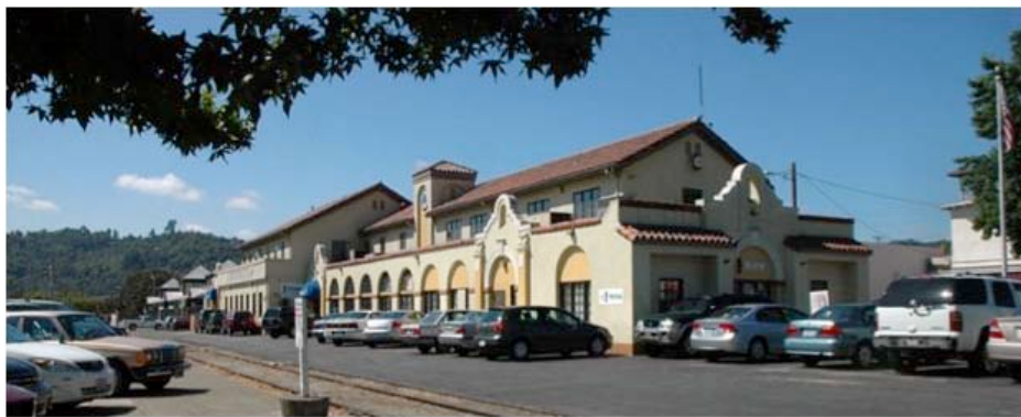
Whistlestop Building - Former Train Depot
