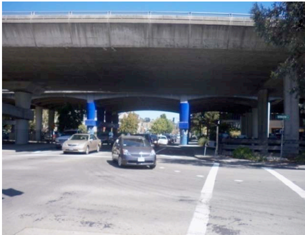
Crosswalk at the south leg of the Third Street / Hetherton Street intersection; note the double-left turn movements that must yield to pedestrians
