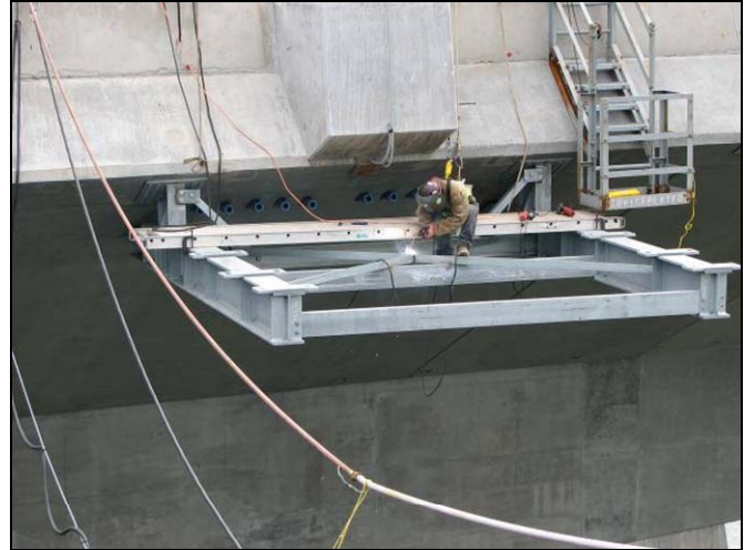
Skyway Erecting the Service Platform
