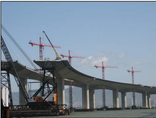
Skyway Looking East (one)
