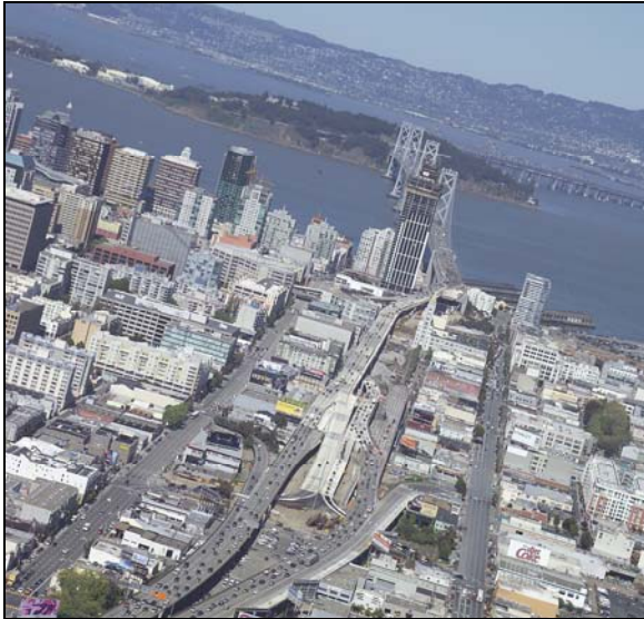
Aerial view of West Approach
