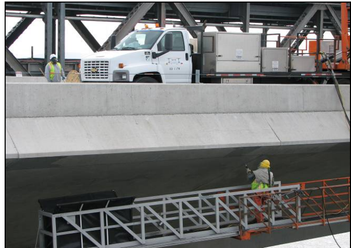
Skyway Sandblasting the Bridge Soffit
