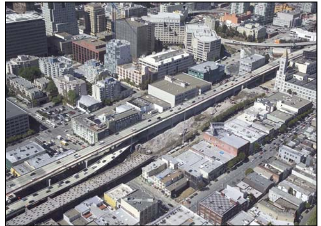
West Approach Overhead View of the newly opened SD60 Ramp & the Old Eastbound 80 Structure
