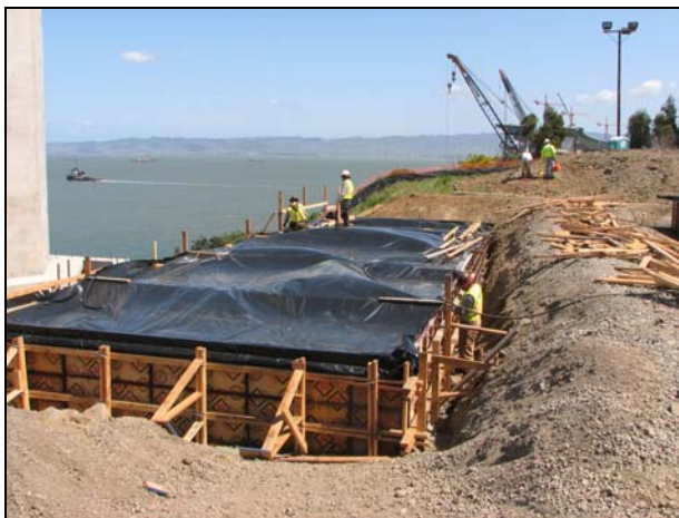
W2 - Preparation for Falsework Erection (one)
