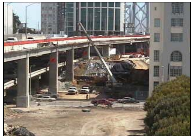
West Approach Demolition Upper deck Westbound
