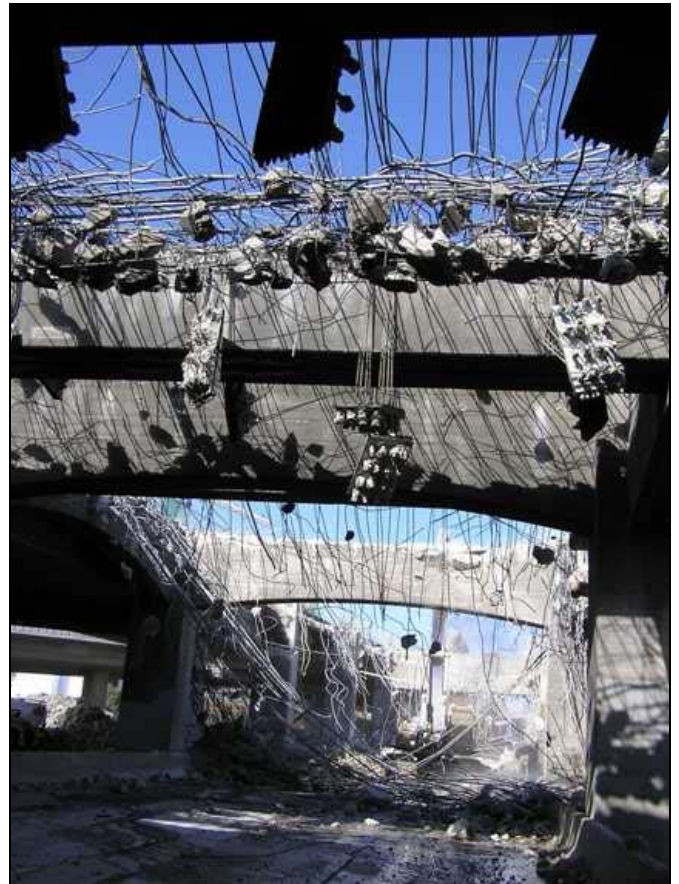
West Approach demolition
