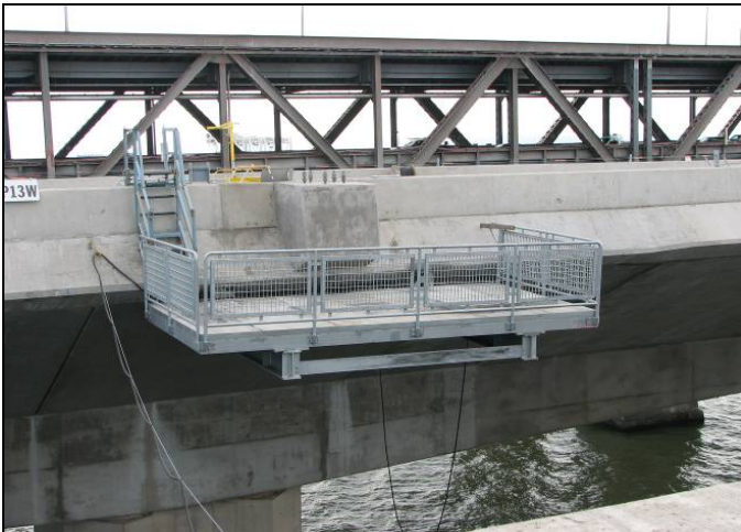
Skyway Erected Service Platform
