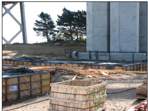
W2 - Preparation for Falsework Erection (two)
