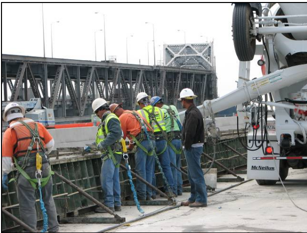
Skyway - Pouring Concrete Bridge Barrier
