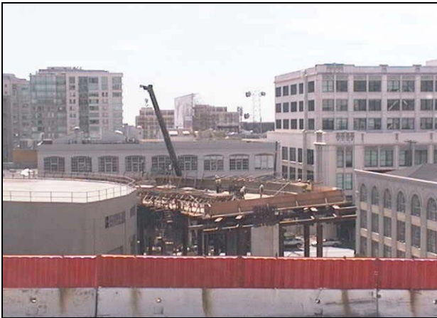
West Approach New Harrison Off-ramp Falsework
