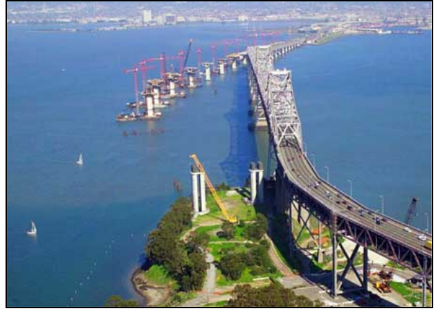
Footings and Pier Columns for Bent 48
