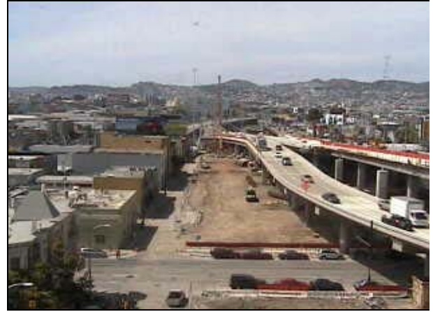
West Approach Demo Upper deck Westbound (two)
