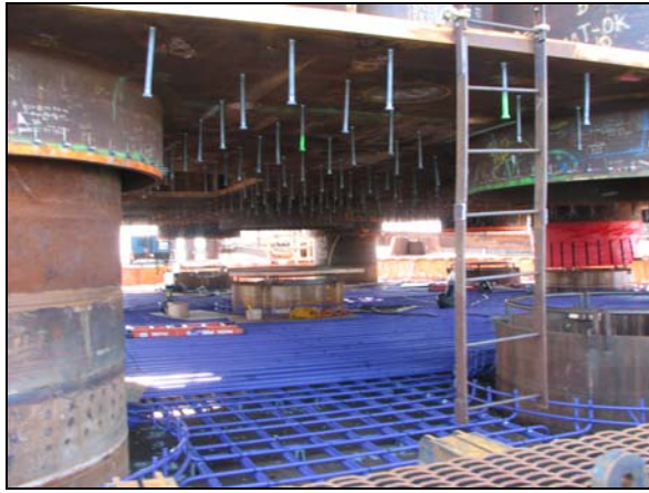
T1 - Bottom Slab Concrete
