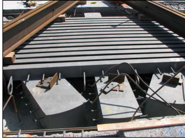
Skyway Expansion Joint Installation
