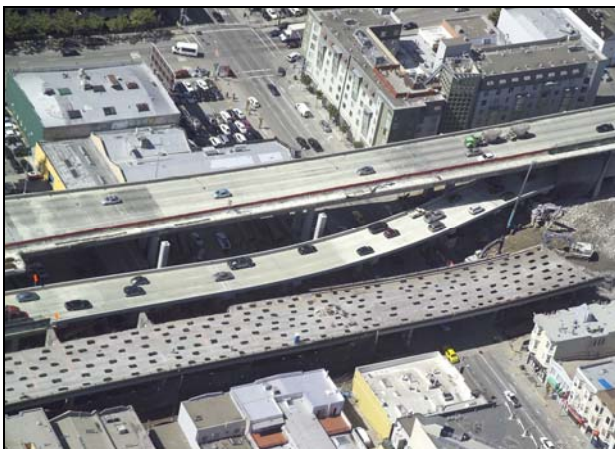
West Approach Overhead View of the newly opened SD60 Ramp & the Old Eastbound 80 Structure (Wider View)
