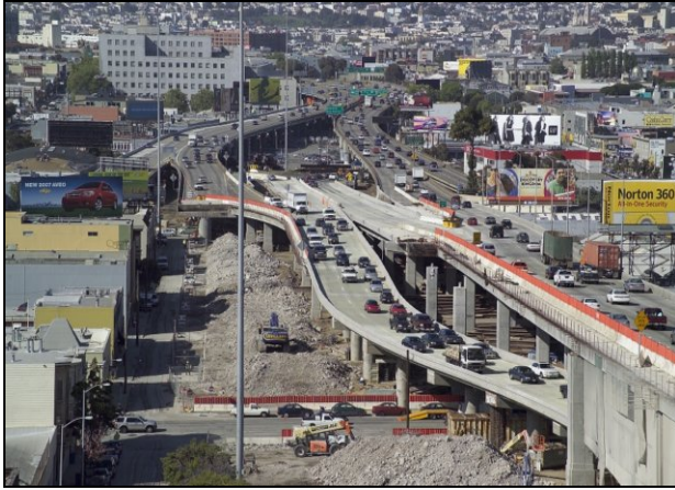
West Approach Demo Upper deck Westbound (one)
