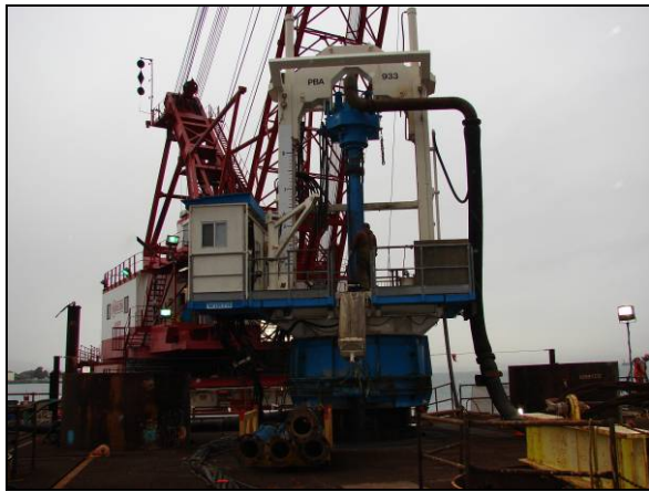
Rock Socket Drilling in Pile # 4 at T1
