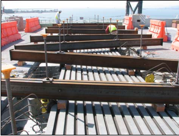
Skyway Eastbound Hinge BE Expansion Joint
