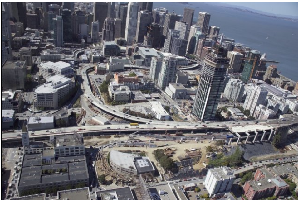
West Approach Overhead View
