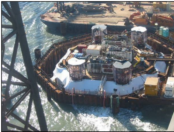
E2 Prepared and Sheltered for pile head connection welding
