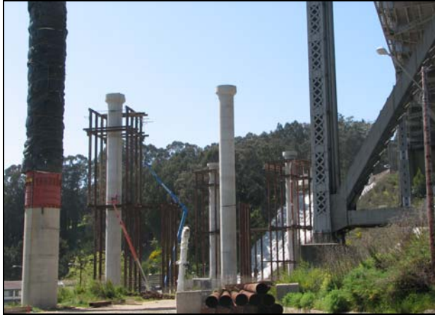
Viaduct Bent Cap Falsework
