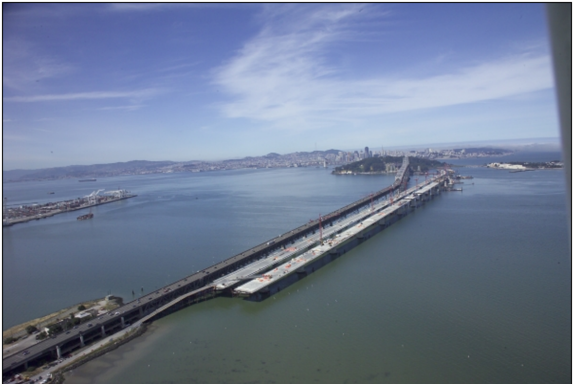
Aerial view of Skyway construction
