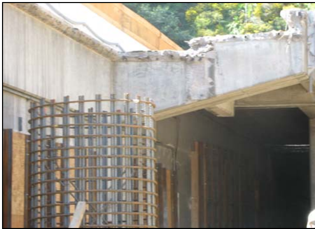
WTI Phase 1 - Demolition of North Overhang
