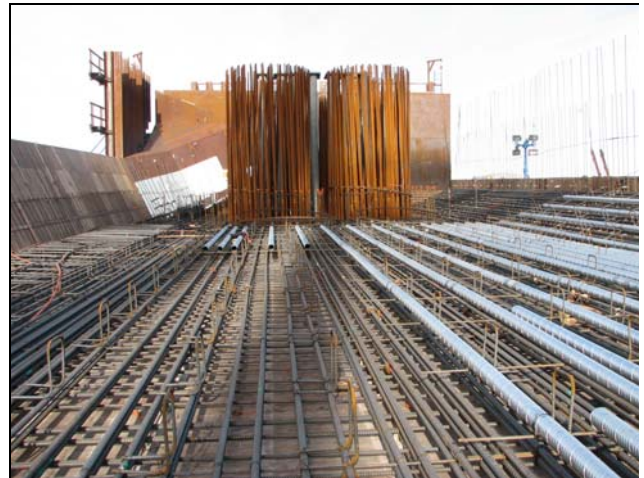
SAS - W2 Steel Reinforcement
