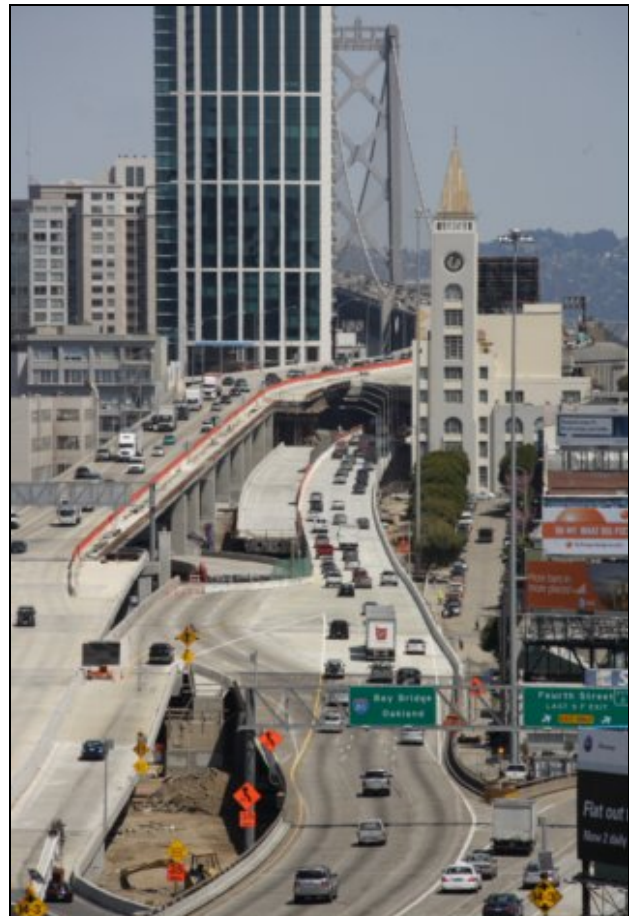
West Approach – Opened to Traffic April 12, 2008
