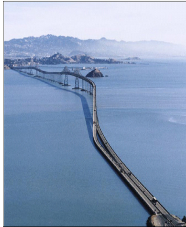
The Richmond-San Rafael Bridge
