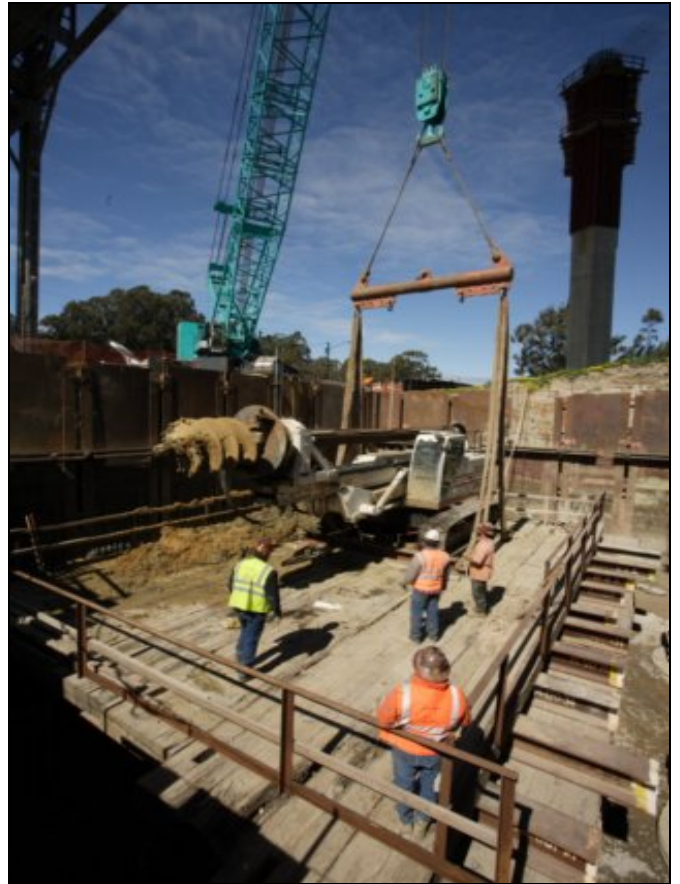
YBID - Bent W6 Construction YBI Advanced Work
