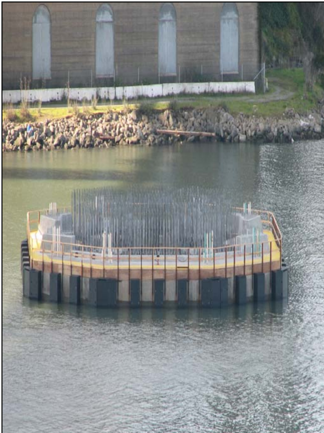
E2-T1 - Completed T1 Footing
