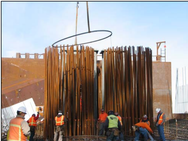
SAS - W2 Steel Reinforcement
