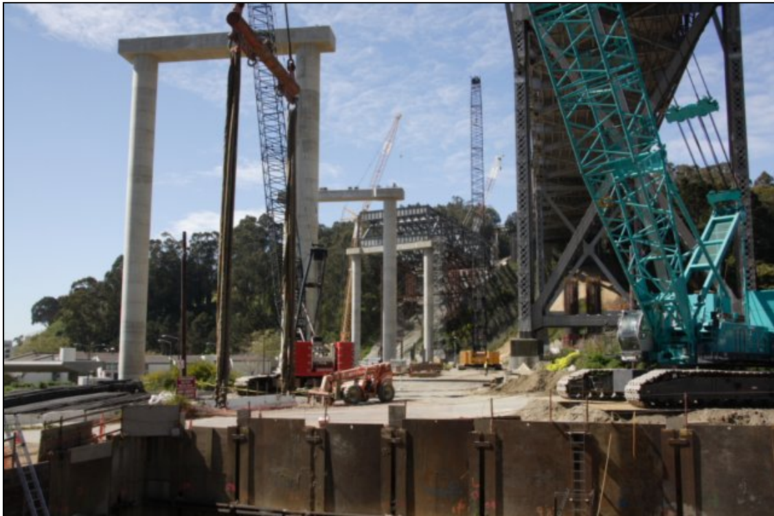
Skid Bents with YBID in the Background
