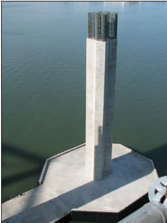
SAS E2-T1 - Completed E2 Column Westbound
