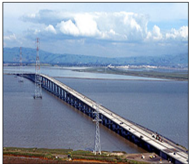
The Dumbarton Bridge
