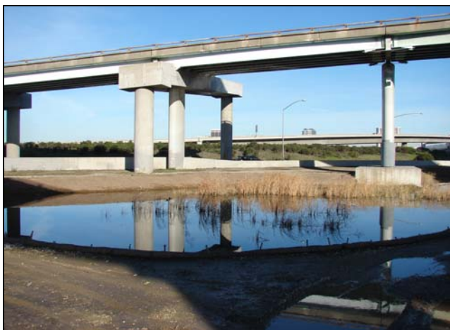
Stormwater - Forebay Location 5
