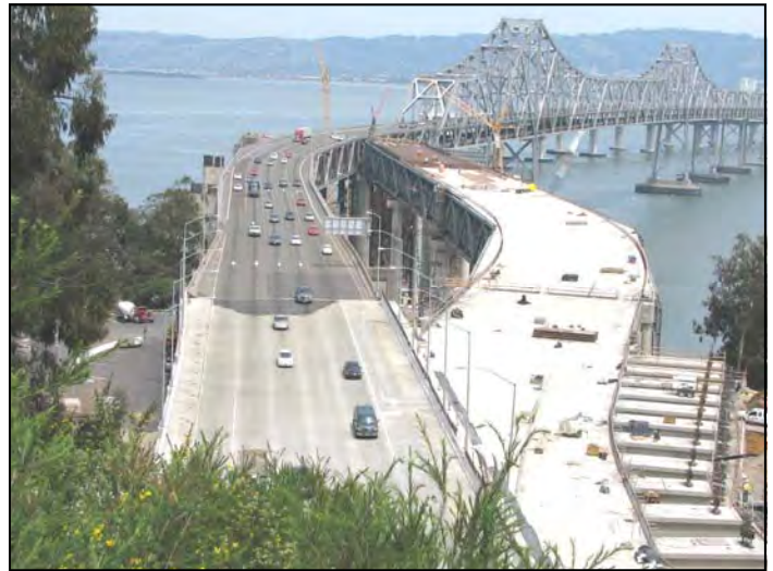
Current Progress on Detour Structure
