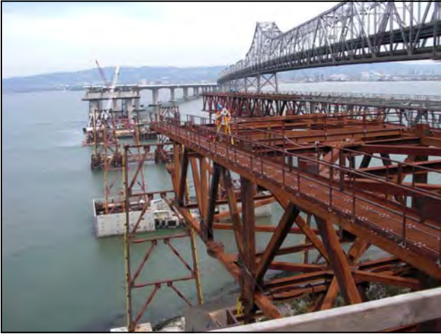
Temporary Support Structures for the SAS
