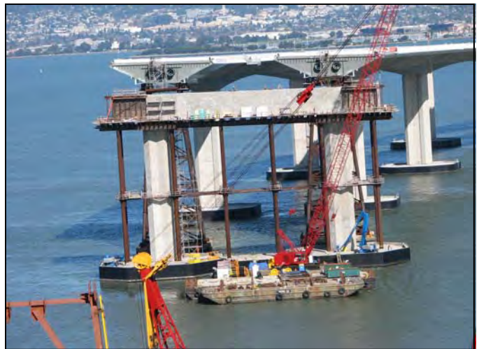
Nearly Completed Cross Beam at Pier E2
