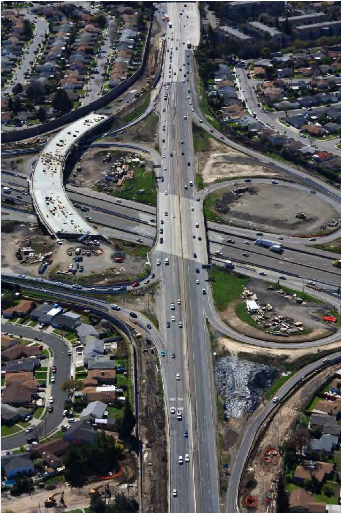
Overview of 92/880 Interchange
