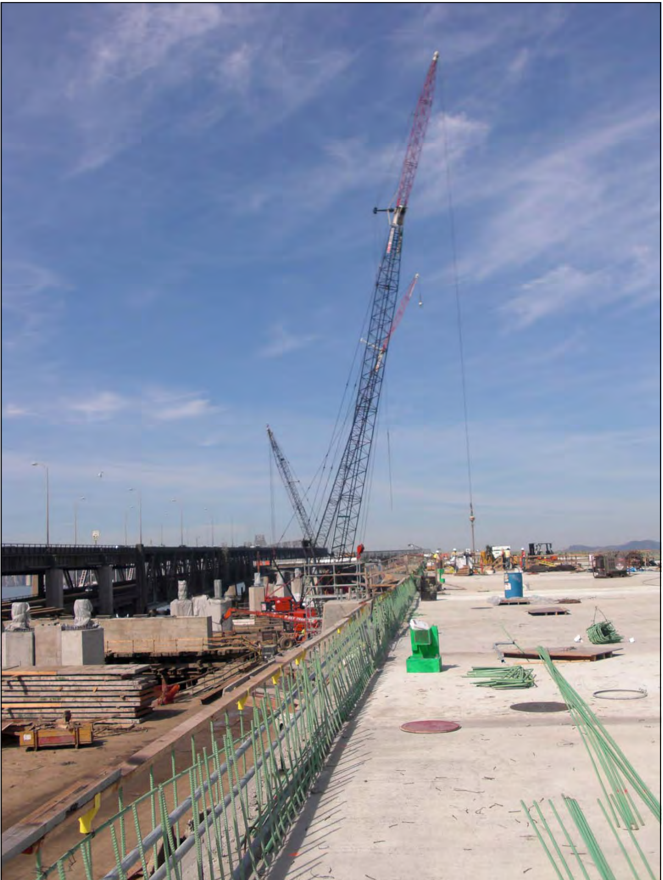
OTD #1 Westbound Barrier Lighting Conduit and Poles Installation
