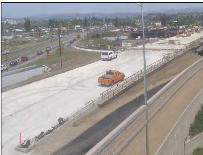
New East Route 92 to North Interstate 880 Direct Connector Under Construction
