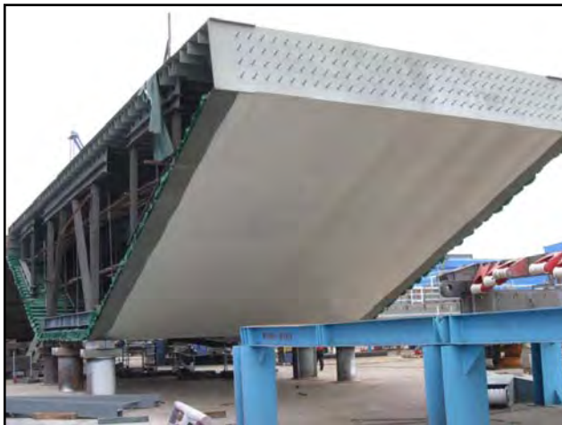
Painted Roadway Box Section Ready For Fit-up
