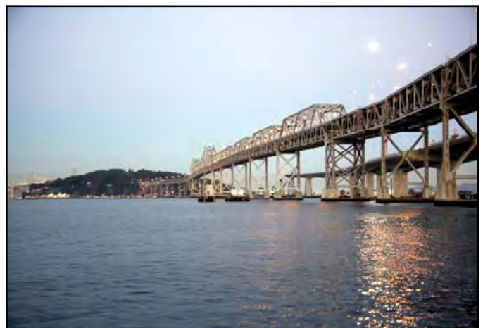
Existing East Span of Bay Bridge
