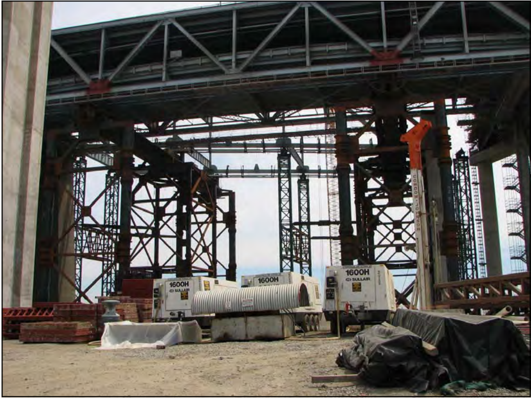
East Tie-in Skid Bent System Framing
