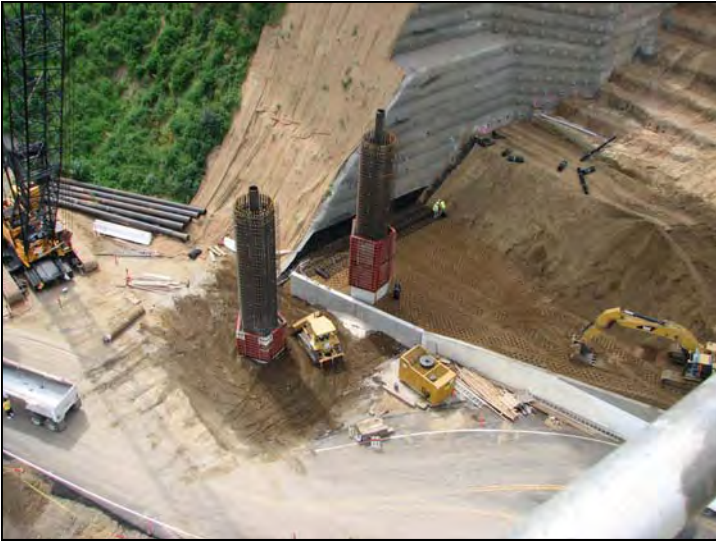
Soil Nail Wall
