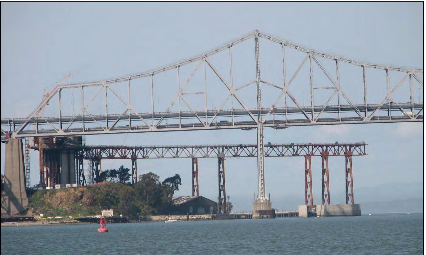
Temporary Support Structures Erected Behind Existing East Span
