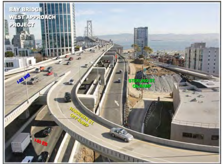
Recently Reopened Harrison Street Off-ramp
