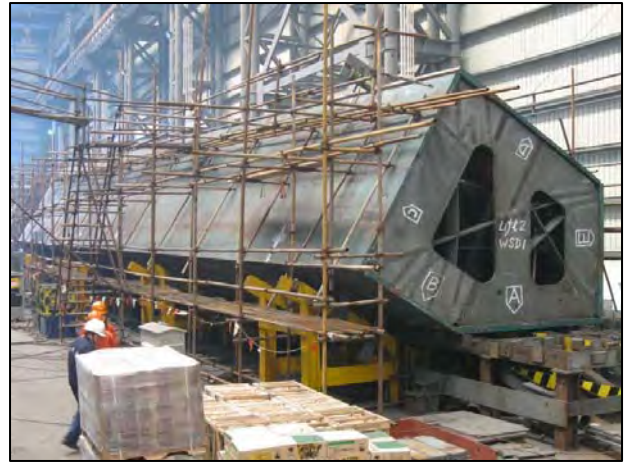
West Shaft, Lift 2 Assembly
