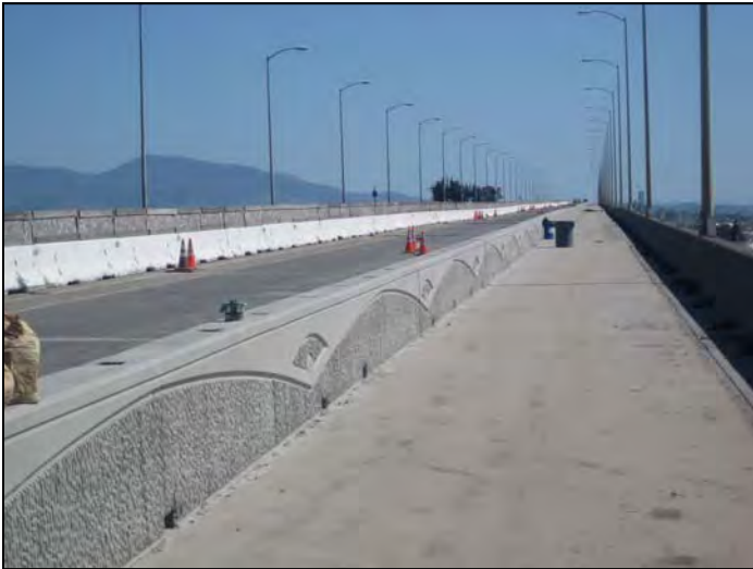
New Bicycle/Pedestrian Pathway on Benicia Martinez Bridge
