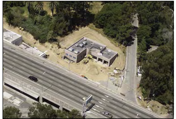
New YBI Electrical Substation
