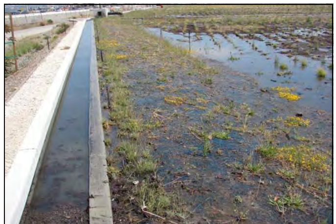
Storm Water Retention Basin
