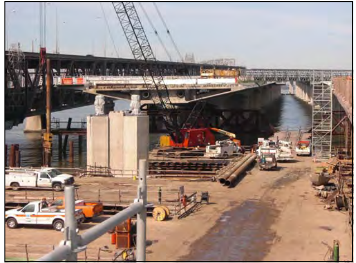
Oakland Touchdown #1 Pier Construction
