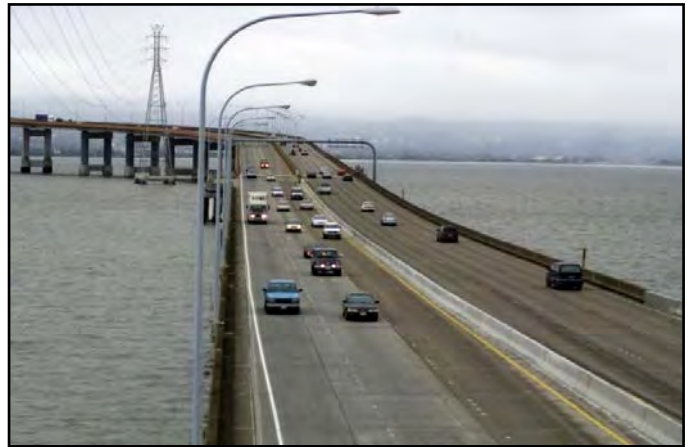
High-Rise Section of San Mateo-Hayward Bridge
