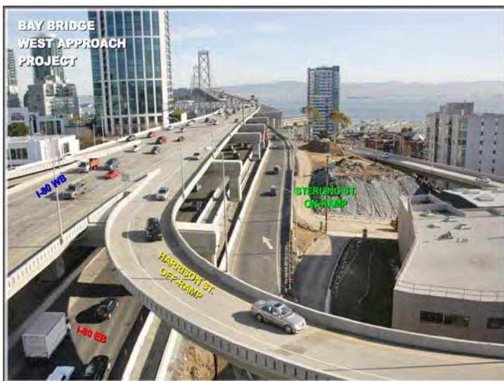
Recently Reopened Harrison Street Off-Ramp
