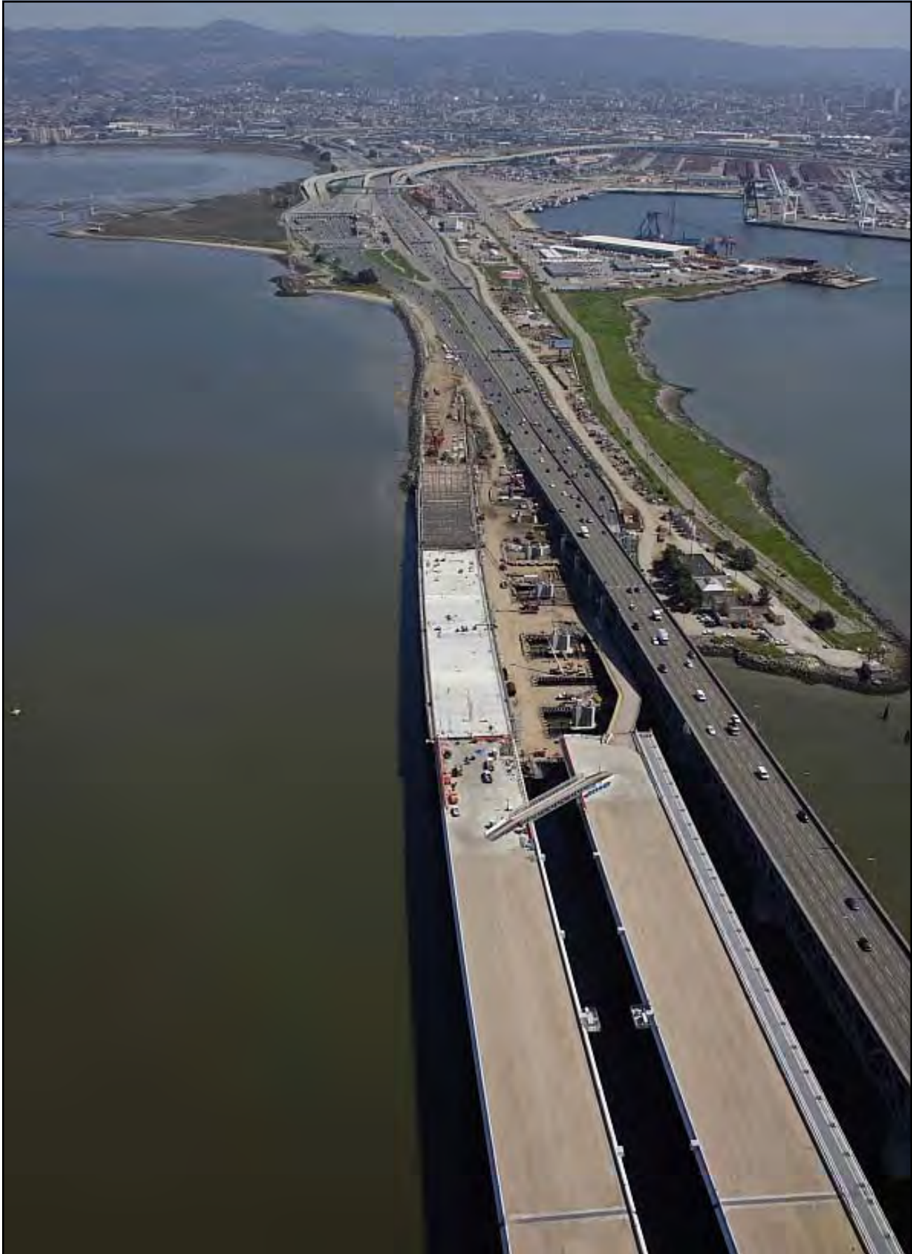
Oakland Touchdown under Construction with New Westbound Structure on Left
