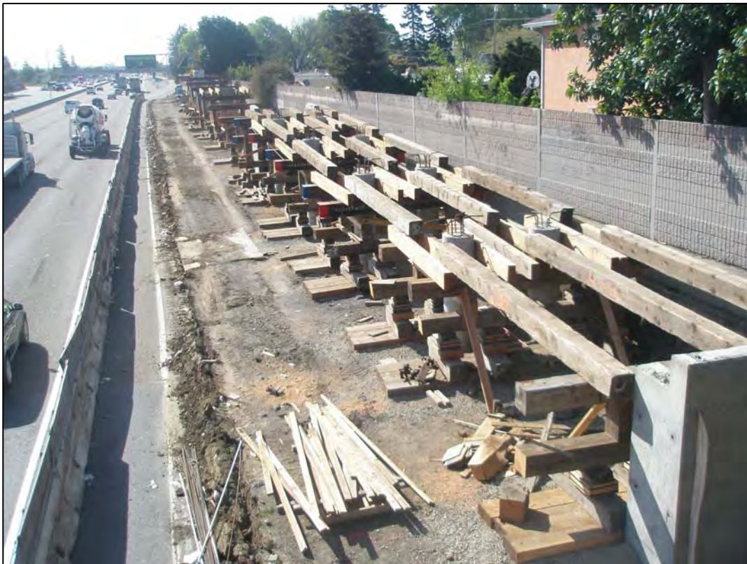
Work at Eldridge Avenue
