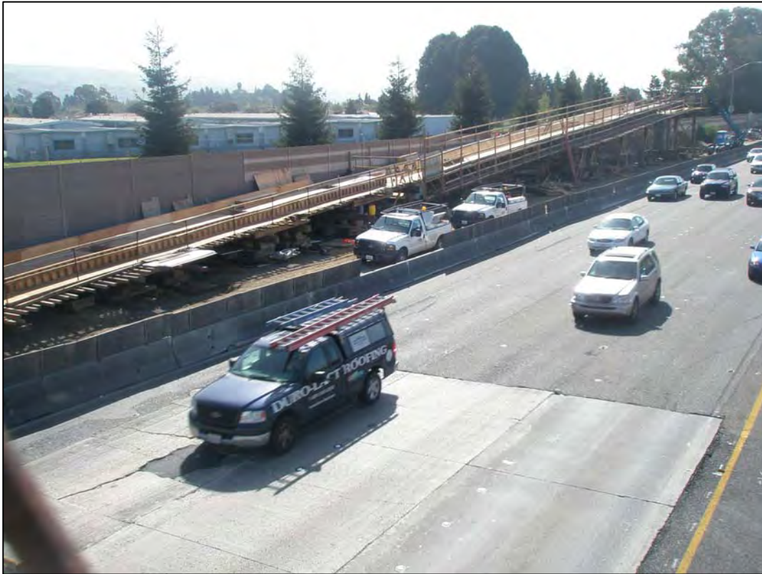
Work at Eldridge Avenue
