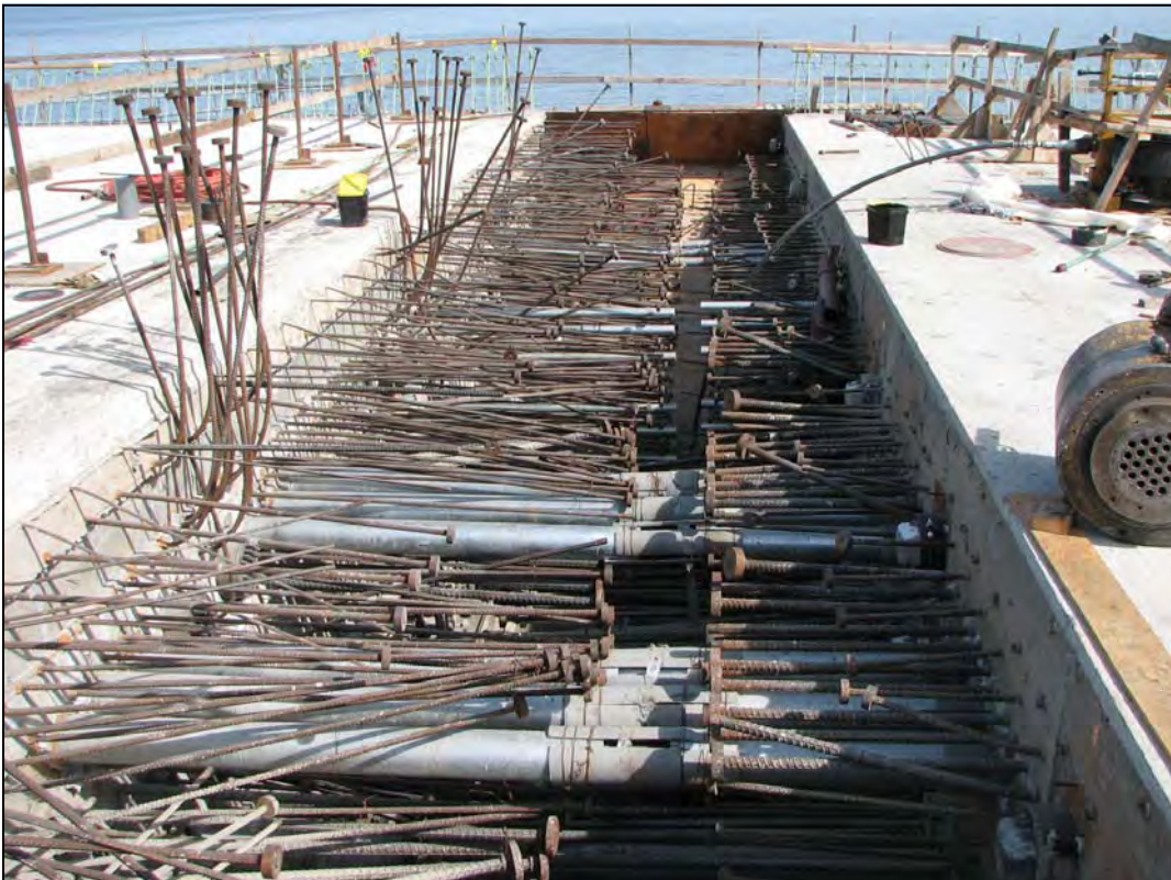
Completed Frame Two Pre-Stressing
