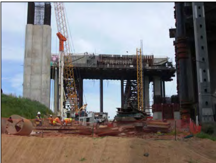
SAS W2 Cap Beam
