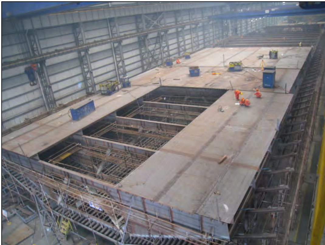
Overview of East Jig in Bay 14
