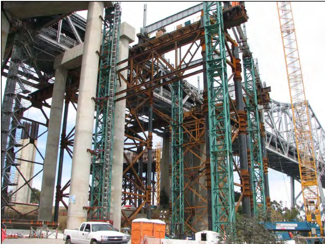
East Tie-in Skid Beams and Truss Supports
