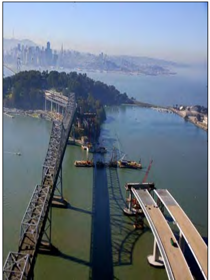
Western End of Completed Skyway
