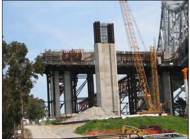
YBITS Advanced Foundation and Column Work
