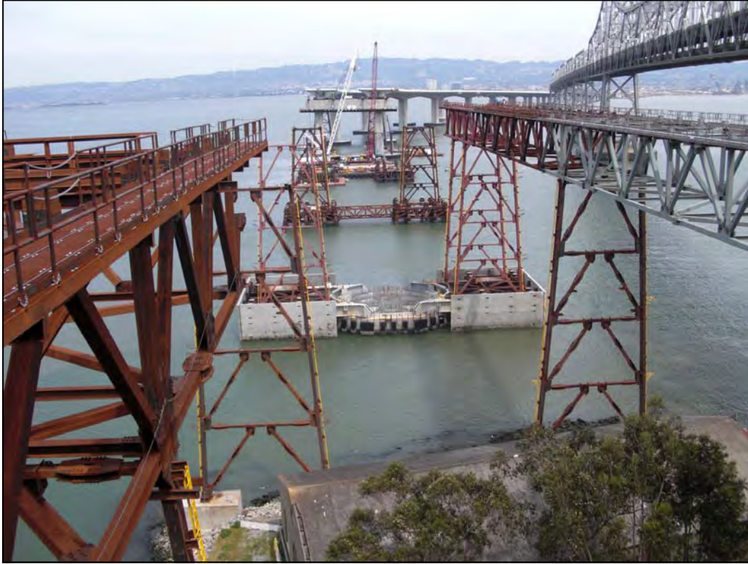
Temporary Towers Looking from W2 to the East
