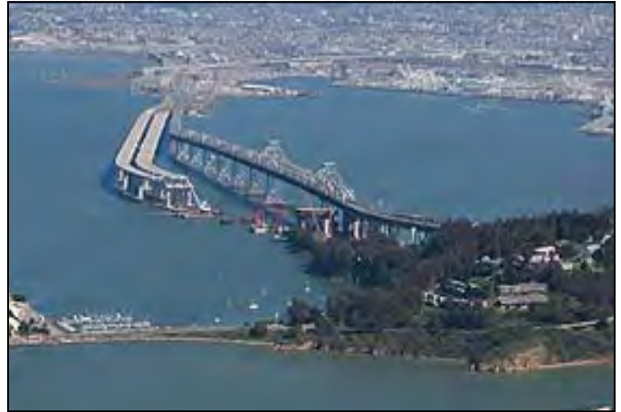
Completed Skyway Left of Existing East Span
