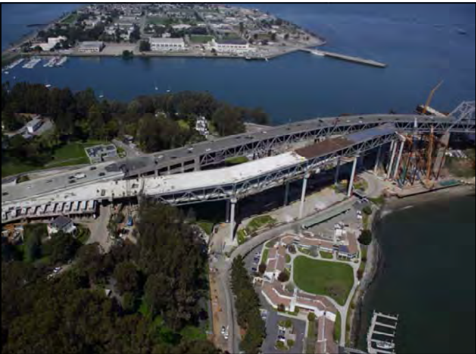
Yerba Buena Island Detour Structure Under Construction
