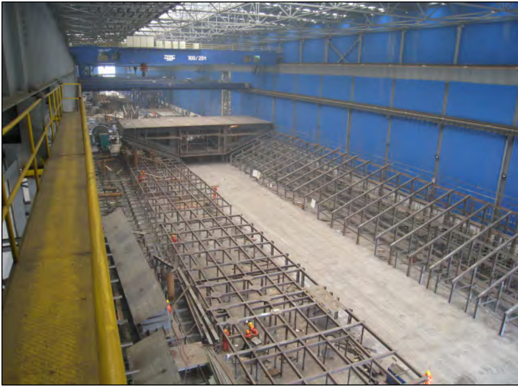
Overview of 1 BW Assembly in Bay 13
