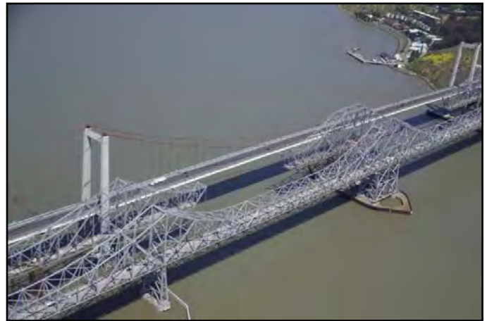
1958 Carquinez Bridge (foreground) with the 1927 Span (middle) under Demolition and the New Alfred Zampa Memorial Bridge (background)
