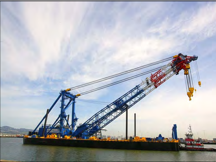
Shear-Leg Crane Barge Arrived in San Francisco Bay on March 12, 2009
