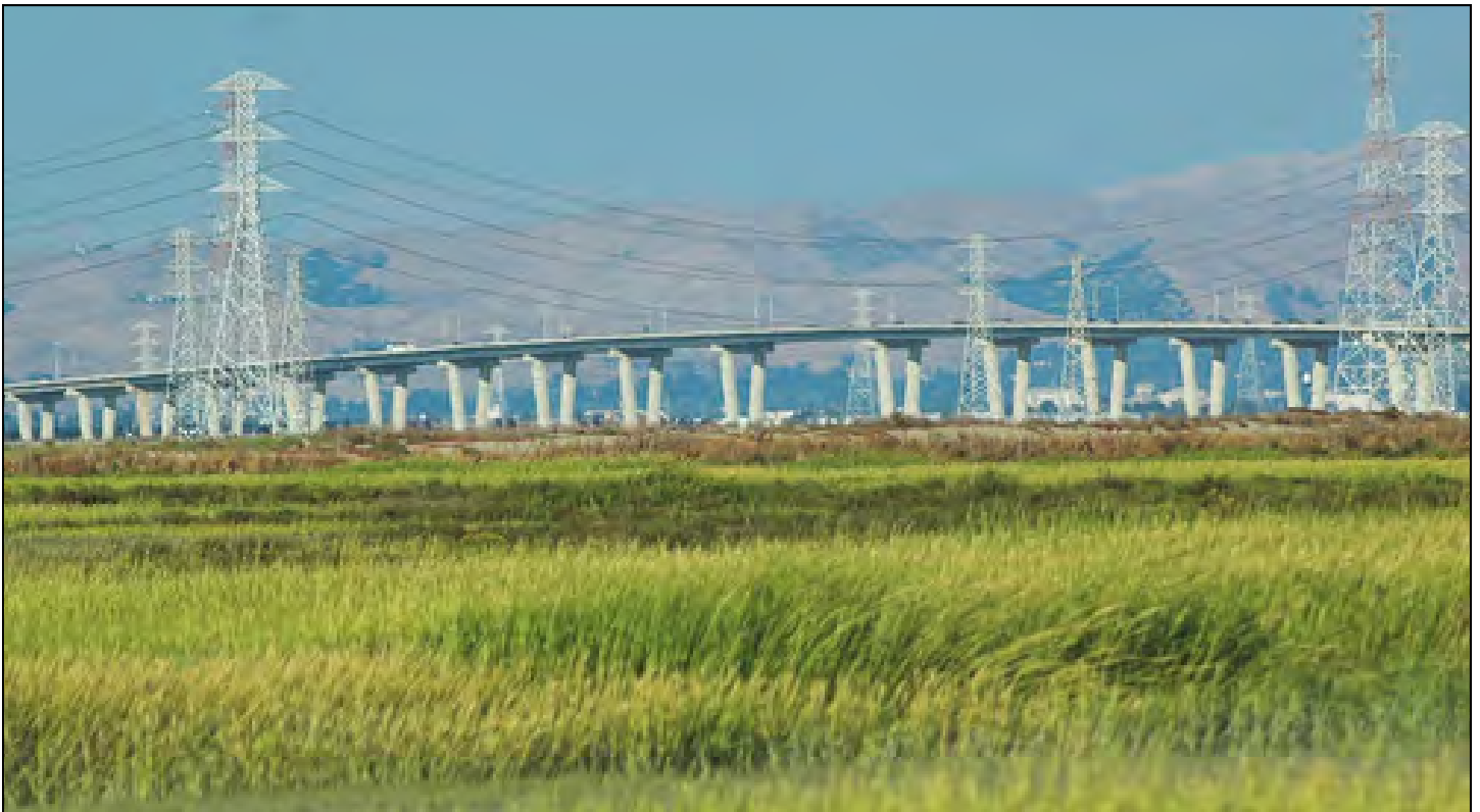
Existing Dumbarton Bridge Looking East towards the Alameda County Foothills
