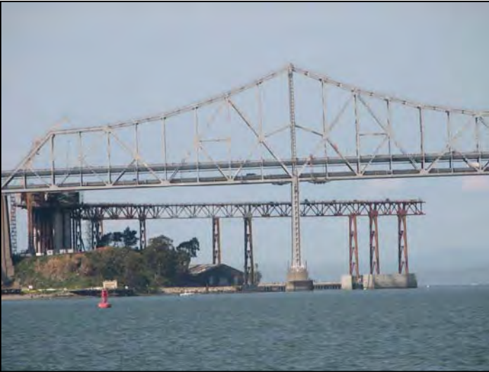
Temporary Support Structures for the SAS Bridge Erection
