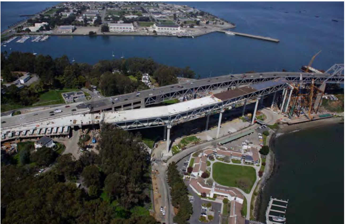
Yerba Buena Island Detour Viaduct under Construction (foreground) with East Tie-In Support Structures Being Erected (right)
