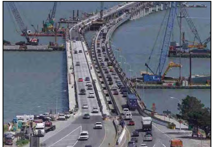
New Richmond-San Rafael Bridge West Approach Trestle under Construction
