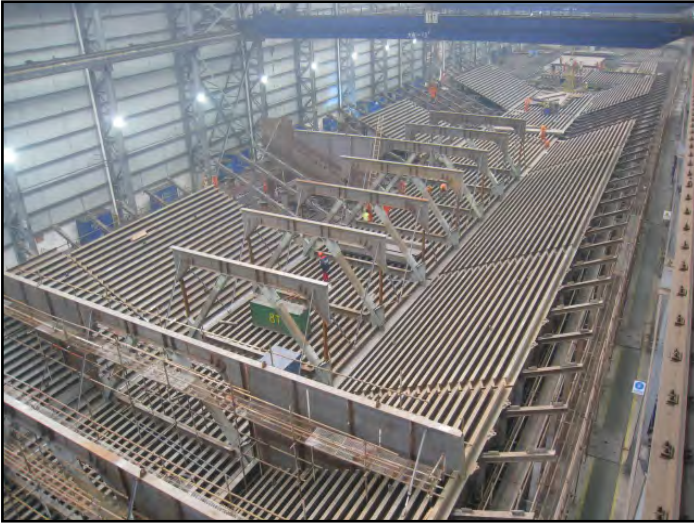
SAS Roadway Boxes in Fabrication
