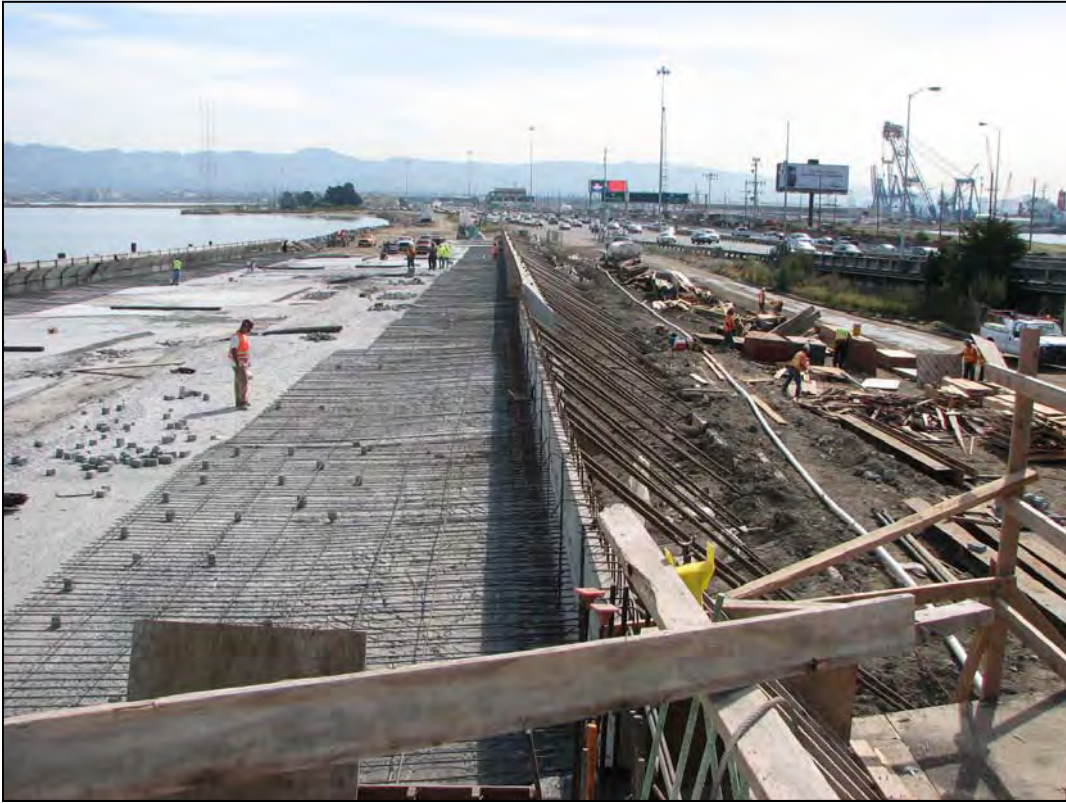
Westbound Precast Panels Installed
