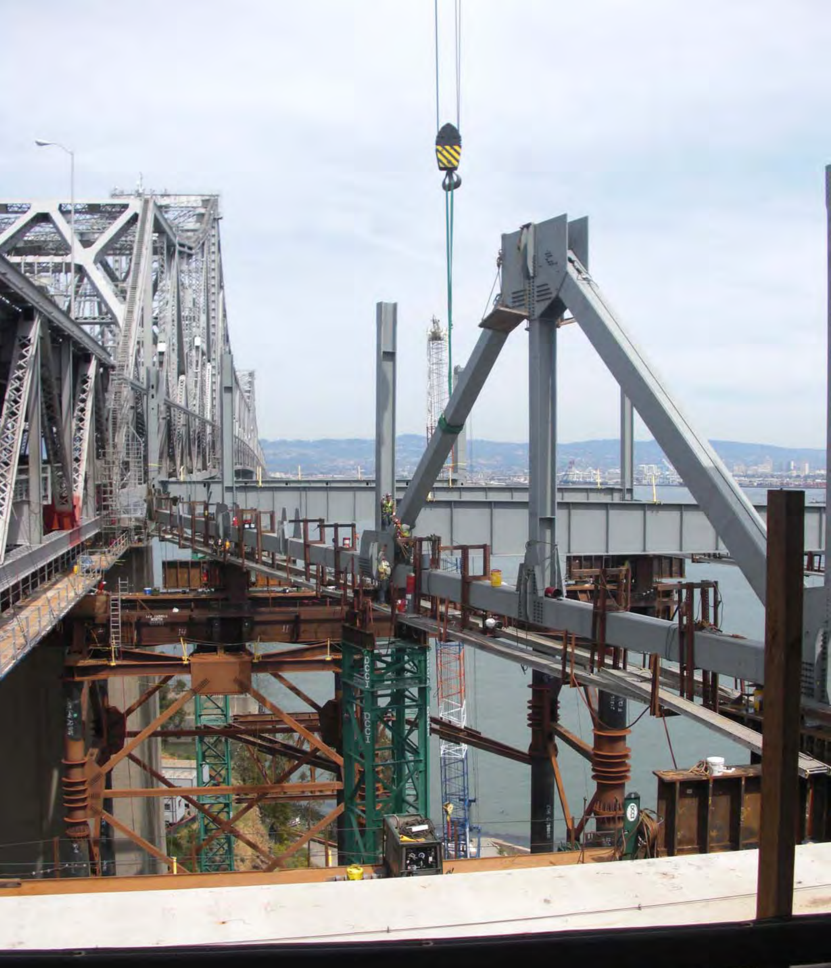
East Tie-In Truss structure under Construction atop Skid Beams
