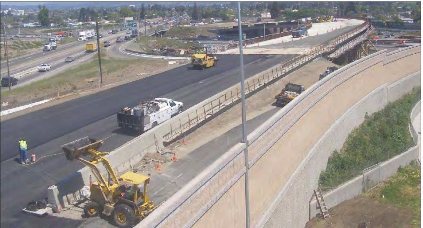
New East Route 92 to North Interstate 880 Connector under Construction.
