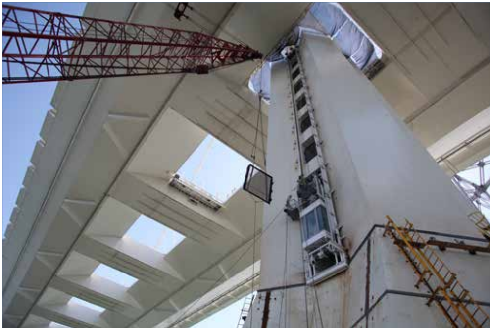
Elevator Installation on the Tower of the Self-Anchored Suspension Bridge
