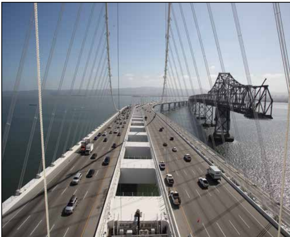
Cantilever Deck Removal in Progress Looking toward Oakland
