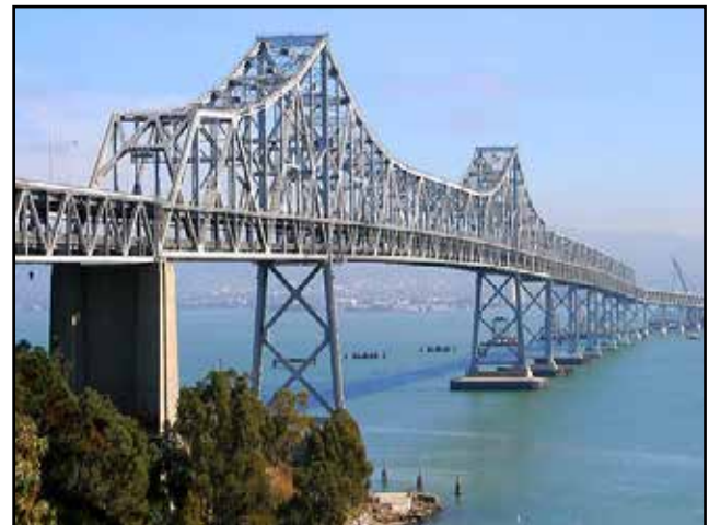
The existing East Span Cantilever Section of the San Francisco-Oakland Bay Bridge to be Dismantled after Seismic Safety Opening of the New Bridge
