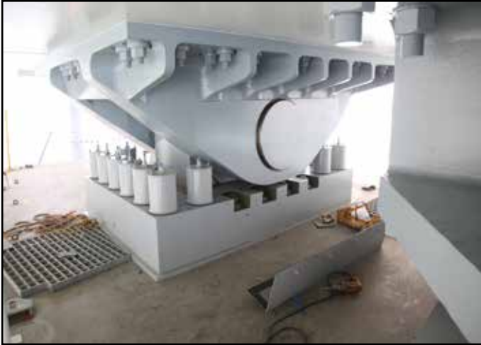
Self-Anchored Suspension Bridge Cover Plate Installation at Bearing B4
