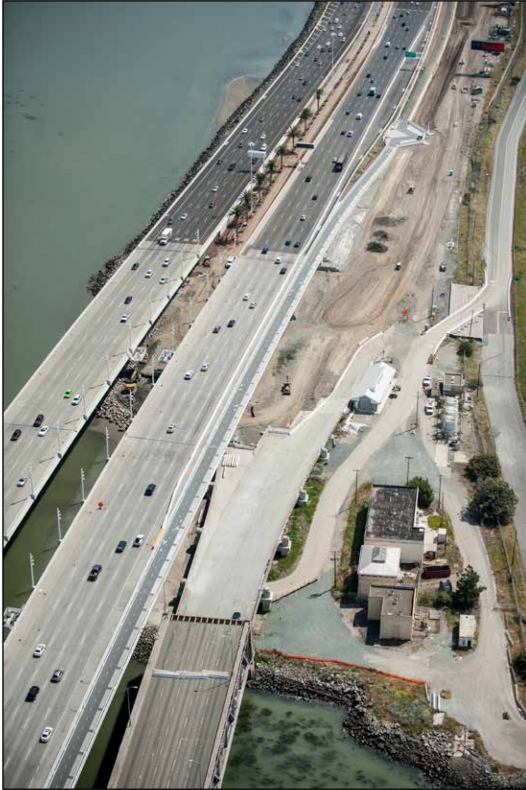
Aerial View of Oakland Touchdown, Construction Progress
