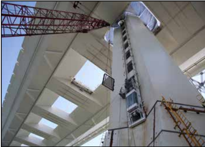
Self-Anchored Suspension Bridge Installing Elevator at Tower
