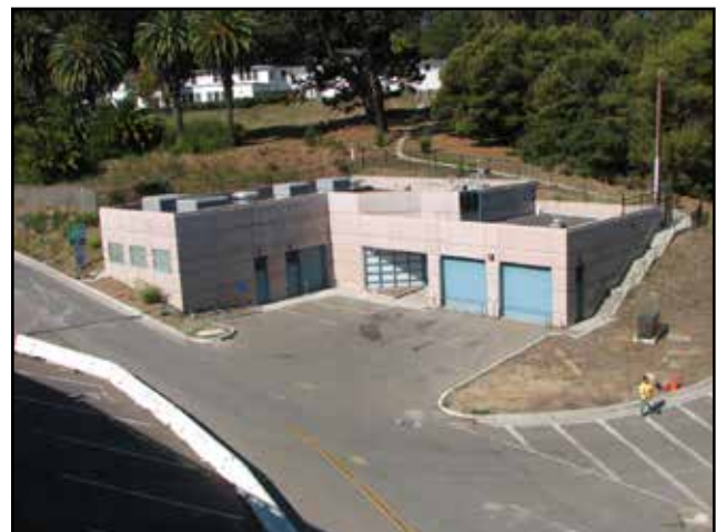
New YBI Electrical Substation
