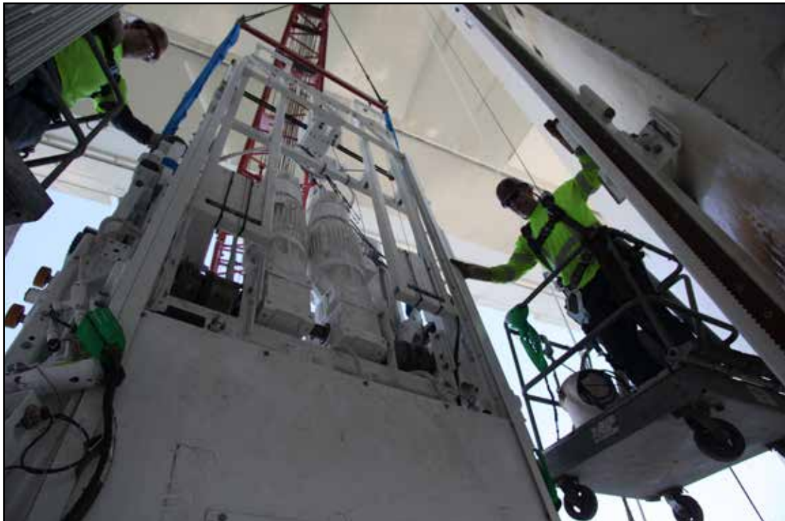
Elevator Cab Erection to Tower
