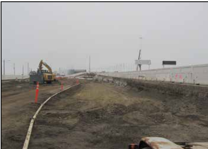
Oakland Touchdown #2 Permanent Bike Path Progress Looking west
