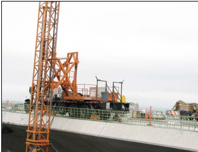
Concrete Finishing of the Soffit
