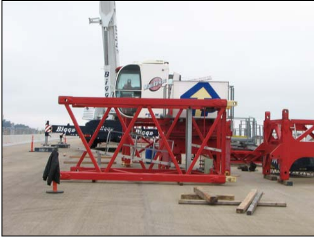
Dismantling tower crane
