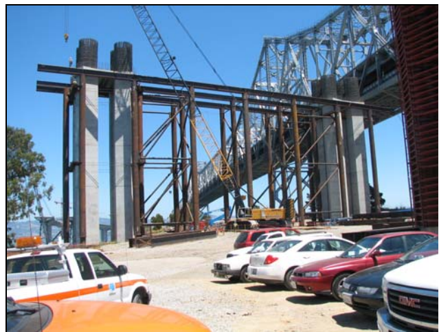
W2 Bent for the Transition Structure
