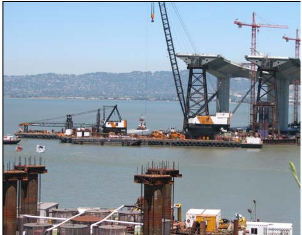
E2&T1 Foundation, with Skyway at the Background
