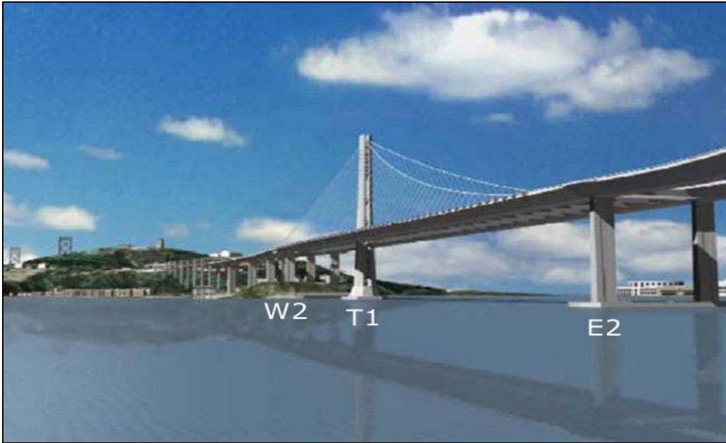
T1 = Foundation for the 530-foot steel tower E2 = Eastern Support of the suspension roadway W2 = Western Support of the suspension roadway
