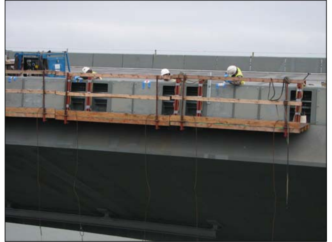
Bridge Rail Erection
