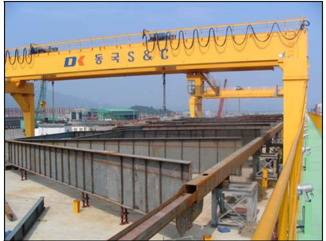
Fabrication of the Viaduct at the Dongkuk Facility
