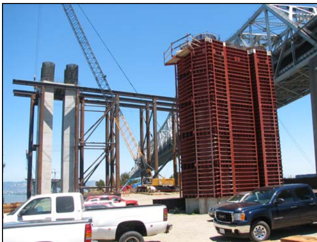
W2 & W3 Bents for the Transition Structure
