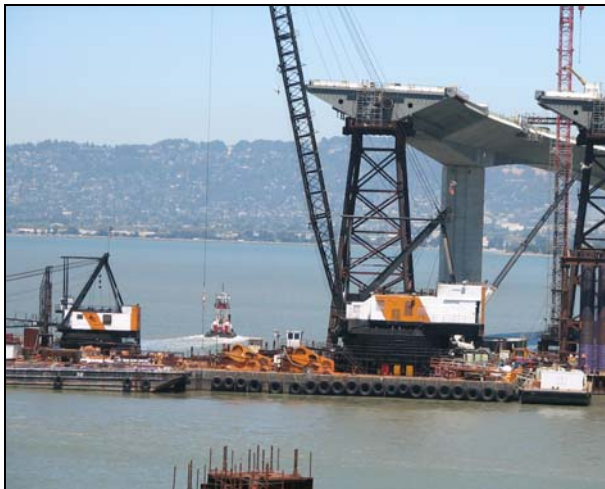
E2 Foundation & Portion of the Skyway Bridge
