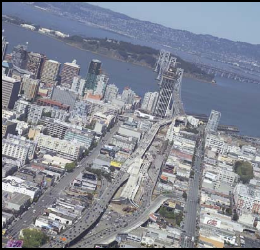
Aerial view of West Approach
