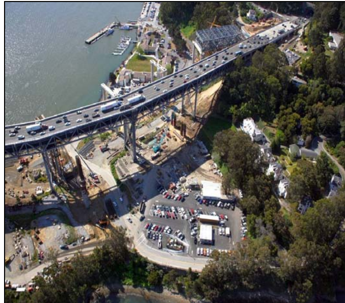
East Span Overview
