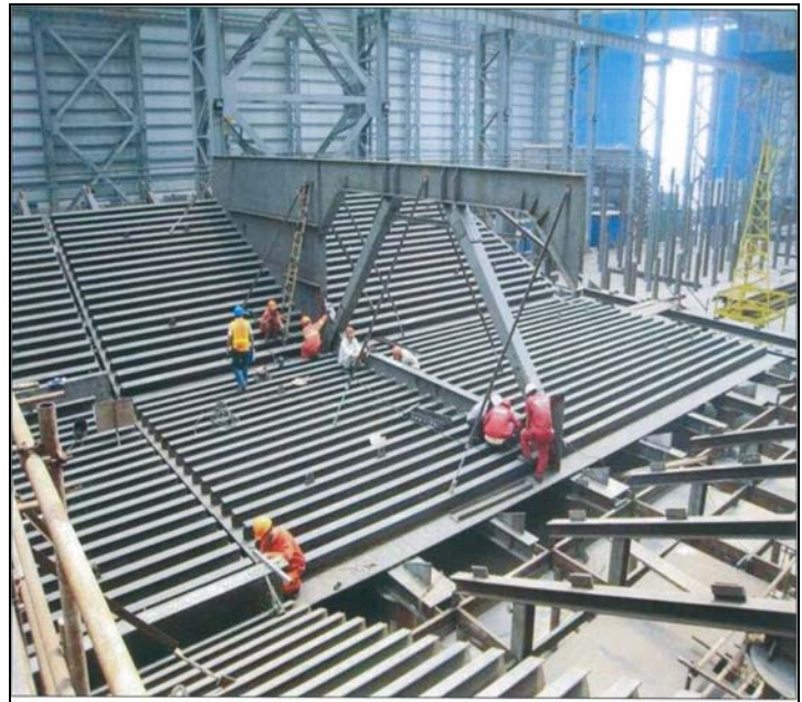
OBG Segment Assembly in the Jig for Bottom and Side Panels
