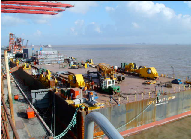
SAS – Barge Crane Installation
