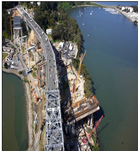
Yerba Buena Island Detour Work
