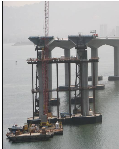
Completed E2/T1 Towers
