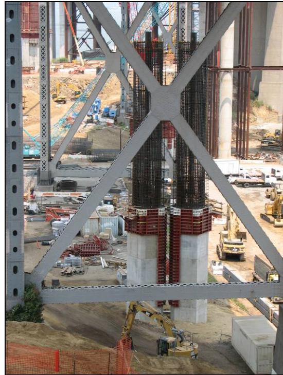
YBITS Advanced Column Work on the YBID Contract
