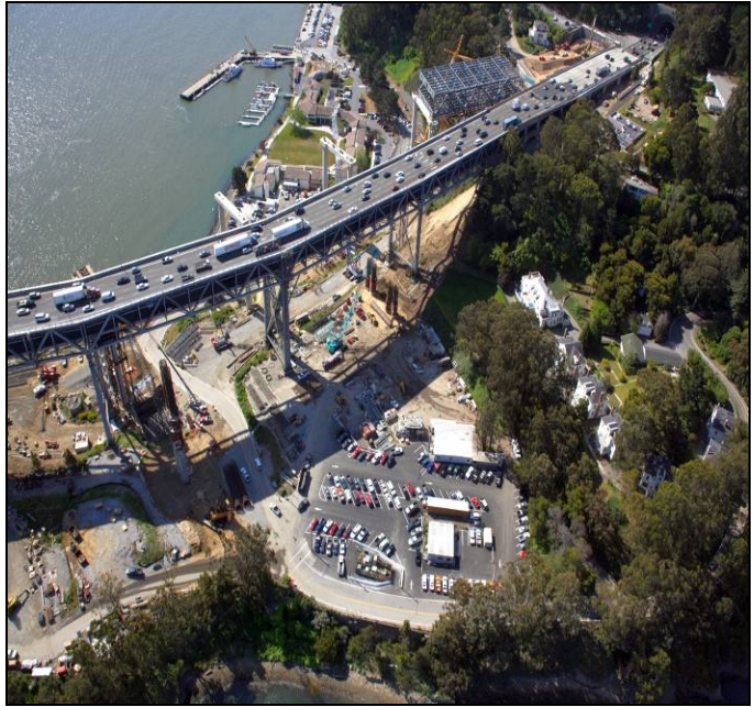
Aerial of YBITS Advanced Work
