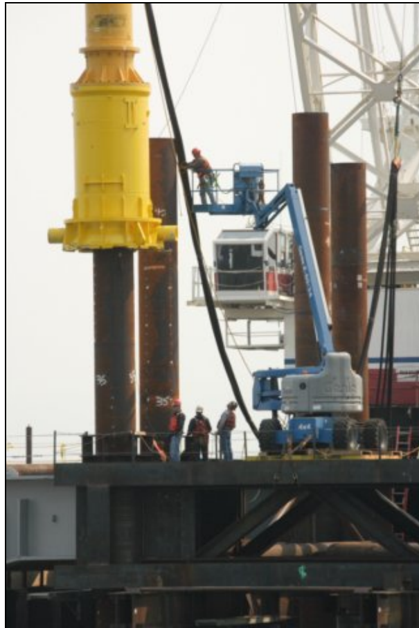
SAS - Temporary Tower D Pile Driving
