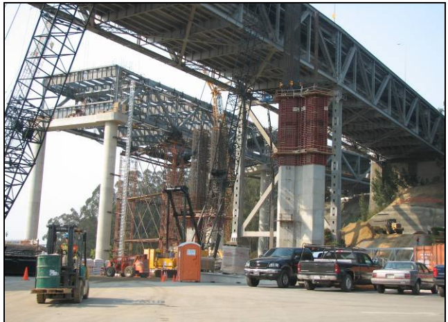
Viaduct Structure and the Advanced YBITS Bent W6 LR
