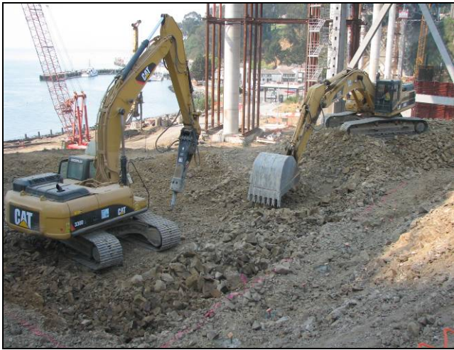
Excavation for Advanced YBITS W3R Footing
