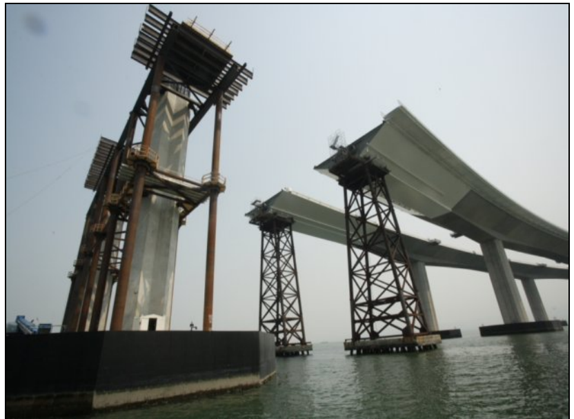
SAS – E2 Temporary Supports
