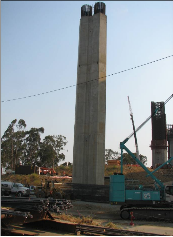
Bent W4L Construction YBI Advanced Work
