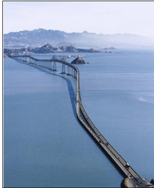
The Richmond-San Rafael Bridge
