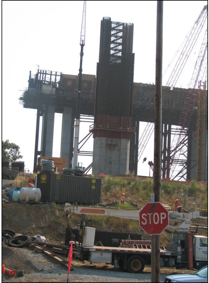
Bent W3L Construction YBI Advanced Work
