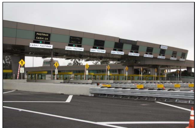
The New Benicia-Martinez Bridge Toll Plaza
