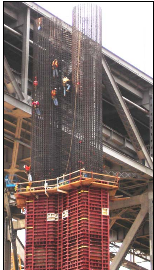
YBITS Advanced Column Work on the YBID Contract
