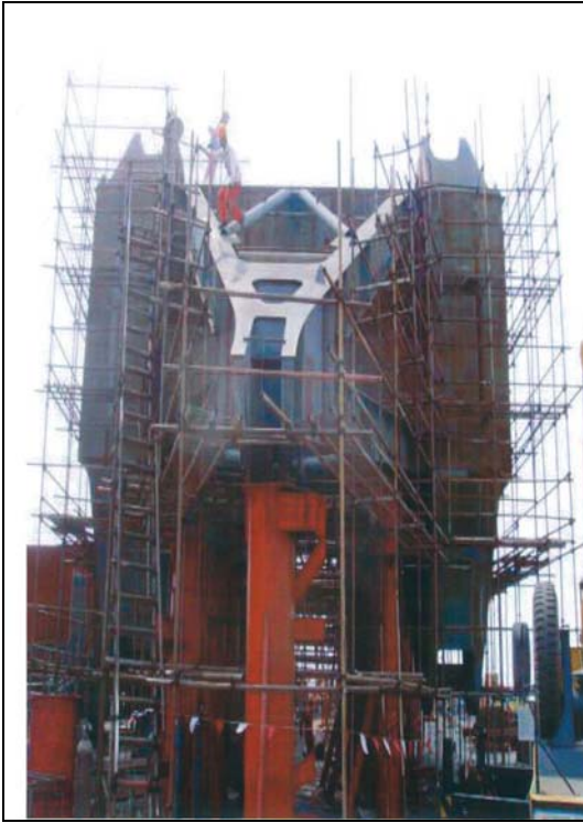
Construction of Crane Head of Shearleg Crane
