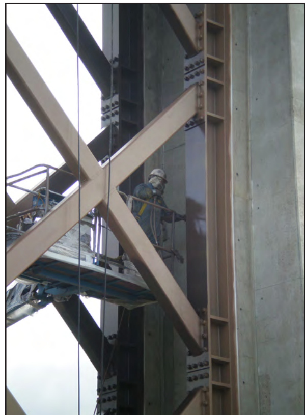
Application of Final Paint Coat at Cross Frames
