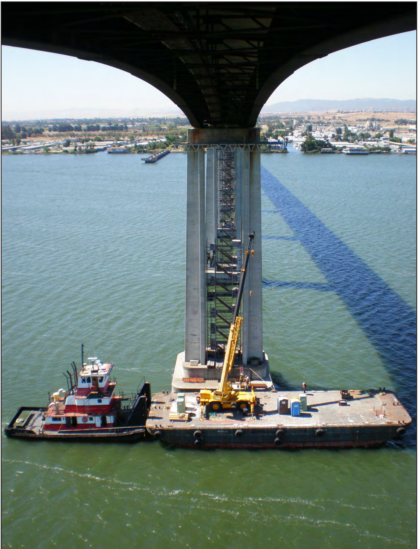
Installation of Access Scaffolding at Pier 14
