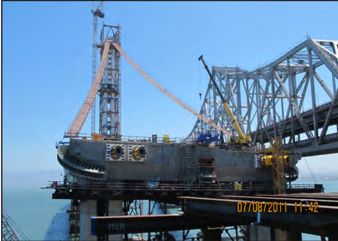
View of the SAS Back Span Catwalk Installed
