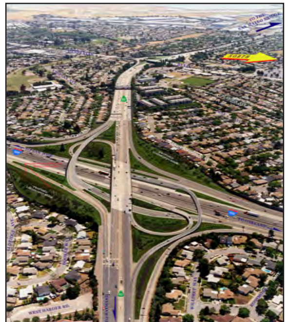
Future Interstate 880/State Route 92 Interchange (as simulated) Looking West toward San Mateo
