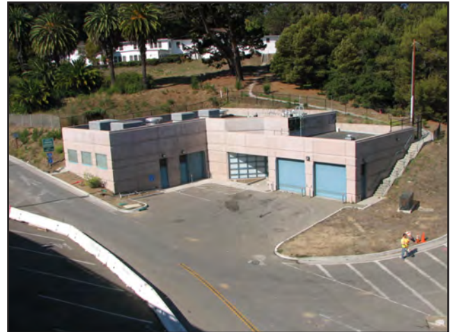
New YBI Electrical Substation
