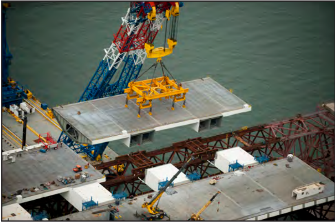
Shear-Leg Crane Barge in Process of Lifting Roadway Box 11 West
