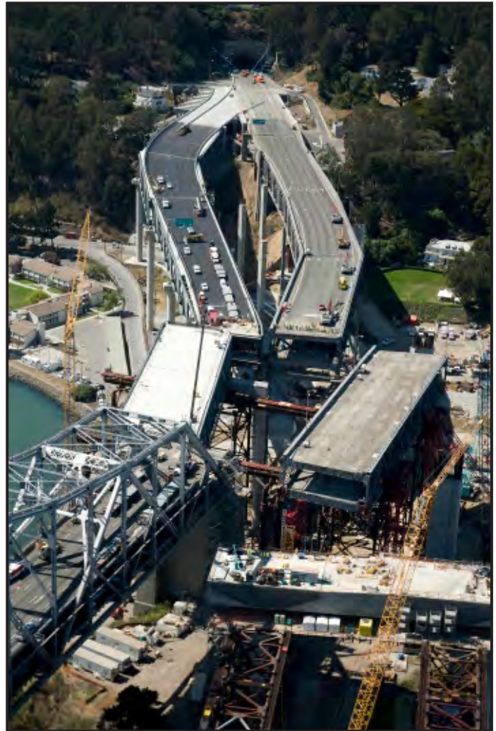
YBI East Tie-In Rolled in on Labor Day 2009 Weekend
