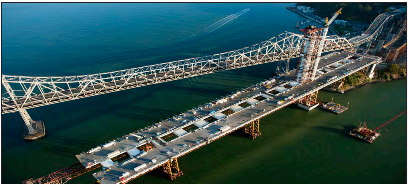
Aerial View of Current Progress on the Self-Anchored Suspension Bridge
