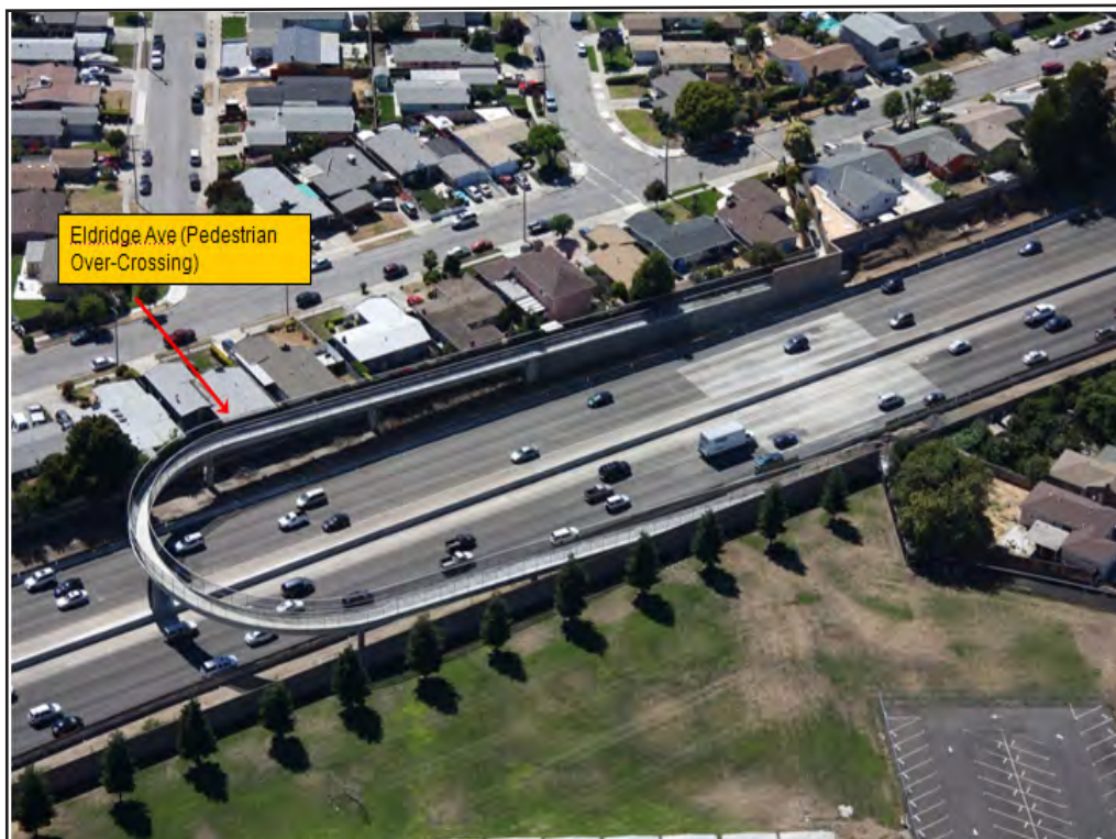
SR-92 Eldridge Avenue Pedestrian Over-Crossing
