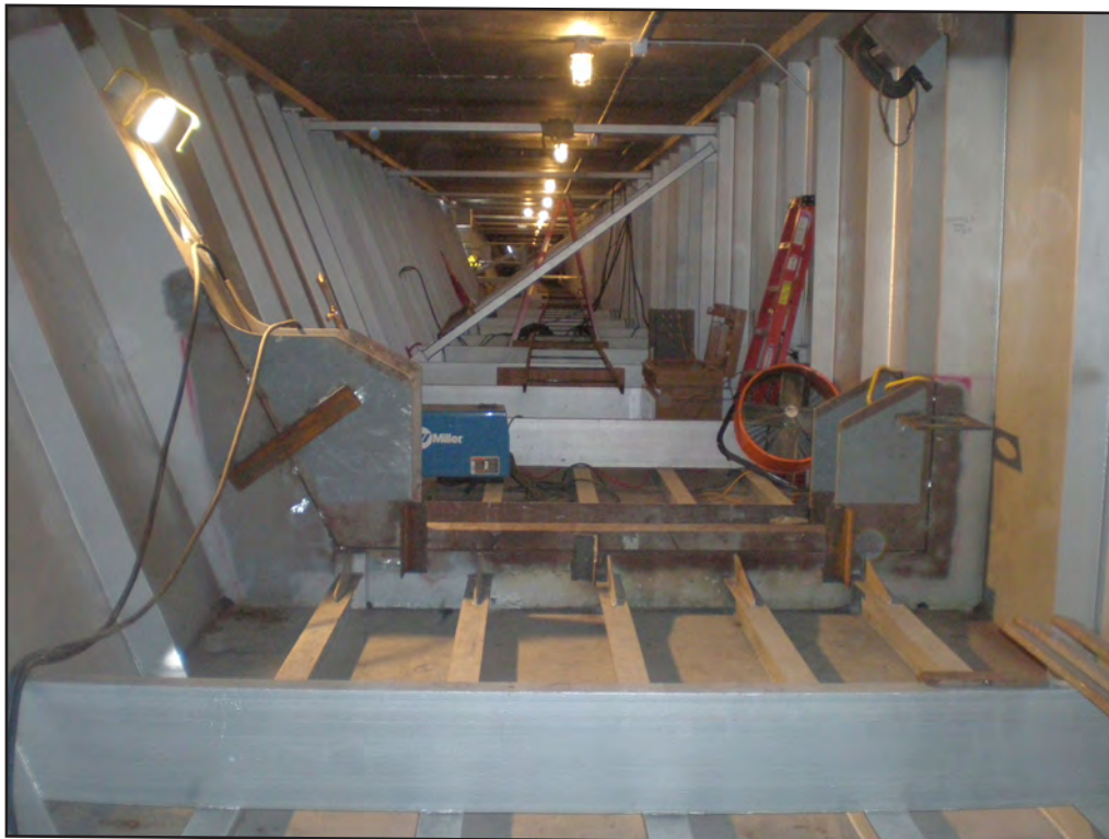
Dumbarton Bridge - Welding of New Cross-Frame Connection Pier 17
