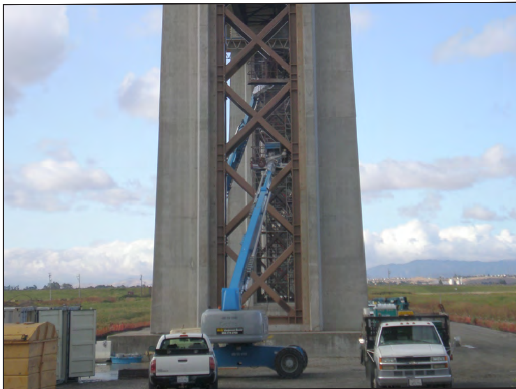
Antioch Bridge - Painting of Cross Frame
