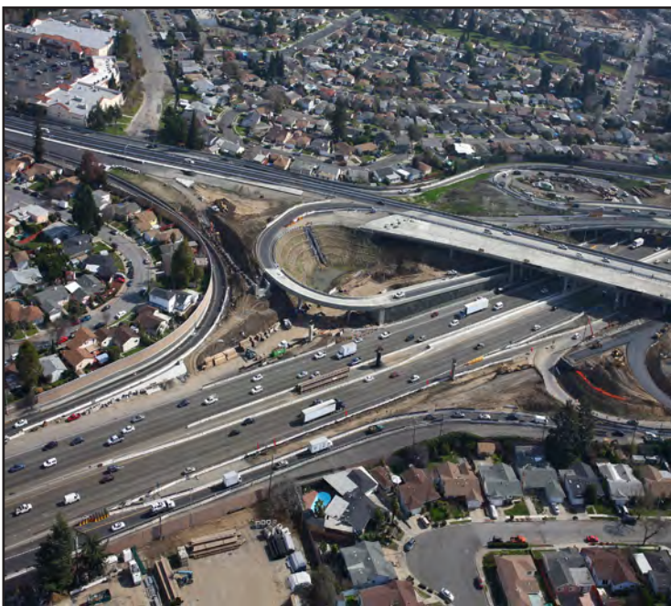
Aerial View of Construction Progress
