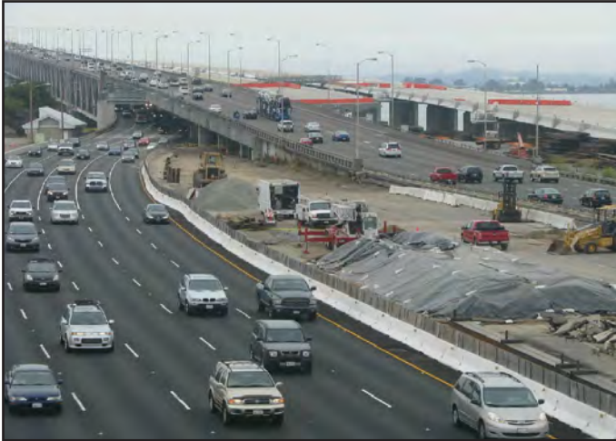
Oakland Detour - Work in Progress
