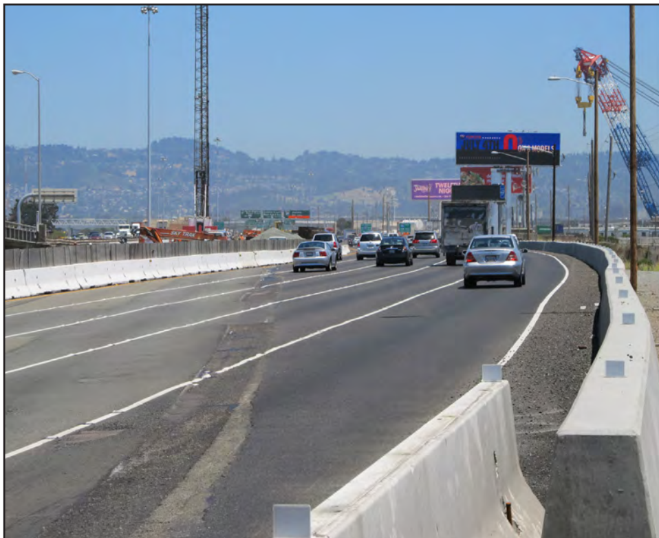
Oakland Detour - Relocated Eastbound Temporary Detour
