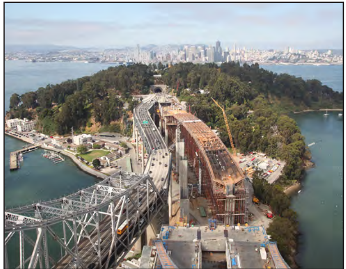
YBITS #1 Westbound Frame 2 Falsework, Formwork and Rebar Installation
