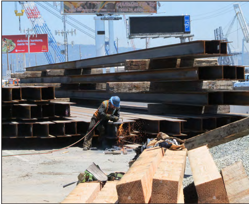
Oakland Detour - Temporary Westbound Piles Being Prepared for Installation
