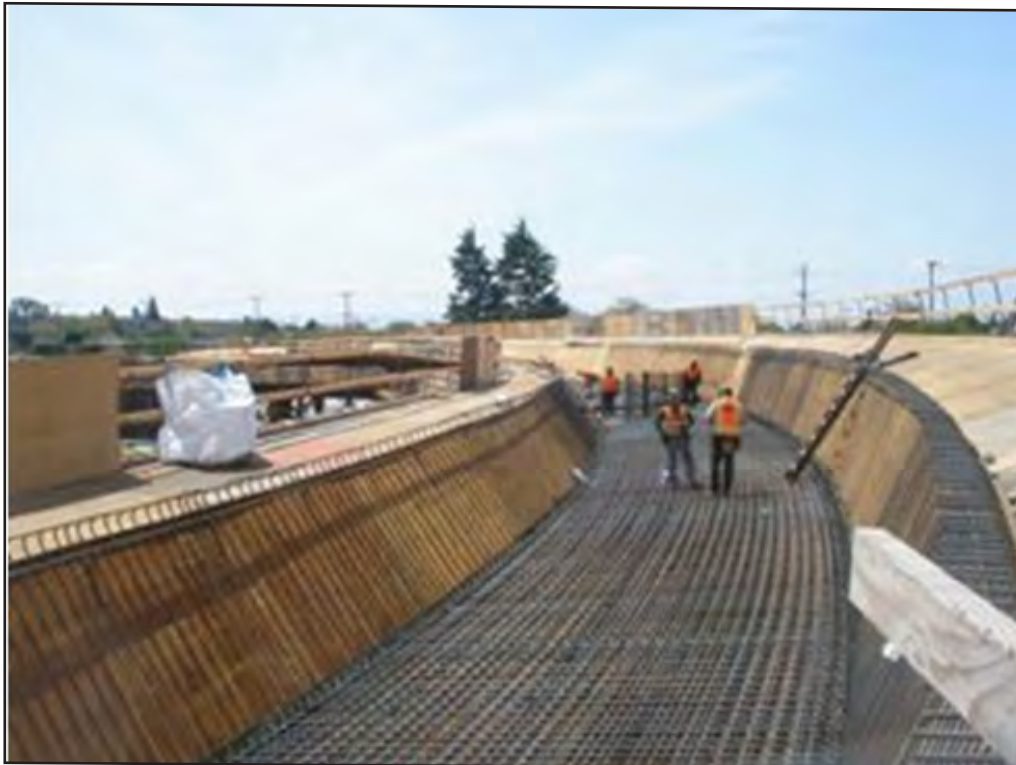
WSCONN Bridge Construction in Progress
