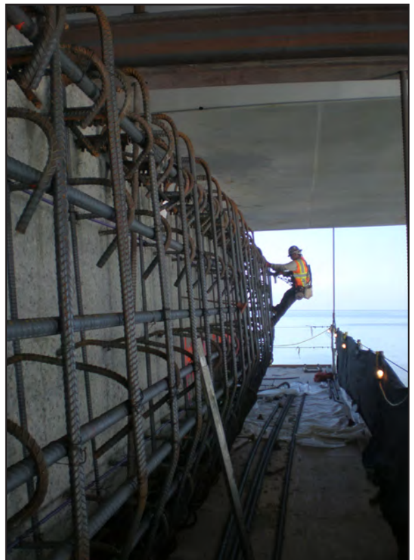
Placement of Reinforcing Steel at Pier 17 Bent
