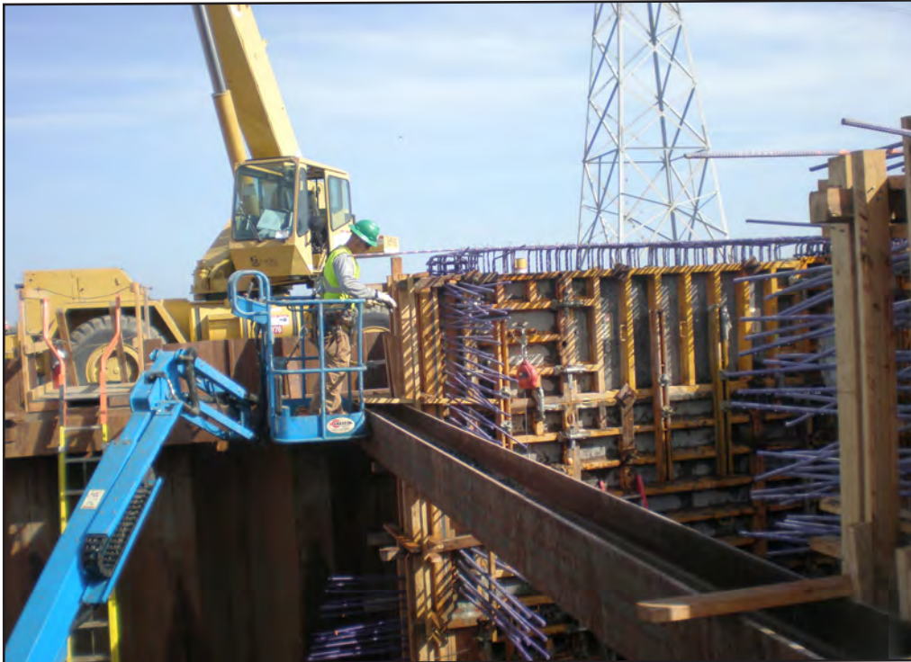
Dumbarton Bridge - Forming Pump Station Walls
