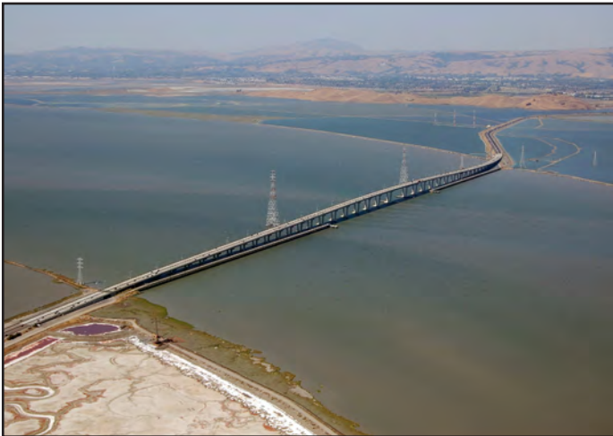
Aerial View of the Dumbarton Bridge
