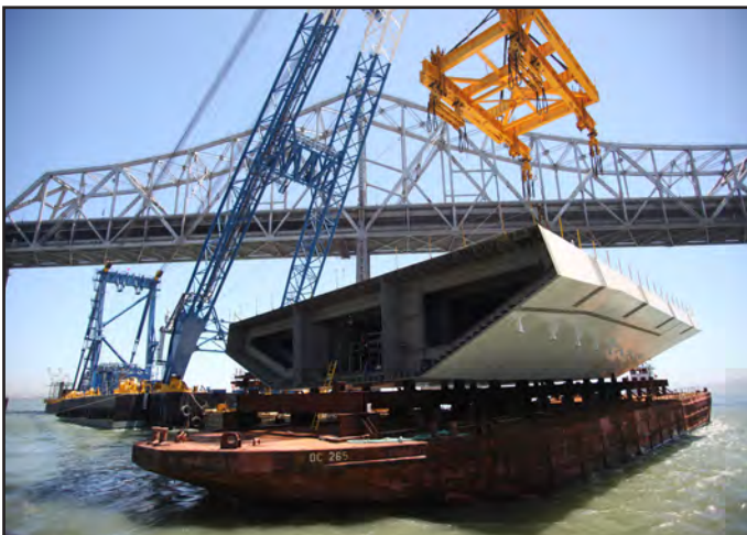
Roadway Box 12 West Being Lifted by the Shear-Leg Crane Barge
