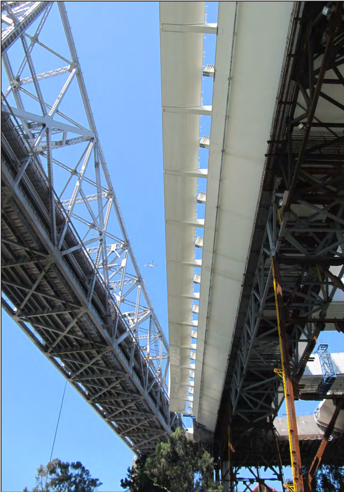
Self-Anchored Suspension Bridge Bike Path Deck Installation in Progress
