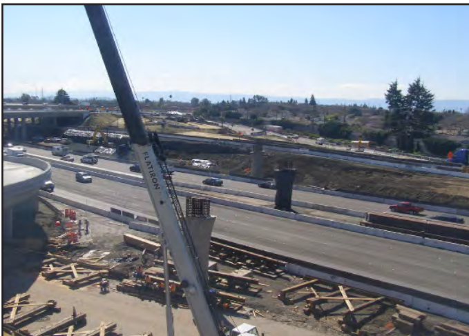
92/880 NWCONN Bridge Construction
