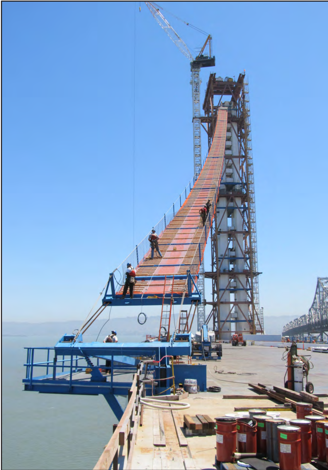
Cable Catwalk Installation for the Westbound Backspan
