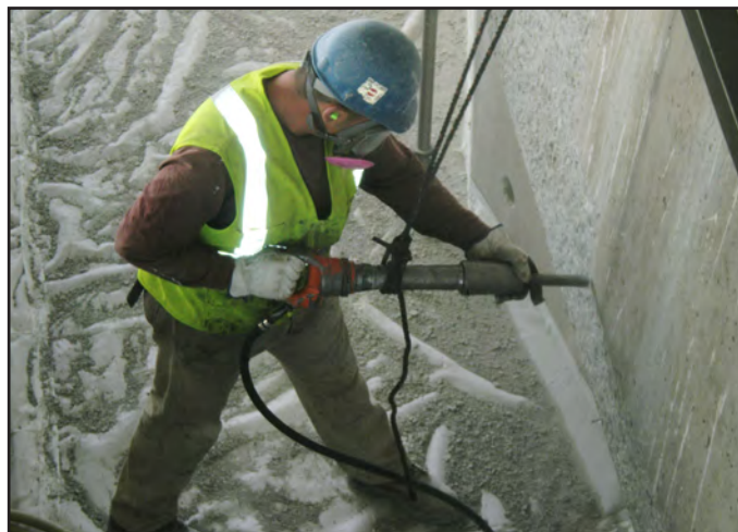
Dumbarton Bridge - Roughening Face of Existing Bent Cap
