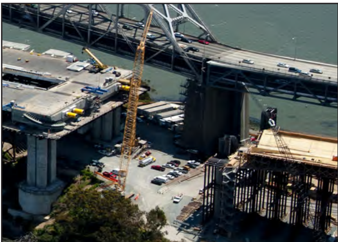
Pier W2 and Hinge K and West Deviation Saddle on left and YBITS #1 on right
