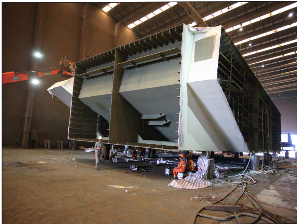
Self-Anchored Suspension Bridge Roadway Box 14 East Bay
