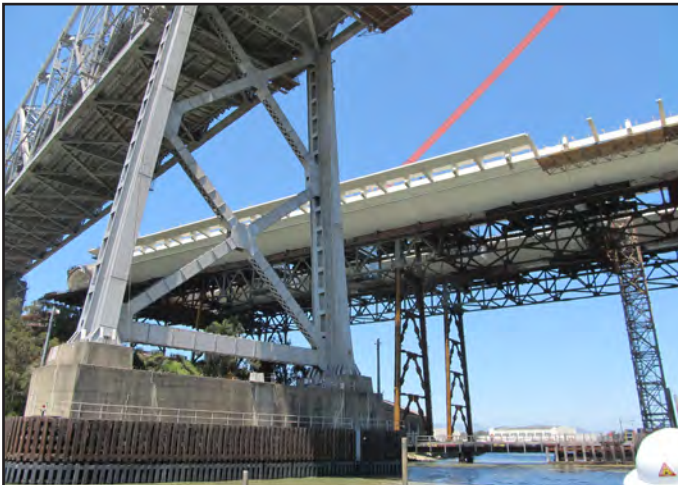
Bike Path Installed on the Eastbound Self-Anchored Suspension Bridge
