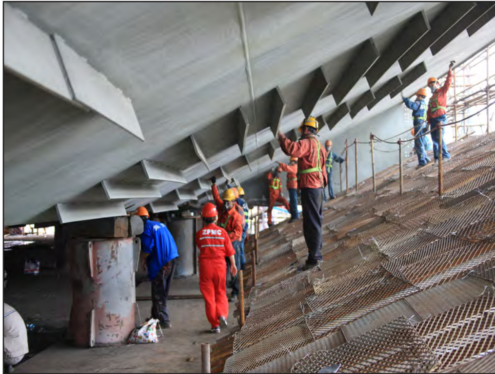
Self-Anchored Suspension Bridge Roadway Box Being Inspected before Shipment
