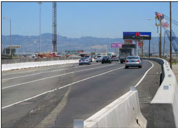
Oakland Detour - Relocated Eastbound Temporary Detour
