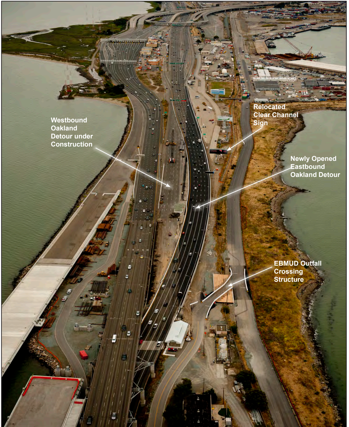
Aerial View of the Newly Opened Eastbound Oakland Detour with the EBMUD Outfall Crossing Structure on the right, the Relocated Clear Channel Sign and the Westbound Oakland Detour under Construction
