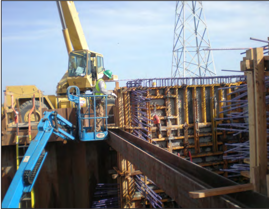
Forms in Place for Pump Station Walls
