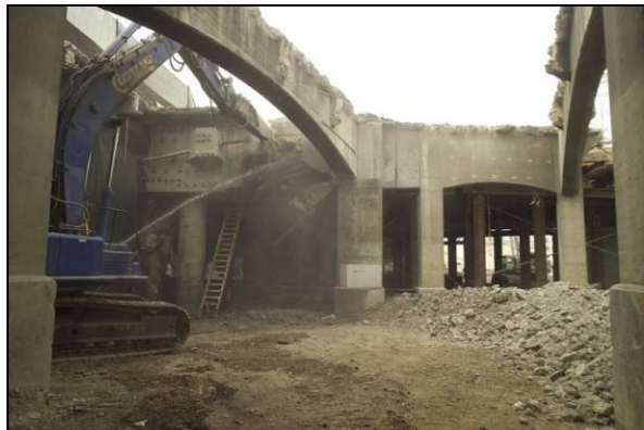
West Approach Tendon Cutting 3.
