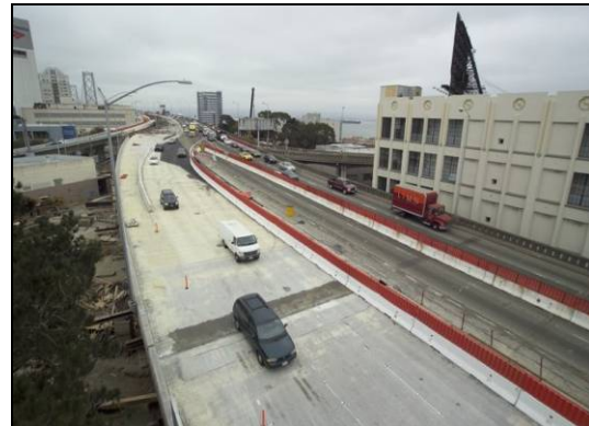
West Approach: New I-80 Westbound Crossover.
