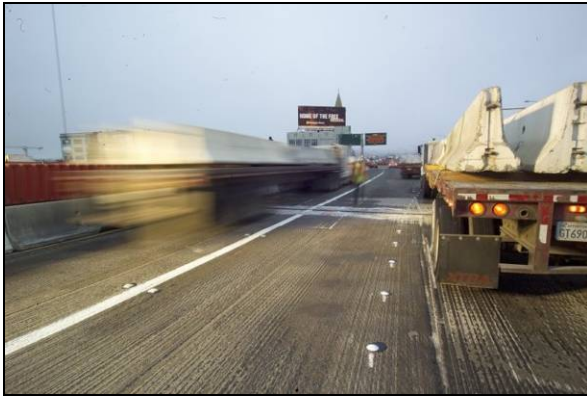
West Approach Tendon Cutting 6.
