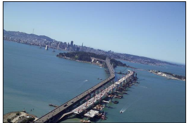
View of Skyway construction Looking West.
