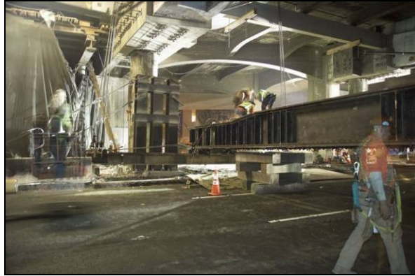
West Approach Support Beam Installation 8.
