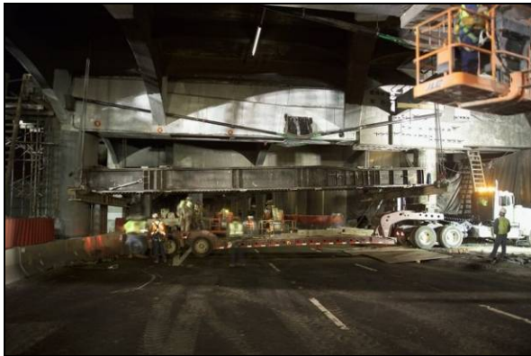
West Approach Support Beam Installation 9.
