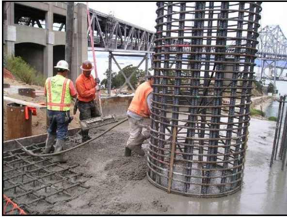
Pouring Concrete for New Pier Footing.
