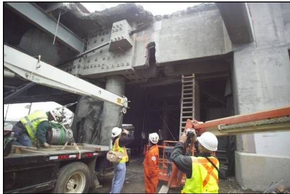
West Approach Tendon Cutting 1.
