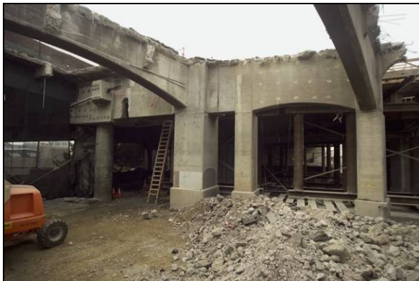
West Approach Tendon Cutting 2.
