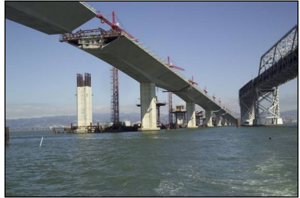
View of Skyway Construction from water level 1.
