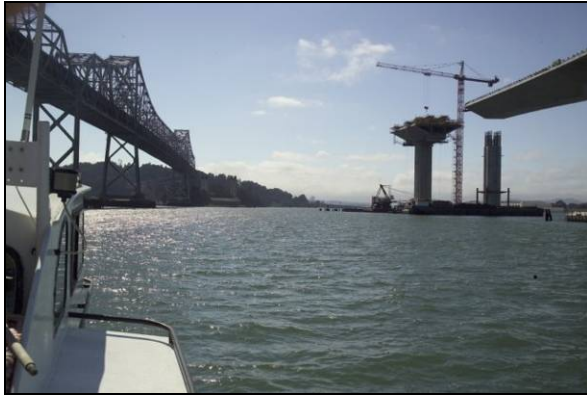
View of new Eastbound Roadway Looking West.
