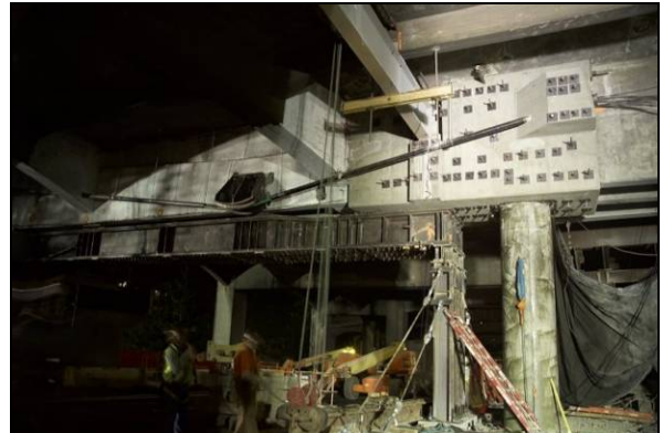
West Approach Support Beam Installation 2.
