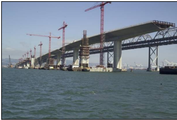
View of Skyway Construction from water level 2.
