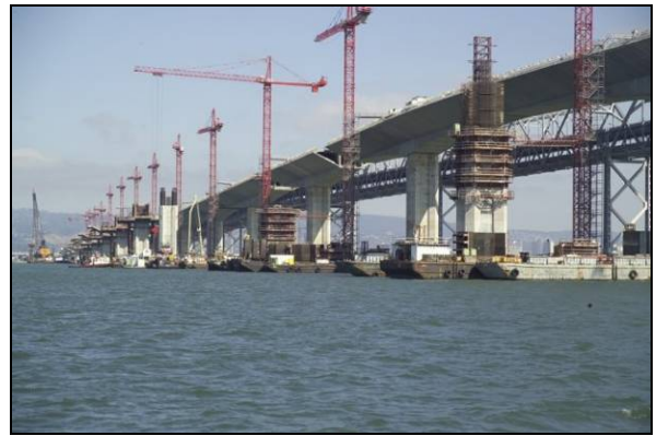
View of Skyway Construction from water level 3.
