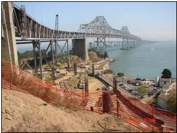
Pier Column Construction for the South-South Detour 1.
