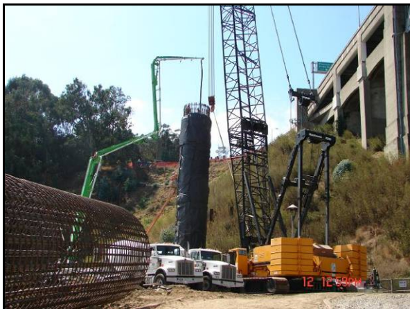
Pier Column Construction for the South-South Detour 3.
