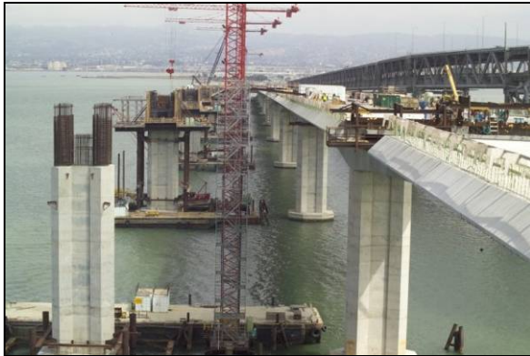
Construction of Eastbound-Westbound Bridge Segments (Looking East).
