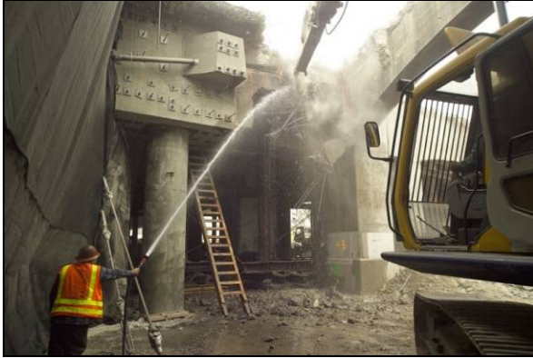
West Approach Tendon Cutting 4.
