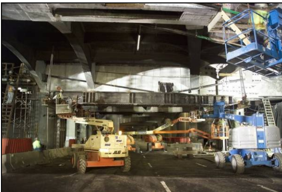
West Approach Support Beam Installation 5.
