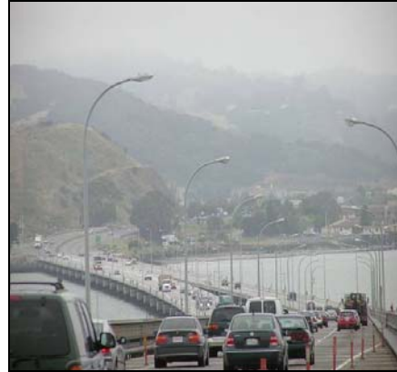
Richmond-San Rafael Bridge Westbound
