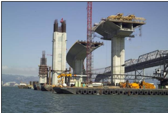
View of Skyway Piers from water level.
