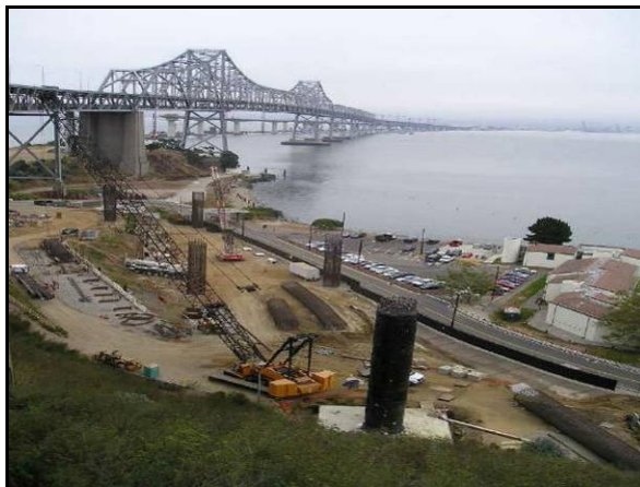
Pier Column Construction for the South-South Detour 4.
