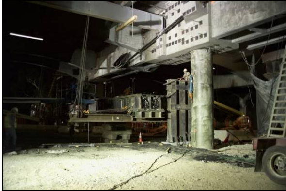
West Approach Support Beam Installation 7.
