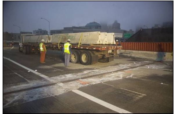
West Approach Tendon Cutting 7.
