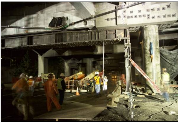
West Approach Support Beam Installation 3.
