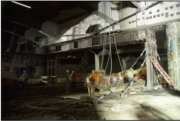
West Approach Support Beam Installation 1.
