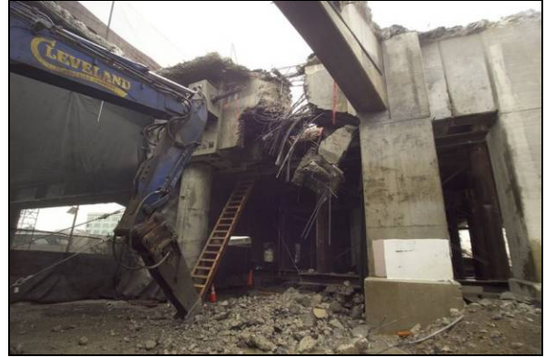
West Approach Tendon Cutting 5.
