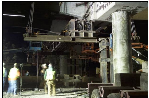
West Approach Support Beam Installation 6.
