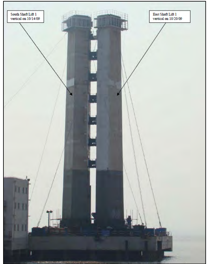
SAS Tower Lift 1 South and East Lift in Vertical Position
