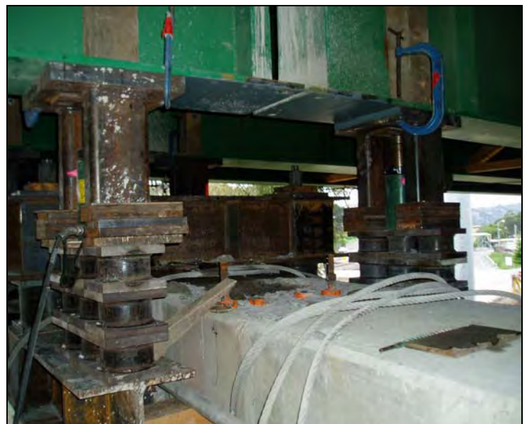
Mococo Road Bridge Jacking
