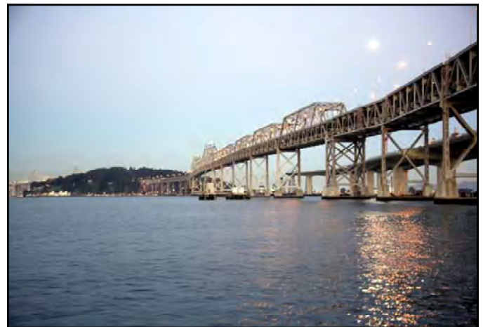
Existing East Span of Bay Bridge
