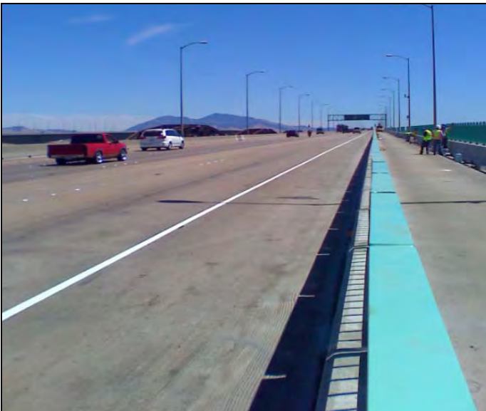
New Pedestrian Bicycle Path on Benicia-Martinez Bridge Under Construction
