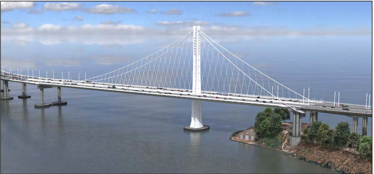
Architectural Rendering of the New Self-Anchored Suspension Bridge on the East Span of the Bay Bridge
