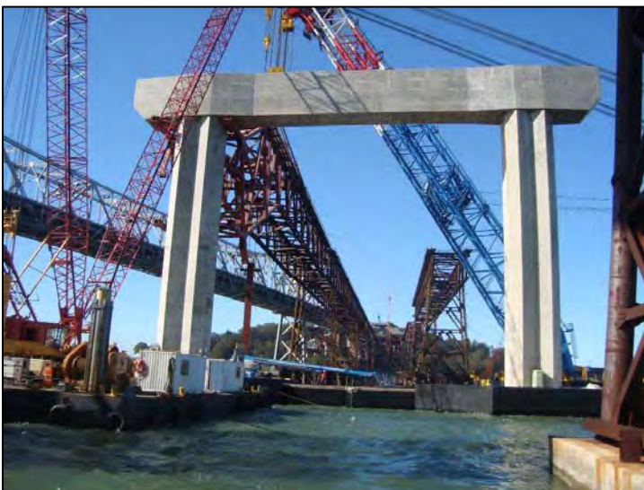
SAS View from East of E2
