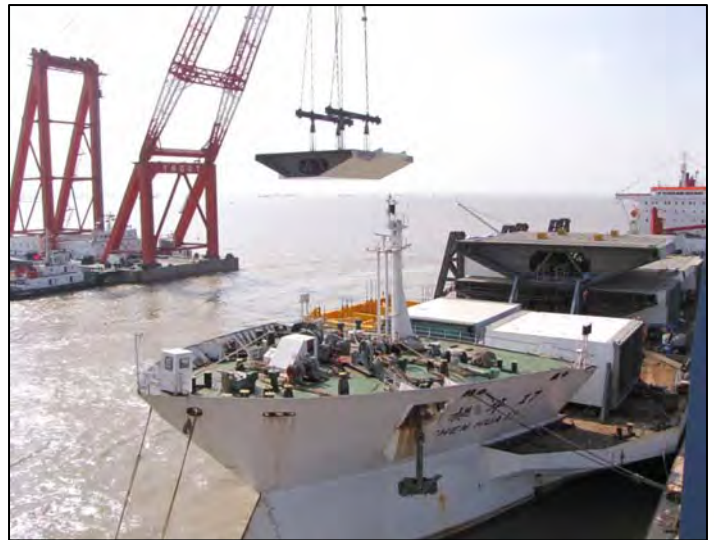
SAS Loading of Segment 3W onto Ship
