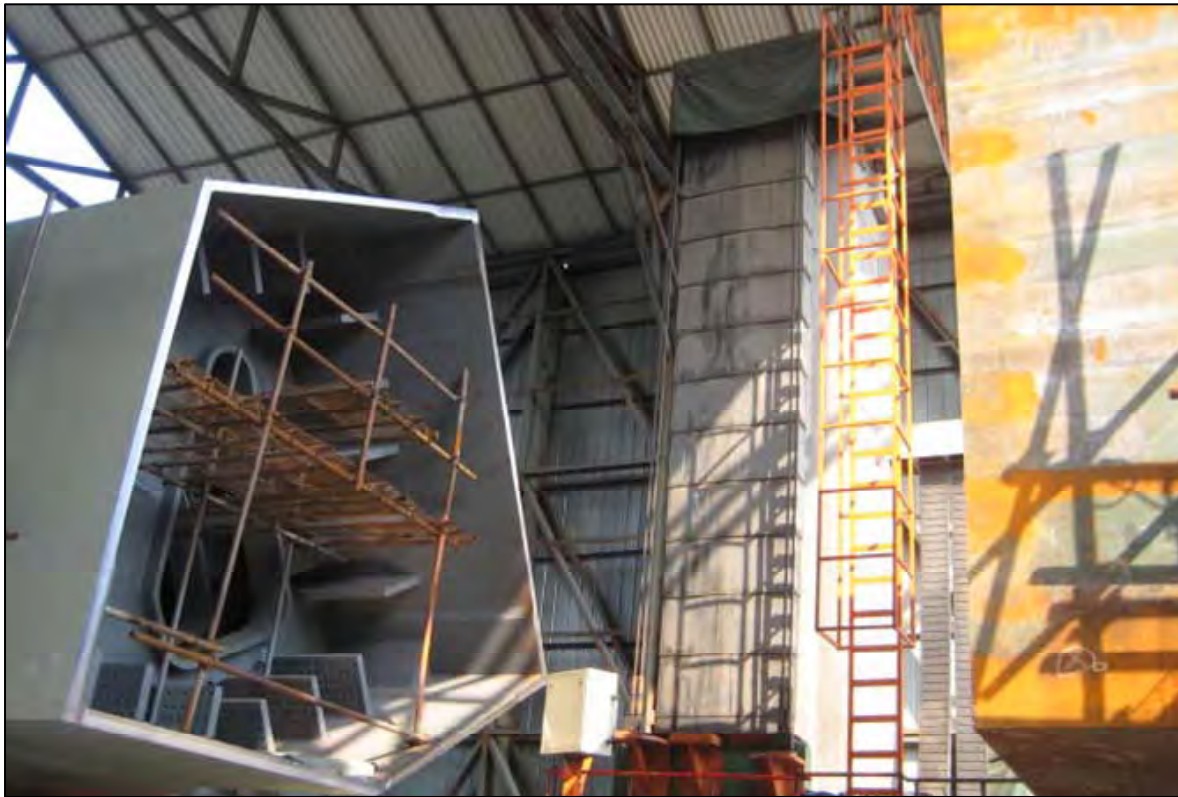
SAS Tower Shaft Lift 1 North-Perimeter Milling in Milling Yard
