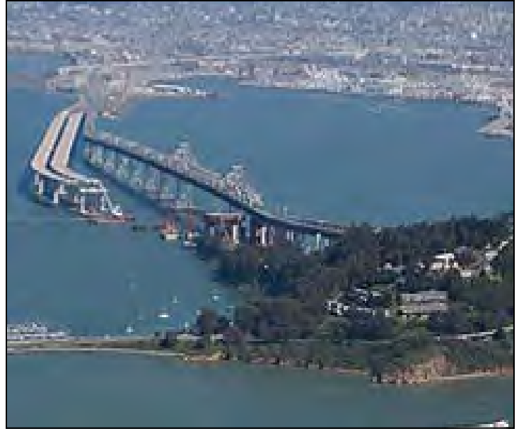
Completed Skyway Left of Existing East Span
