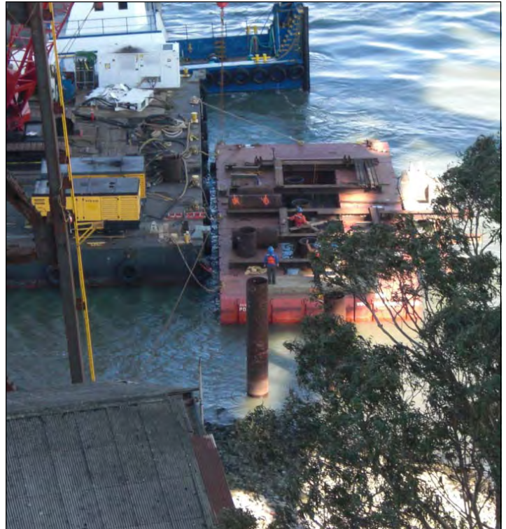
SAS Tower Temporary Trestle Piling Installation in Progress
