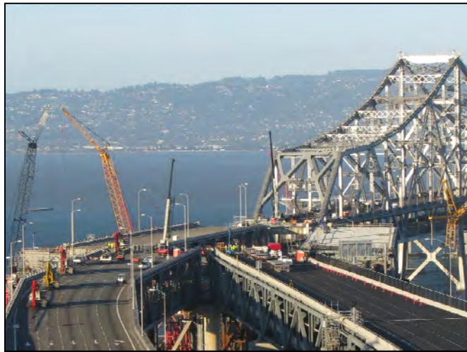
Stage 2 - Roll-Out of Existing Truss
