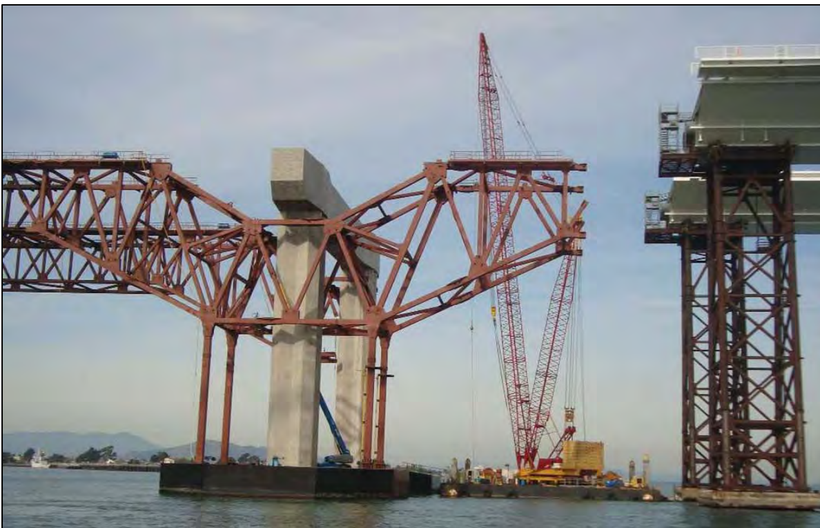
SAS - Temporary Support Structures "E" Line H (E2) toward Skyway
