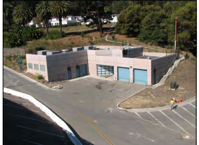
New YBI Electrical Substation
