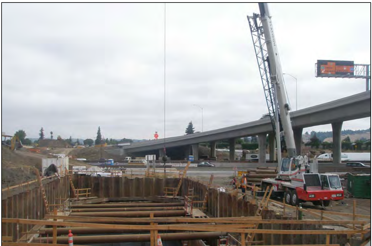
92/880 Pump Station Construction in Progress
