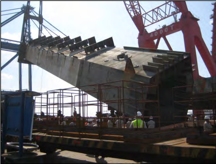
SAS Tower Lifting up Lift 1 South Shaft Tower to Vertical Position
