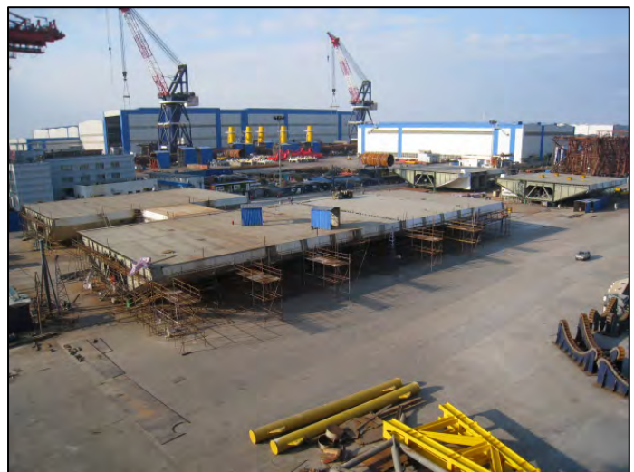
SAS Segment Assembly in Trial Assembly Yard
