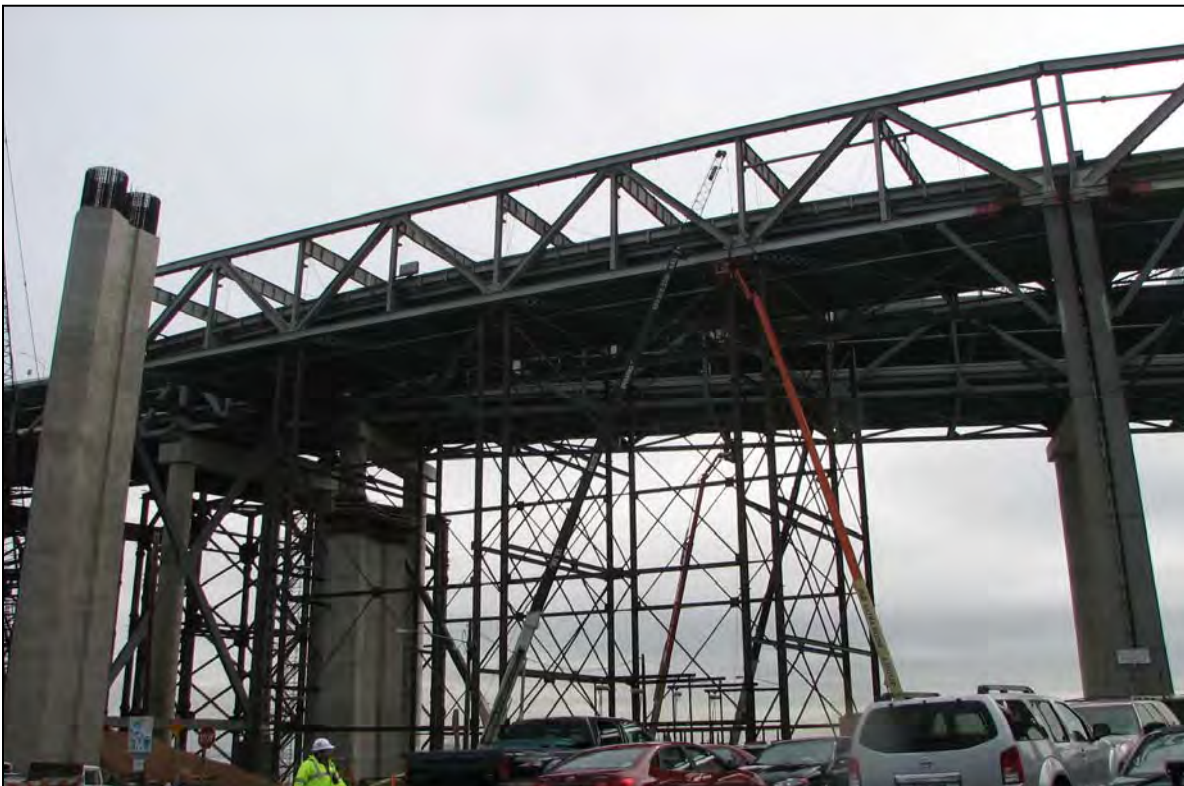
Existing Viaduct Bridge Spans YB3 and YB2 Demolition in Progress
