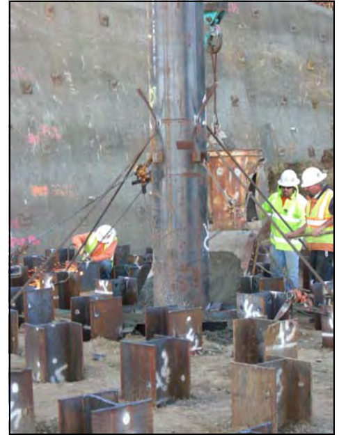
Yerba Buena Island Transition Column W7L North Foundation Piles Installation
