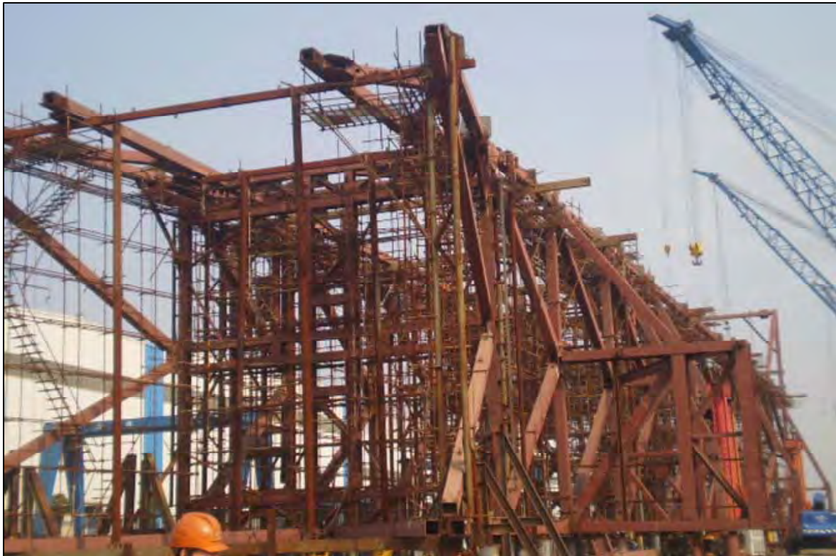
SAS Trial Assembling of T-1 Erection Tower in the Open Yard
