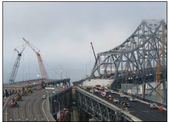
Stage 5 - Prepare Bridge Joints, Barriers, and Striping
