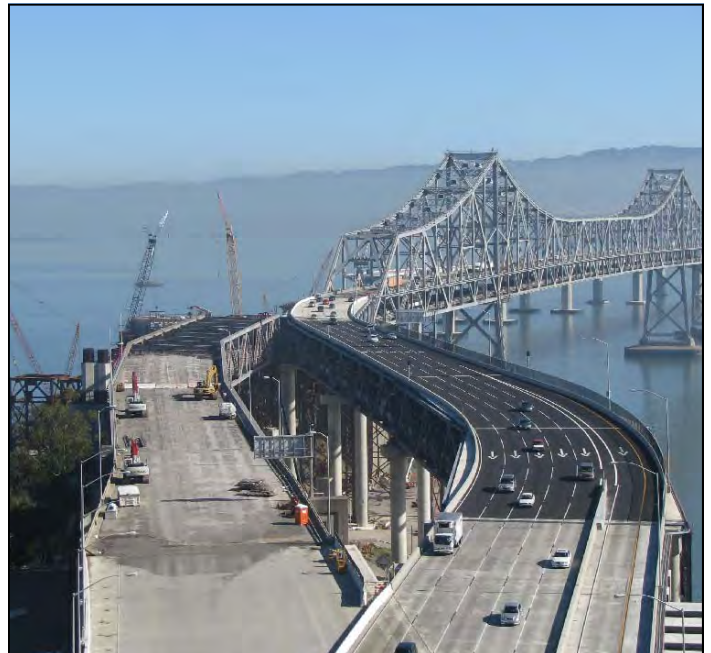
Detour Structure East Tie-In Span Completed over the Labor Day Weekend
