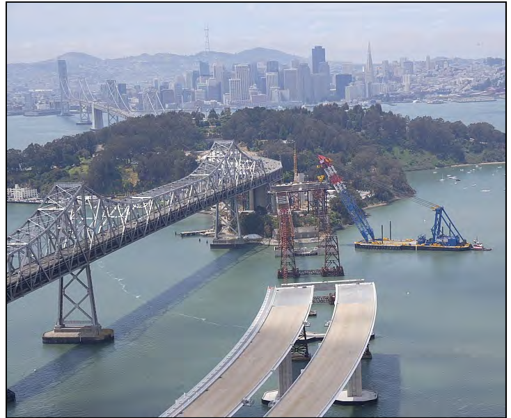
Western End of Completed Skyway
