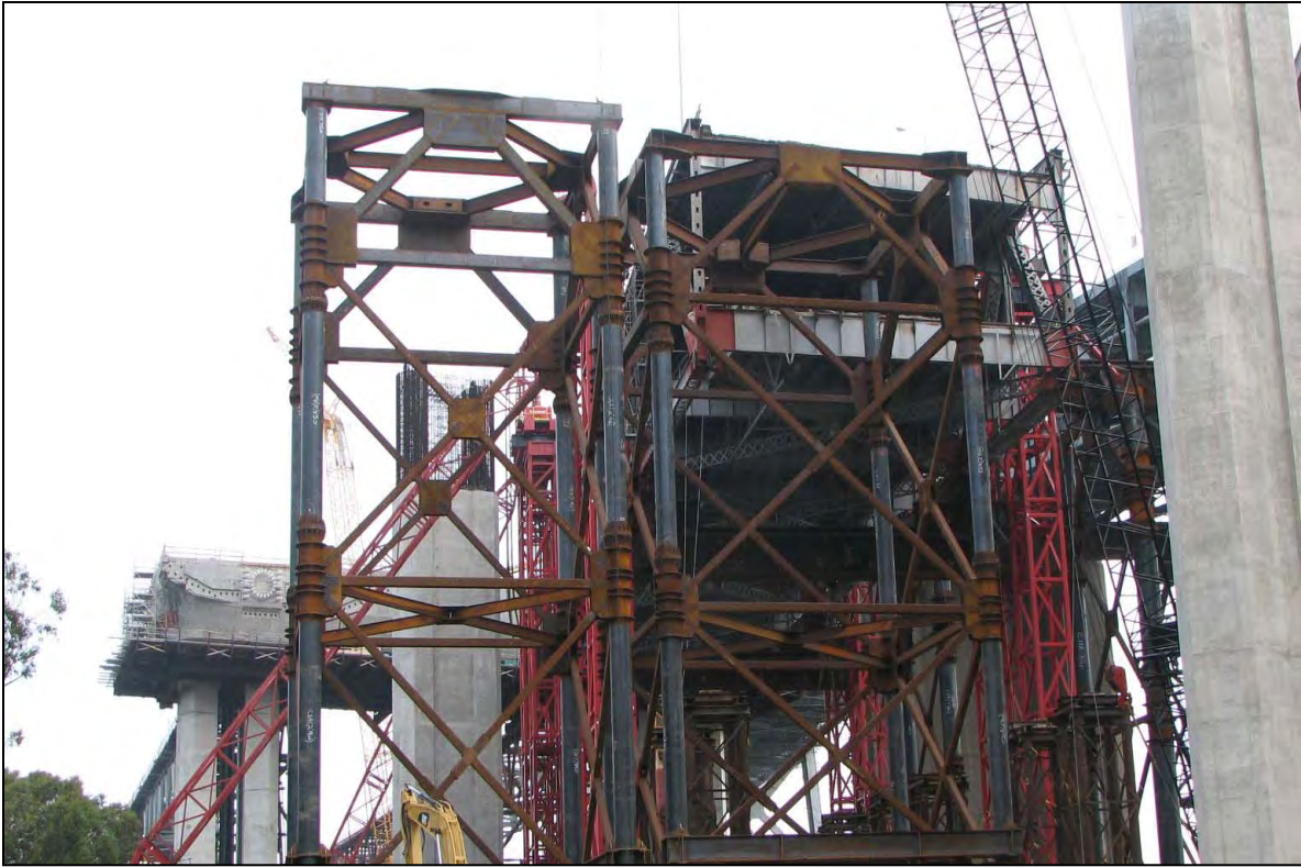
YBID Skid Bent A1 and B1 Moved Out and being Disassembled
