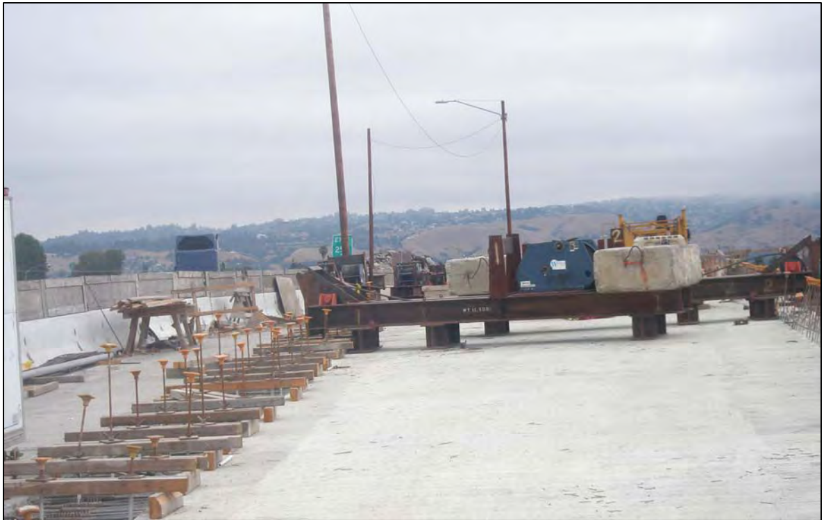
92/880 Widening at Mount Eden Overhead Crossing
