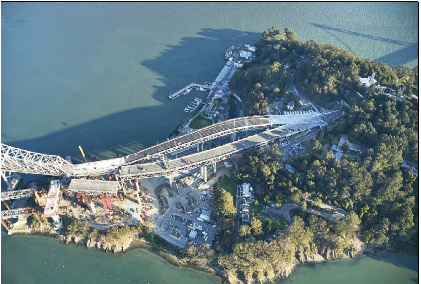
Completed Yerba Buena Island Detour East Tie-In Roll-Out/Roll-In Structure
