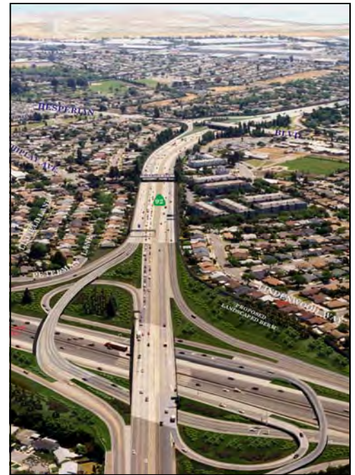
Future Interstate 880/State Route 92 Interchange (as simulated), Looking West toward San Mateo.
