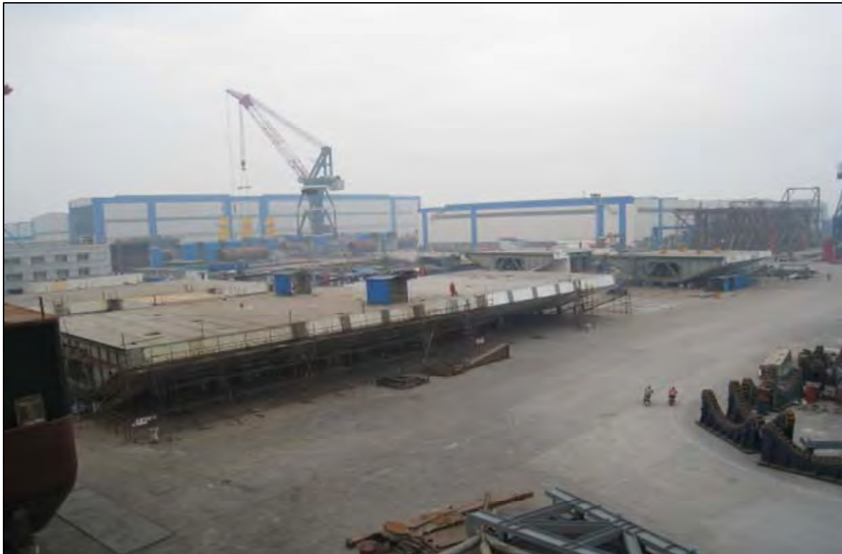
SAS Segment Assembly in the Assembly Yard
