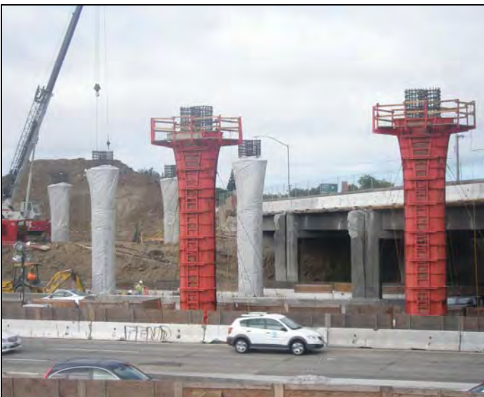
Bents 2, 3 and 4 of the I-880/SR92 Interchange New Separation Bridge
