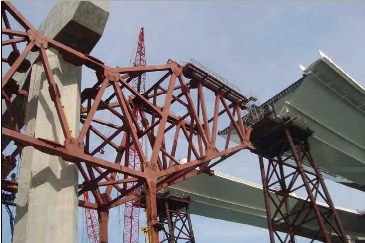
SAS - Temporary Support Structures- "E" Line H (E2) toward Skyway Close-Up
