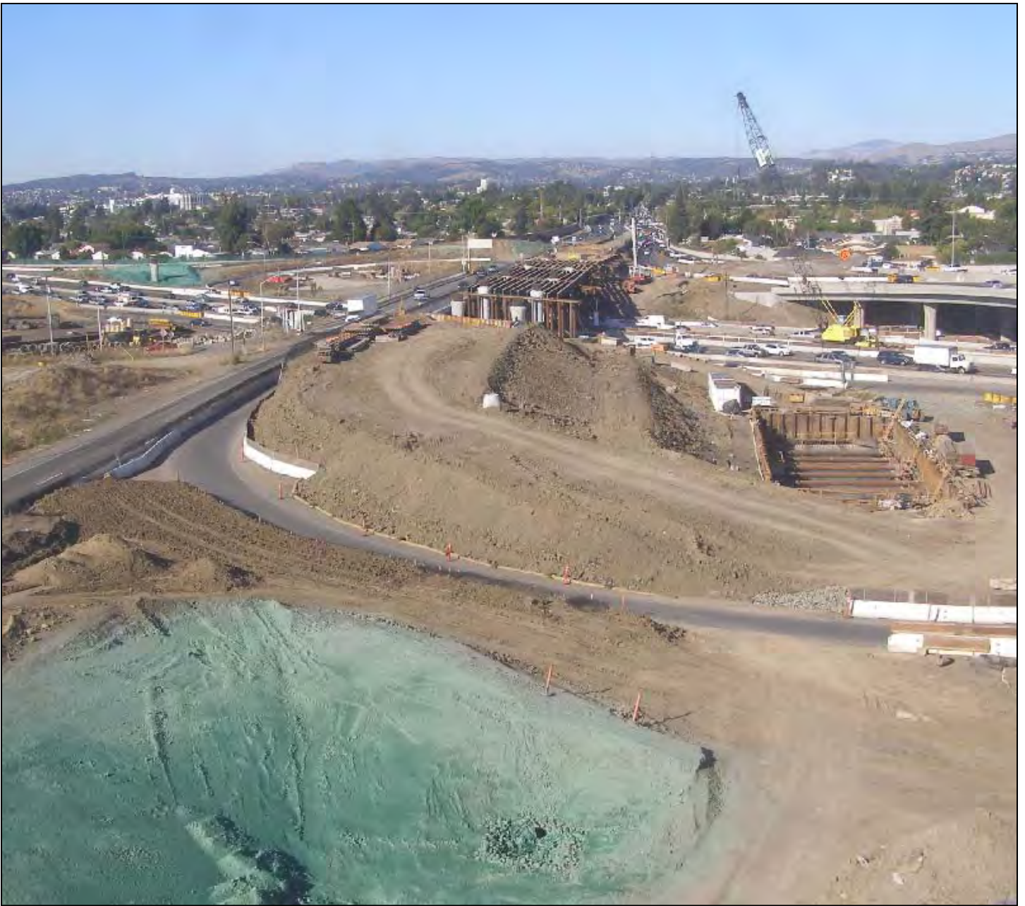
92/880 Site Preparation of New Route 92 and Interstate 880 Separator
