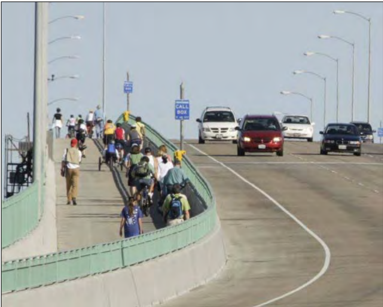
Benicia-Martinez Bridge Pedestrian/Bicycle Pathway Opened to The Public
