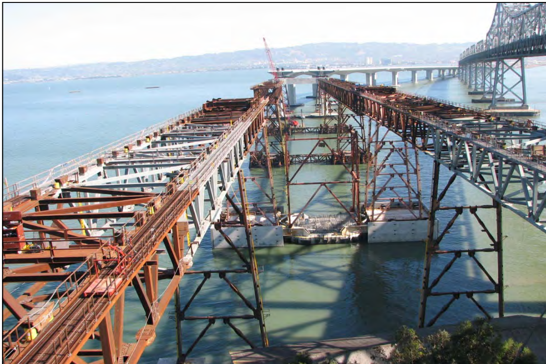
SAS Westbound and Eastbound Temporary Support Structures Looking East
