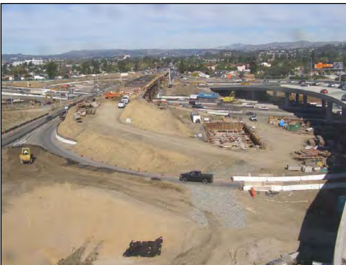
Site Preparation for New Route 92 and Interstate 880 Separator
