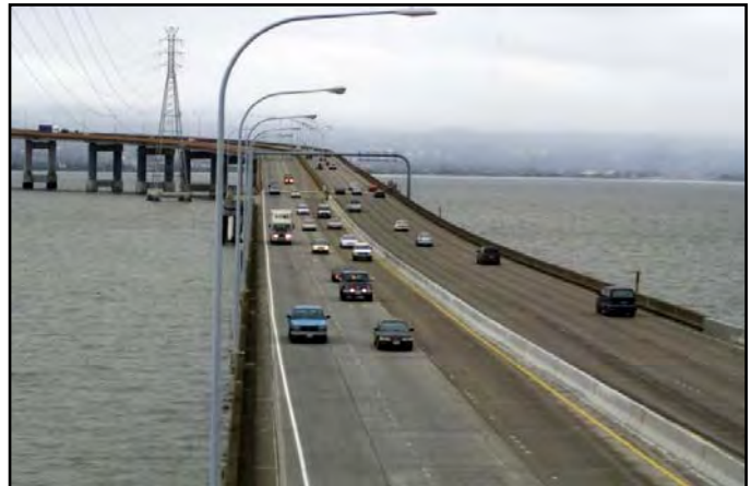
High-Rise Section of San Mateo-Hayward Bridge
