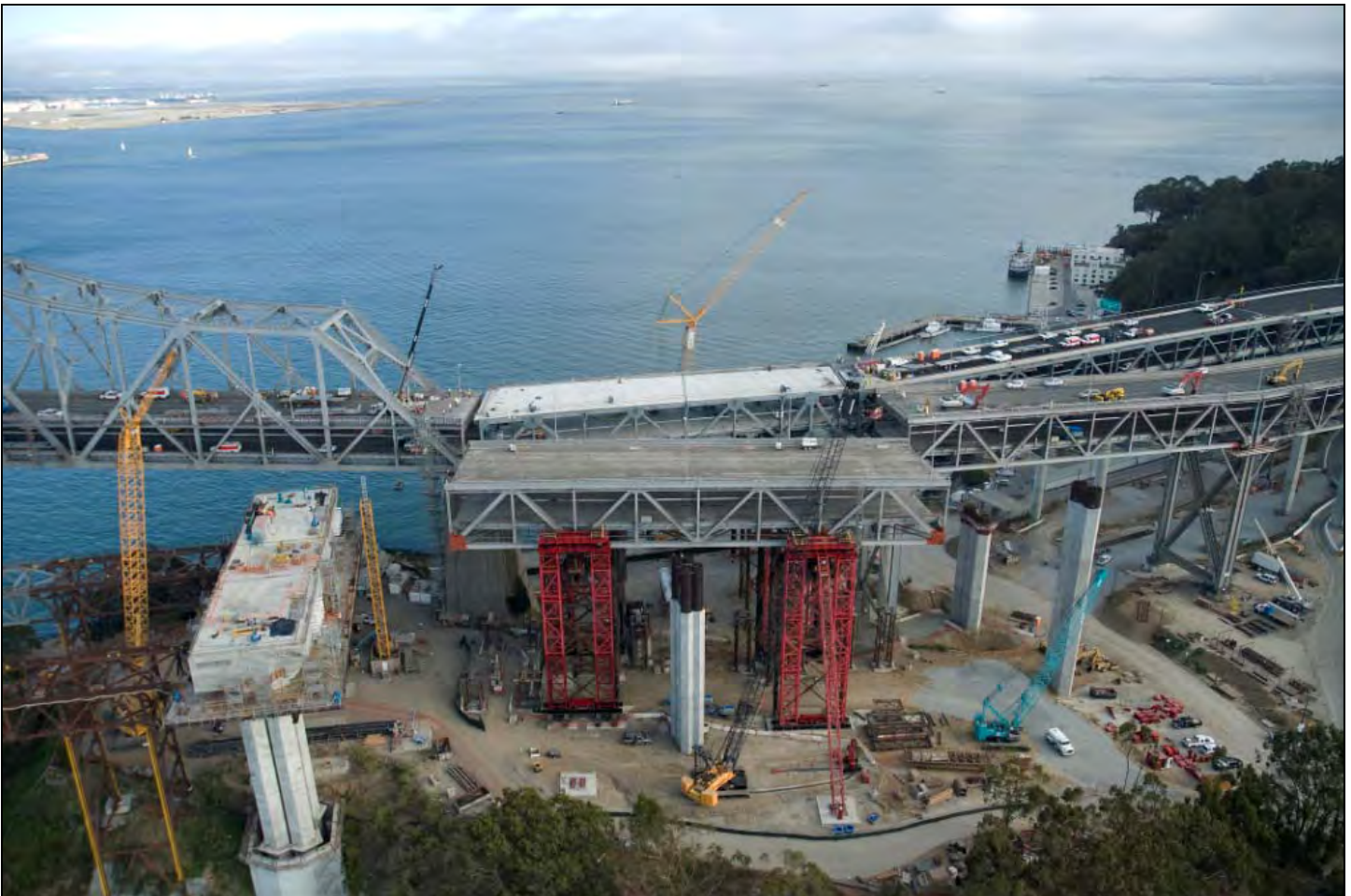
Overview of YBITS Advanced Column Work in Progress
