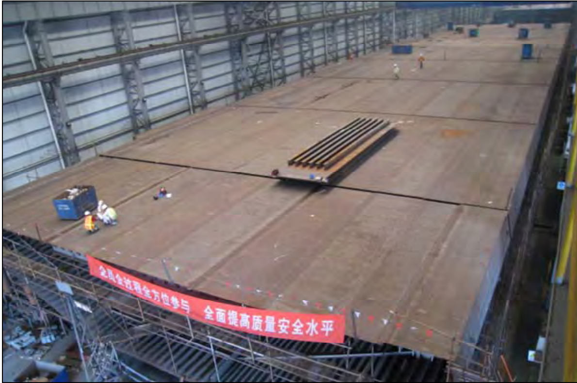
SAS OBG Lift 9 and 10 East-Line Assembly
