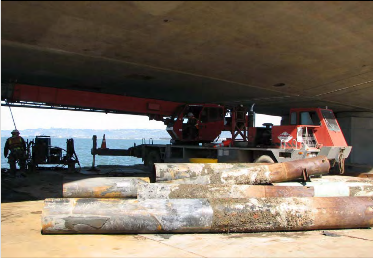
Oakland Touchdown Scaffolding Support Piles Removed
