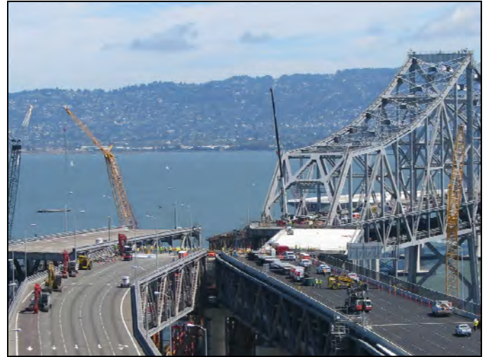
Stage 4 - Roll-In New Truss
