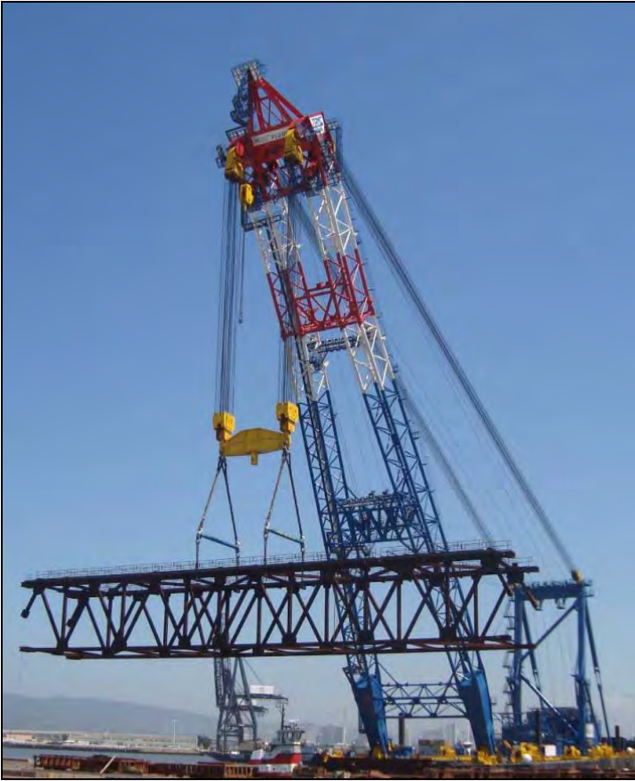
Shear-Leg Barge Crane Lifting a Section of Temporary Support Structure
