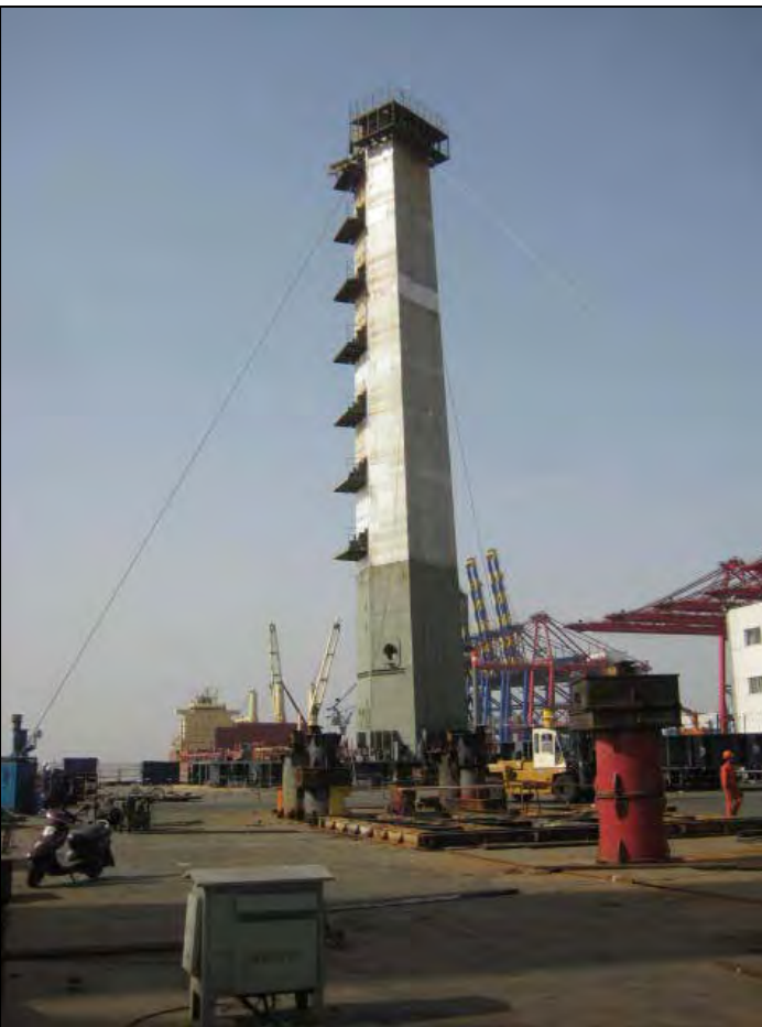
SAS Tower Lift 1 South Shaft in Vertical Position
