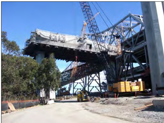
SAS West Elevation of W2
