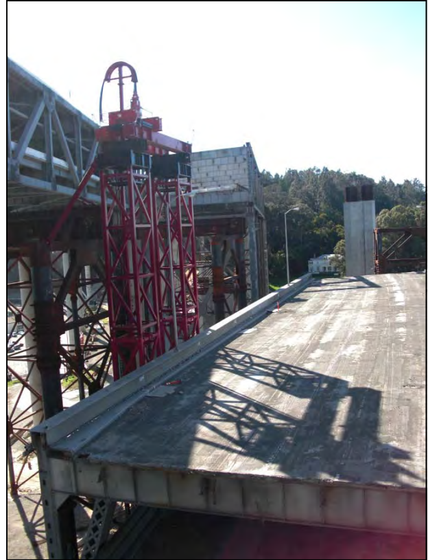
Existing Bridge Viaduct YB4 Span Lowered and Ready for Demolition
