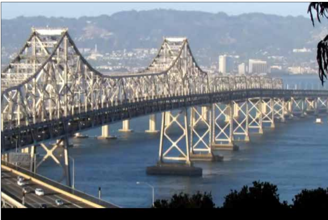
The Former San Francisco-Oakland Bay Bridge Being Prepared for Dismantling
