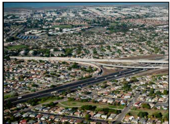
Aerial View of Completed 880/92 Interchange Project
