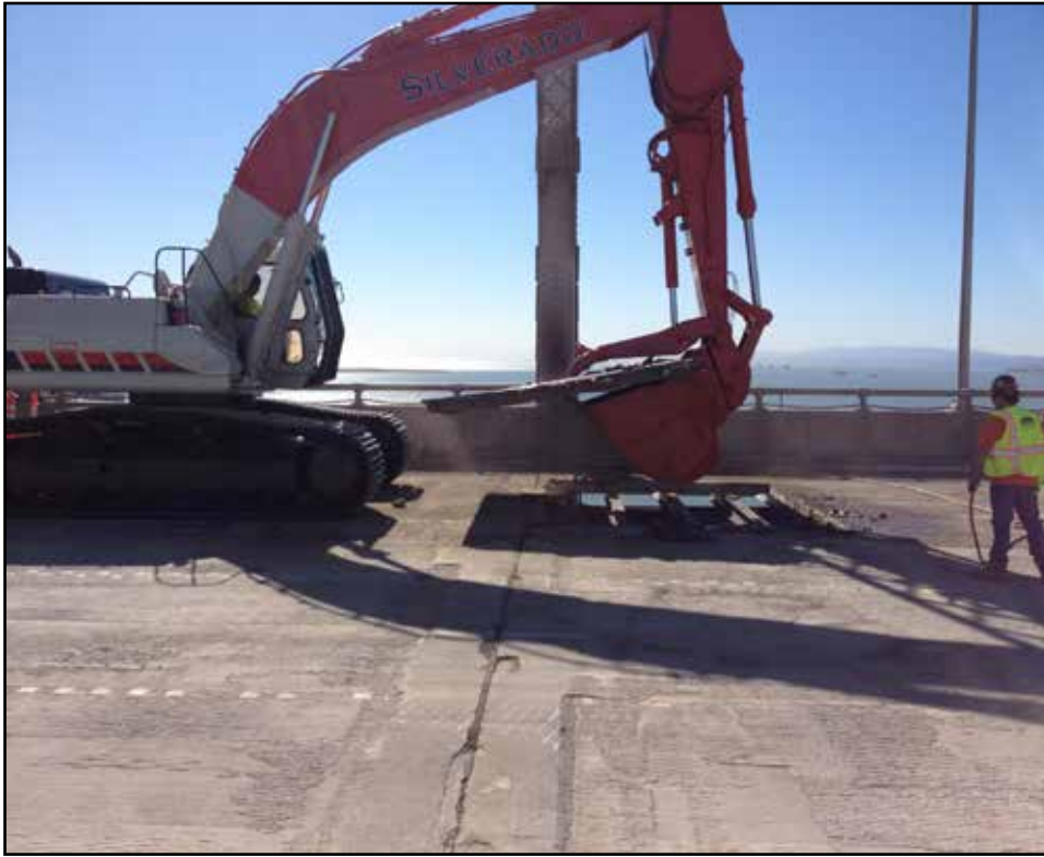
Cantilever Deck Removal in Progress westbound
