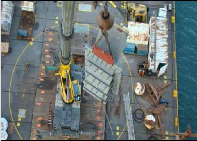
Self-Anchored Suspension Bridge Lower Saddle Installation at E2 Shear Key Anchorage
