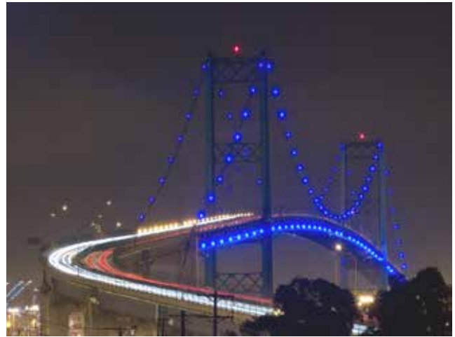
Los Angeles-Vincent Thomas Bridge
