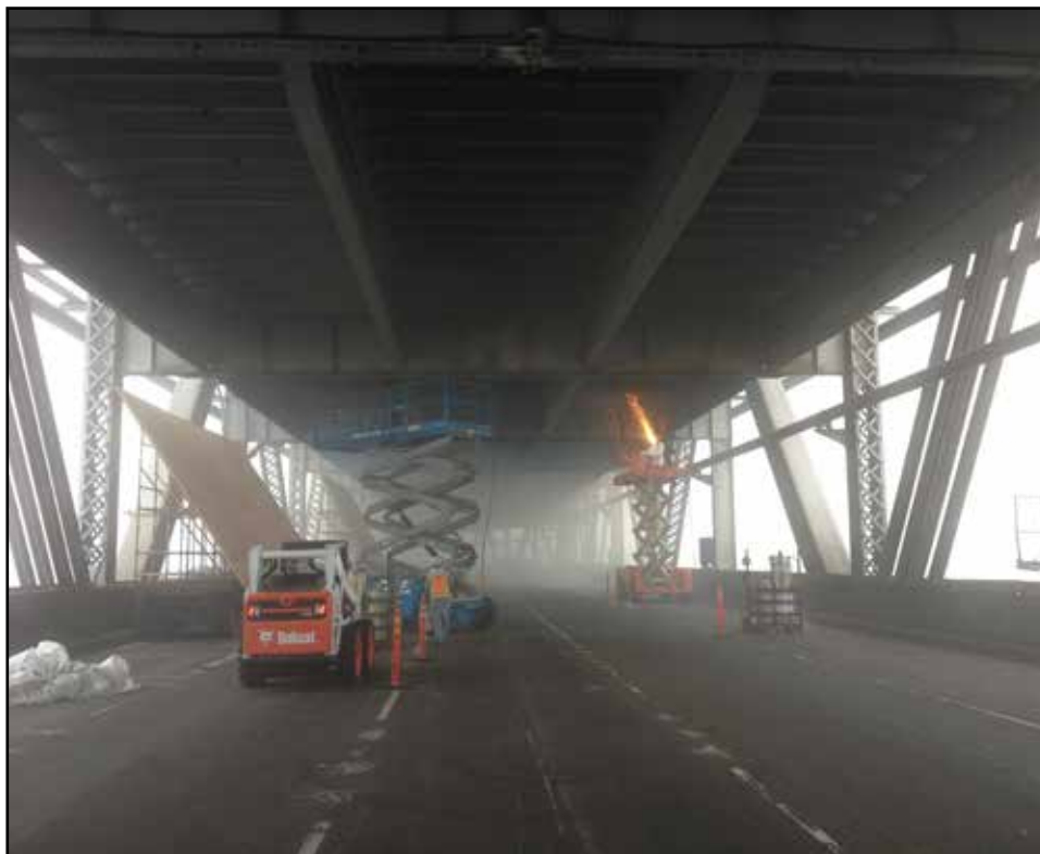
Cantilever Deck Removal in Progress eastbound
