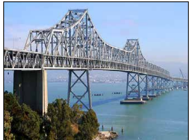
The existing East Span Cantilever Section of the San Francisco-Oakland Bay Bridge to be Dismantled after Seismic Safety Opening of the New Bridge
