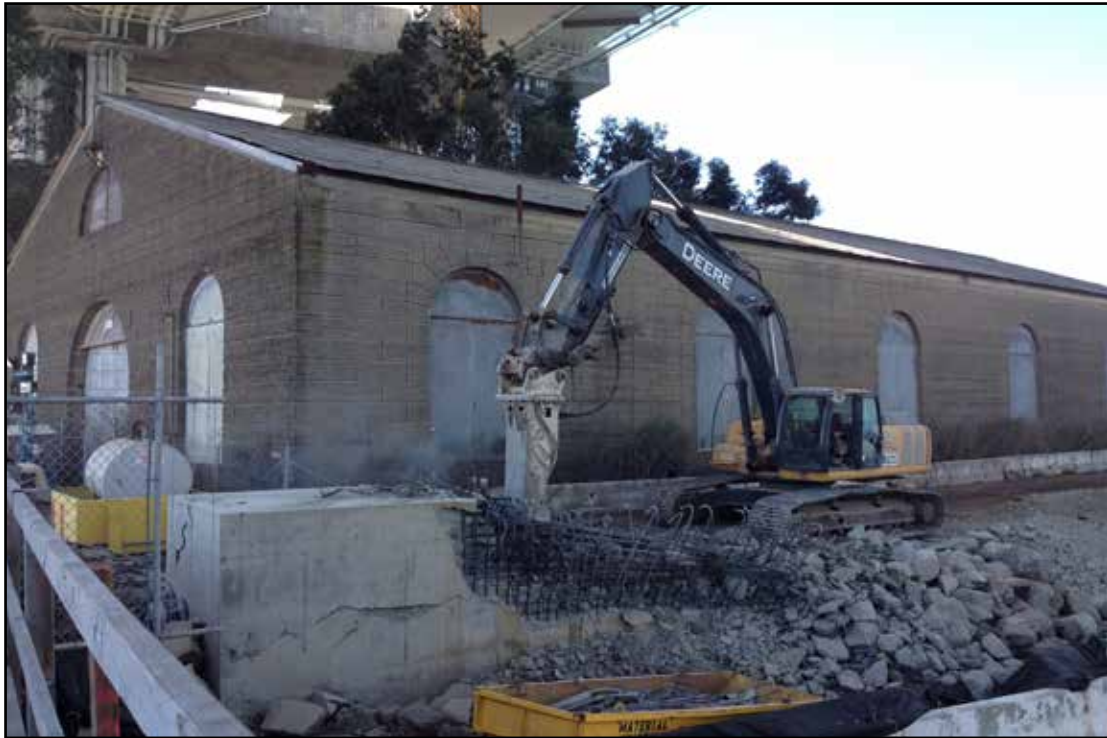
Demolition of the Temporary Truss Foundation
