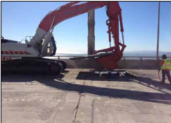
Deck Removal in Progress on the Old San Francisco-Oakland Bay Bridge
