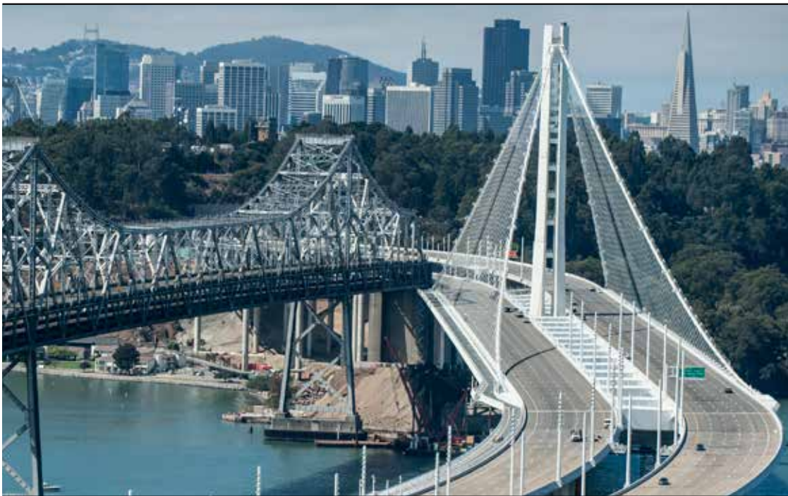
New Self-Anchored Suspension Span
