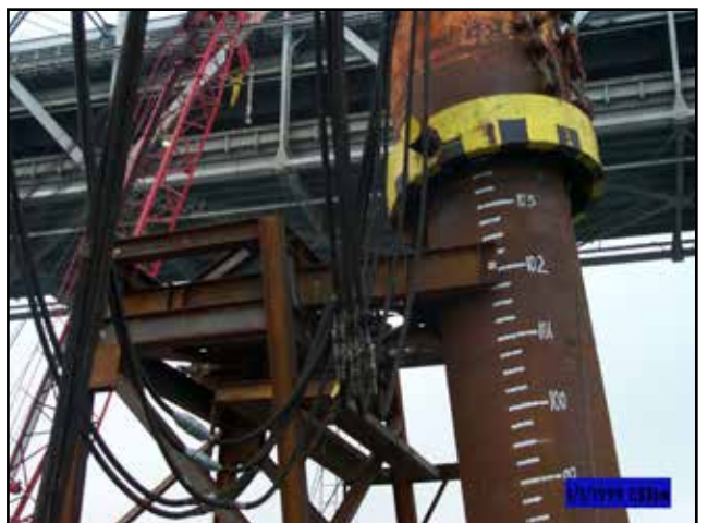
Battered Pile Installation Demonstration
