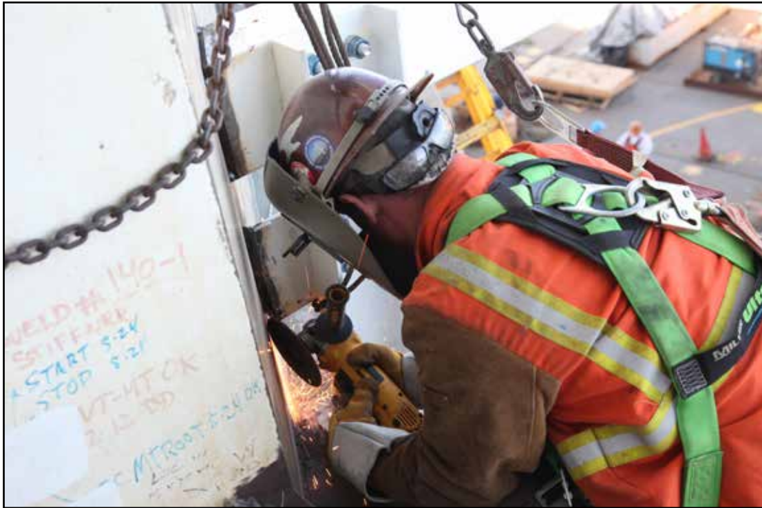
Welding and Grinding Elevator Base Support to Tower Skin
