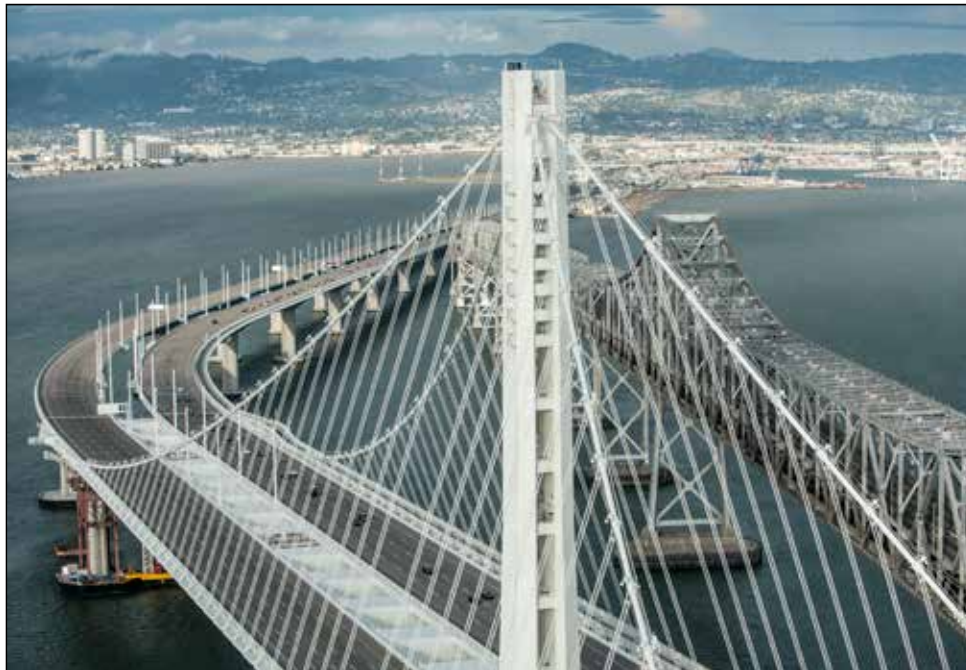
The New San Francisco-Oakland Bay Bridge Self-Anchored Suspension Span with Old Cantilever Bridge on right
