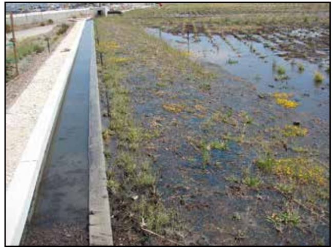
Stormwater Retention Basin
