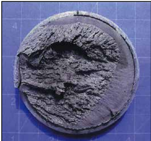
Cross Section of an E2 Shear Key Broken Bolt
