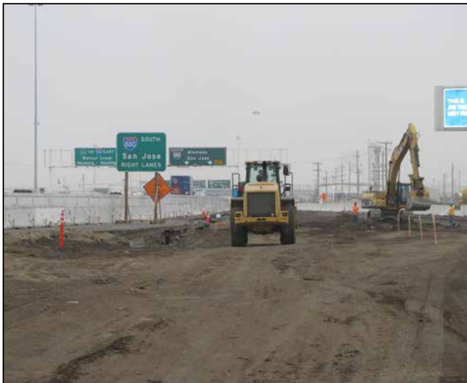
OTD #2 Permanent Bike Path Progress Looking east
