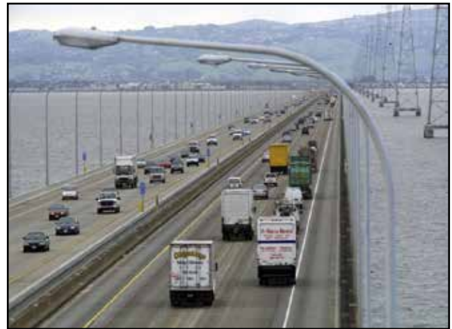
Widening of the San Mateo-Hayward Bridge Trestle on left
