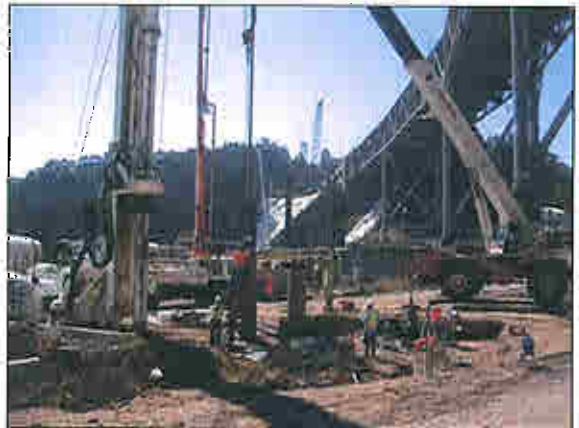
Drilling for CIDH piles for Bent 53
