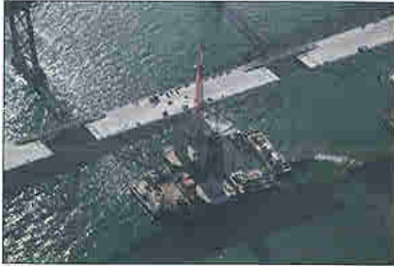
Pier Column construction of the Westbound Skyway
