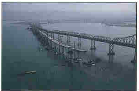
Aerial View of Skyway Construction (looking east)
