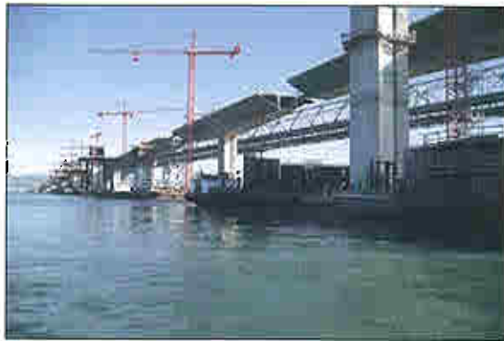
Skyway Construction-Water Level View
