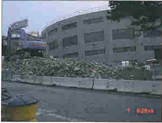
Harrison St. Off-ramp Demolition 1
