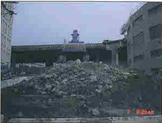
Harrison St. Off-ramp Demolition 3
