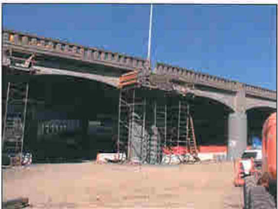
Demolition of Frame 7U North & 8U North over First St. On-ramp 2
