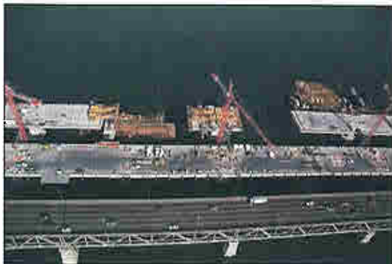
Aerial View of East-bound - West-bound Roadway Section (looking west) 2
