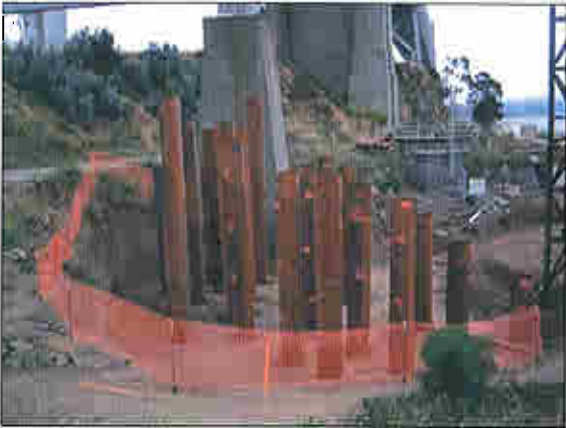
Piles for Bent No. 52
