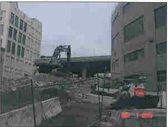
Harrison St. Off-ramp Demolition 5
