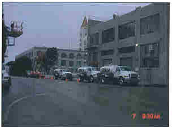
Harrison St. Off-ramp Demolition 4
