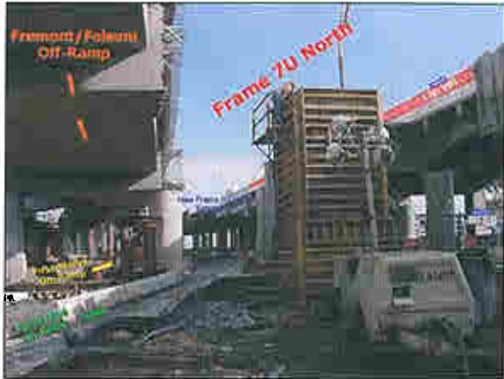
New Frame 7U north False work at bents 20 and 21
