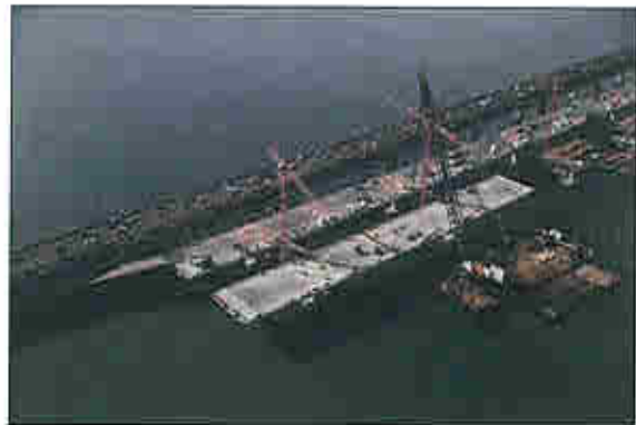
Aerial View of Pier 15 & 16
