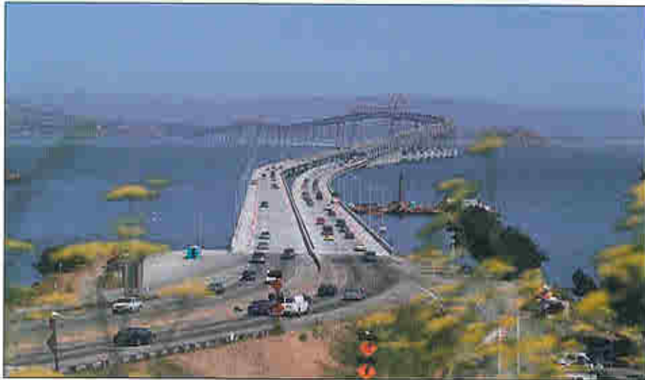
Richmond-San Rafael Toll Bridge
