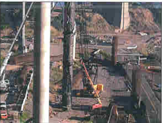
SoSoDet - Construction of columns for the viaduct portion of the Temporary Bypass Structure (TBS) adjacent to the U.S. Coast Guard Road on Yerba Buena Island
