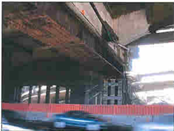
Temporary Support Frame (Super Bent at Bent #43) 4
