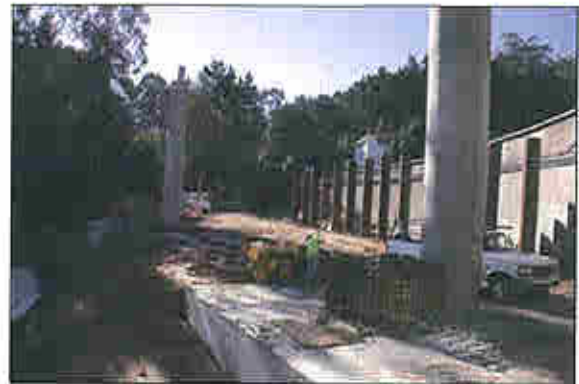
Footings and Pier Columns for Bent 48
