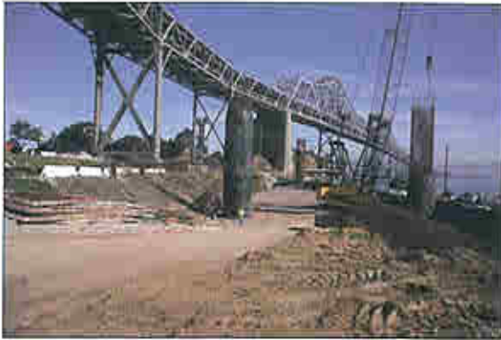
Pier Column Construction for Bents 50 and 51
