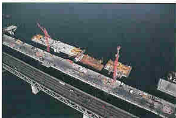
Aerial View of East-bound - West-bound Roadway Section (looking west) 3
