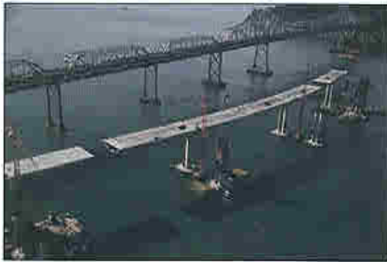
Aerial View of Pier 3,4 & 5 (looking east)
