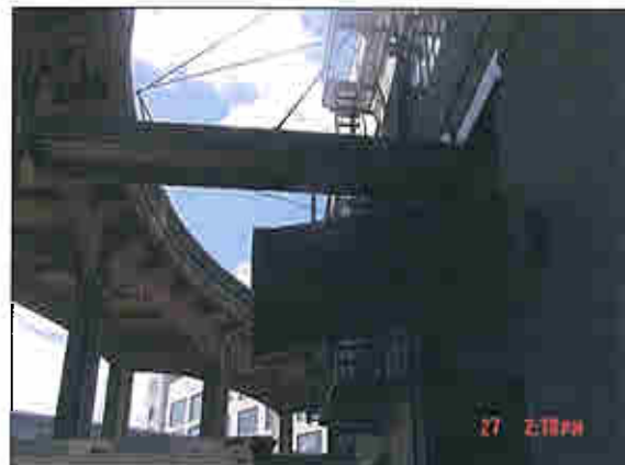
Harrison St. Off-ramp Pre-demolition 1
