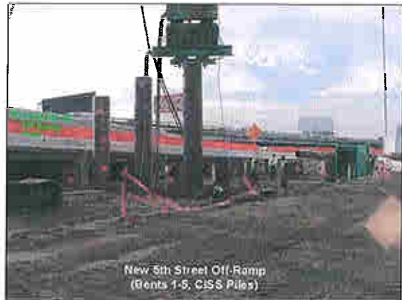
New 5th Street off ramp Bents 1 thru 5, CISS Piles
