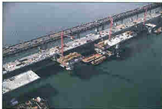
Aerial View of East-bound - West-bound Roadway Section (looking west) 1
