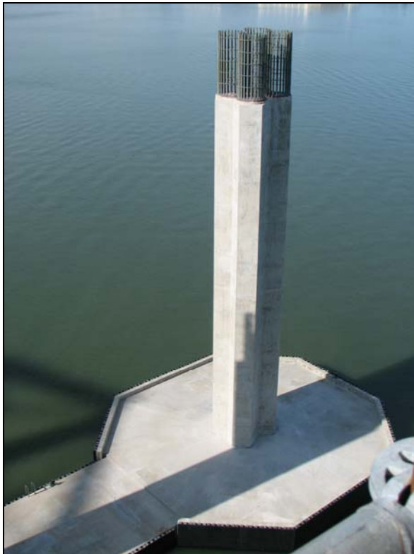
SAS E2-T1 - Completed E2 Column Westbound
