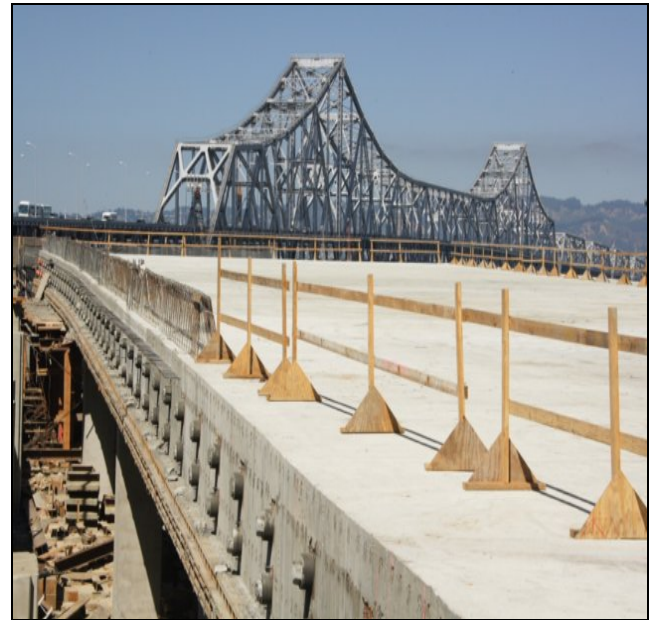
East Span Deck Replacement
