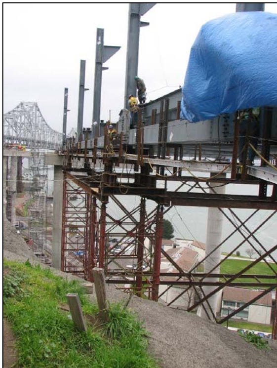
YBID – Detour Viaduct Erection
