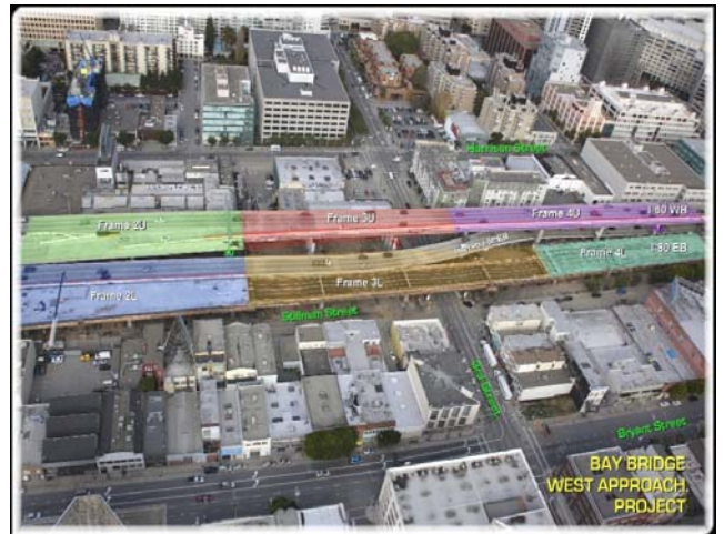
West Approach - I-80 EB WB – 4 th St. to 2 nd St.
