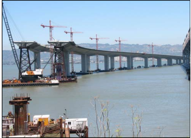
Skyway - Bridge Looking East from Yerba Buena Island
