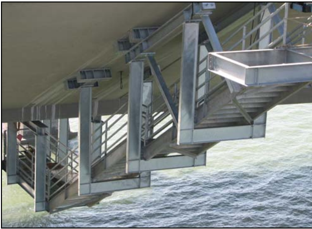
Skyway - Stairs Leading to the Substation
