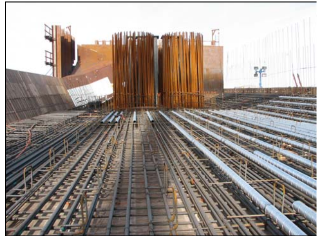
SAS - W2 Steel Reinforcement
