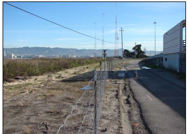
Stormwater - Radio Road Planting
