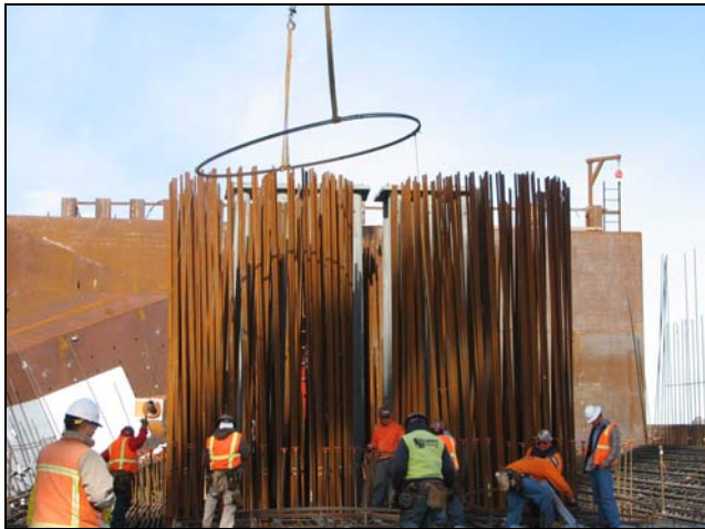
SAS - W2 Steel Reinforcement
