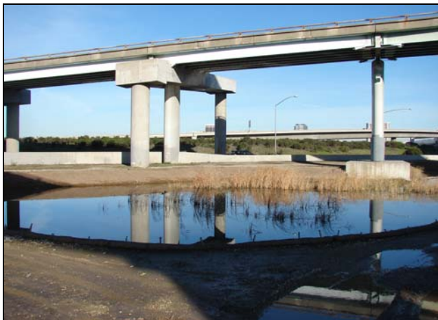
Stormwater - Forebay Location 5
