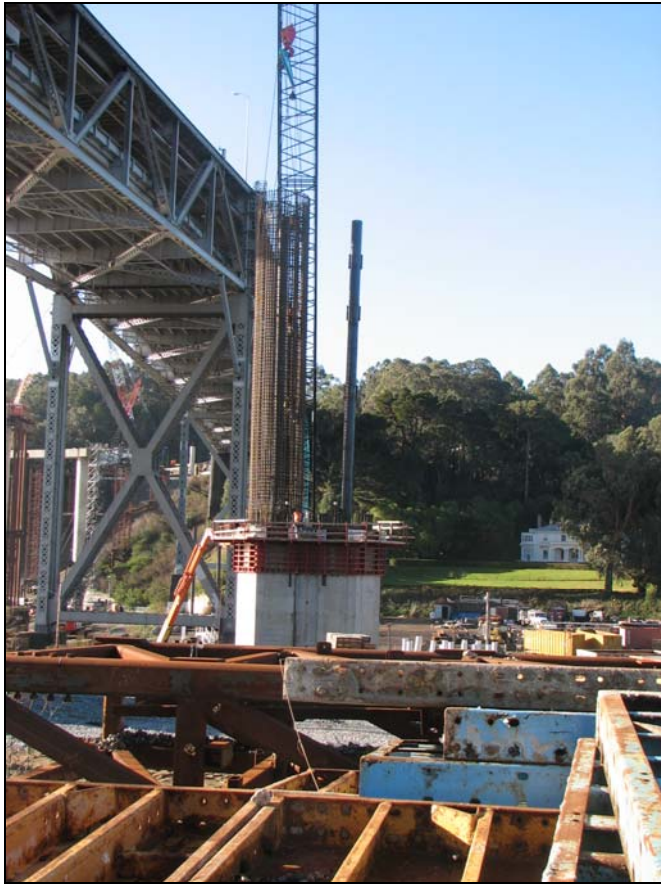
YBID – Bent W4L Construction YBI Advanced Work
