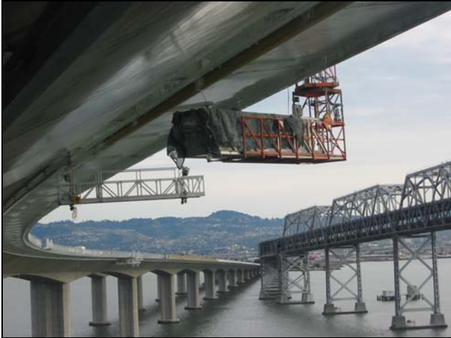
Skyway - Underside Painting
