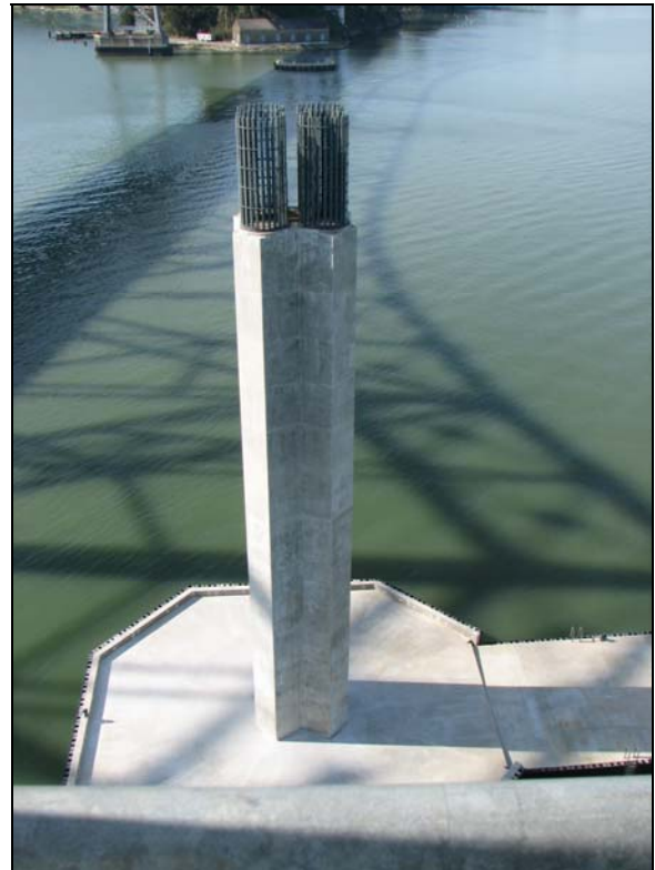
SAS E2-T1 - Completed E2 Column Eastbound T1 Foundation
