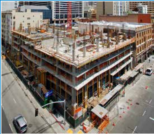
The Eddy and Taylor Family Housing Project in Progress
