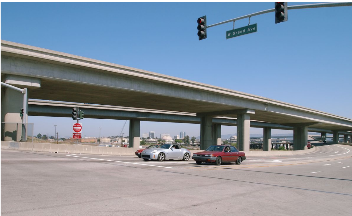
Photo 6. Looking north toward the EBMUD wastewater treatment facility at the Frontage Road and West Grand Avenue intersection.
