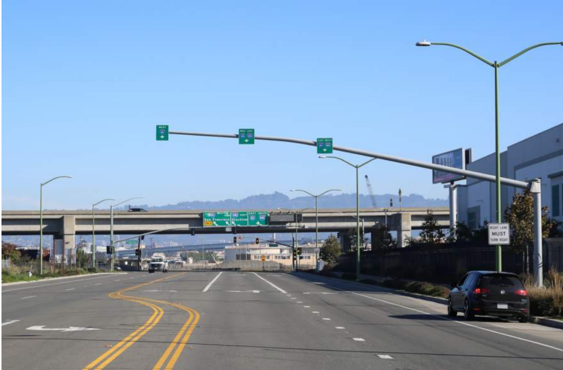
Existing Conditions. View of West Grand Avenue from Maritime Street.
