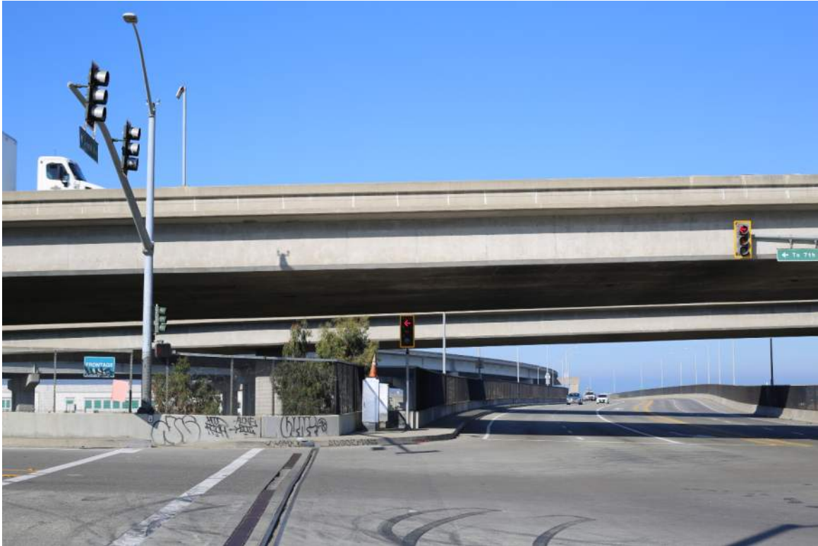
Existing Conditions. View of West Grand Avenue from Frontage Road.
