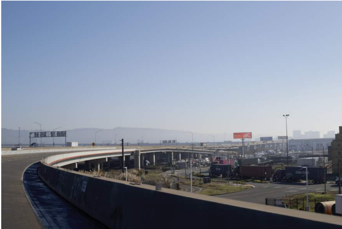
Existing Conditions. View eastward from I-80.
