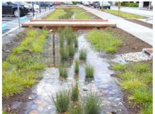
Photo 4: Rain garden and stormwater planters in curb extensions, Donnelly Avenue, Burlingame Photo: City of Burlingame
