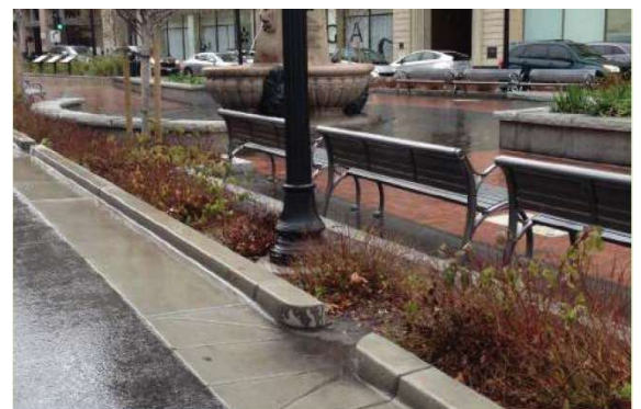
Photo 2: Stormwater planter, Latham Square, Oakland Photo: CD+A
