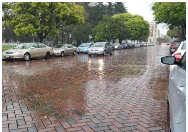
Photo 5: Allston Way pervious pavement, Berkeley Photo: Friends of Five Creeks
