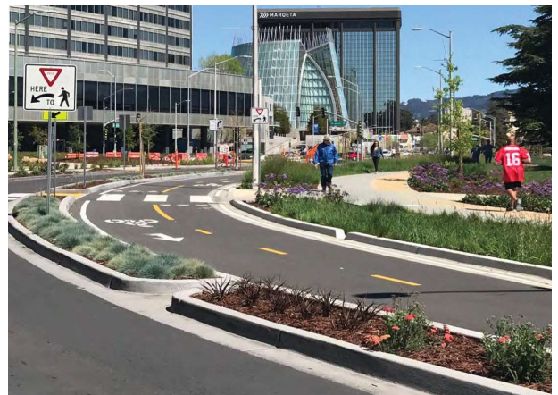
Photo 3: Stormwater planter, Harrison Street, Oakland Photo: CD+A
