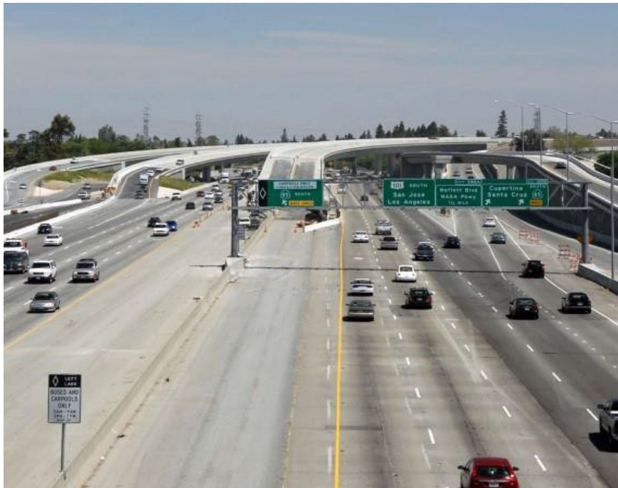
Pictured: 101/SR85 interchange in Mountain View
