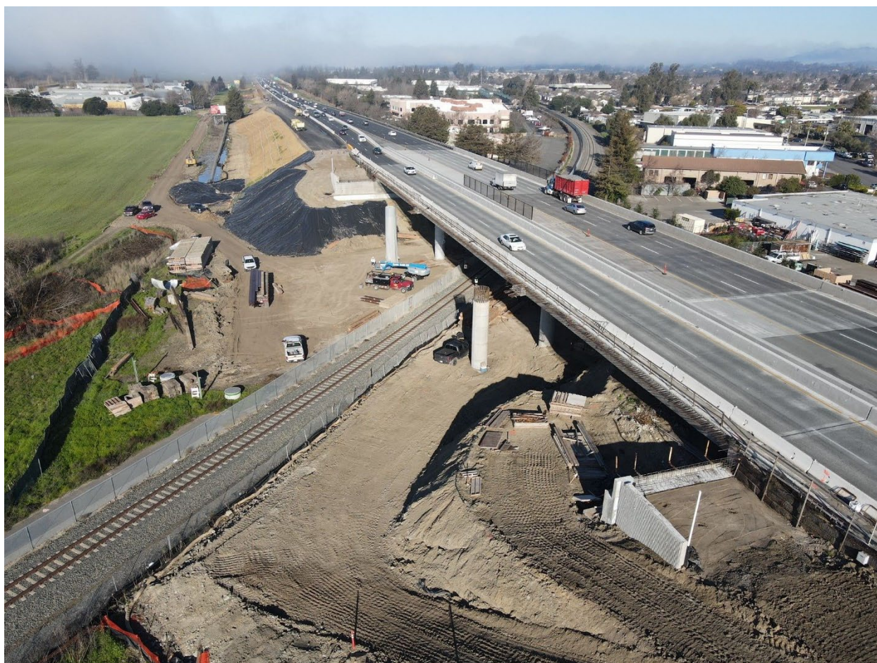
Replacement of the North Petaluma Overhead, Highway 101 over SMART Under construction in 2022
