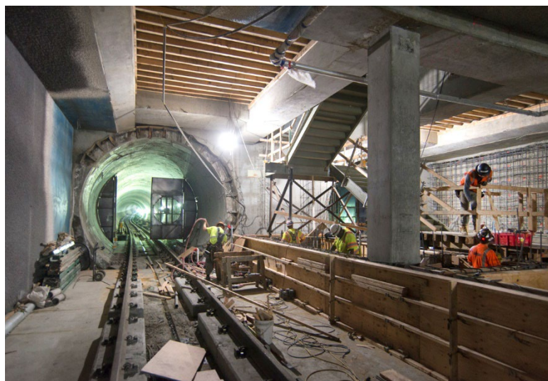
Pictured: Construction of SFMTA's Central Subway Project
