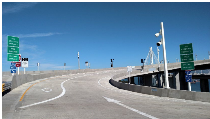
Pictured: WB I-80 on- and off-ramps that connect Yerba Buena Island and Treasure Island to the eastern span of the Bay Bridge.
