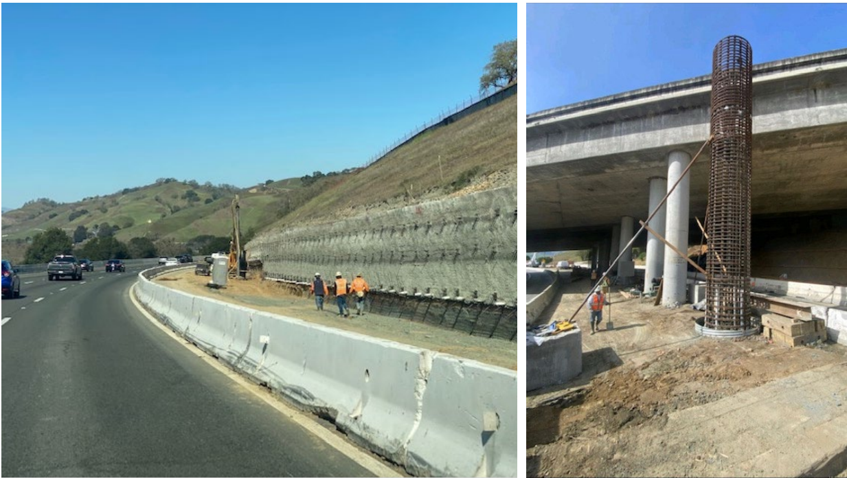
Pictured: I-680/84 Interchange Improvements project under construction
