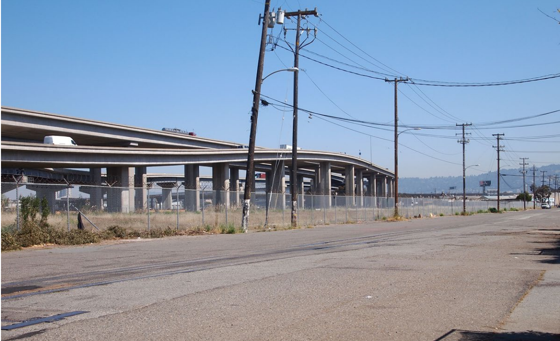
Photo 8. Looking northeast toward the rail line and elevated freeway connectors from Wood Street.
