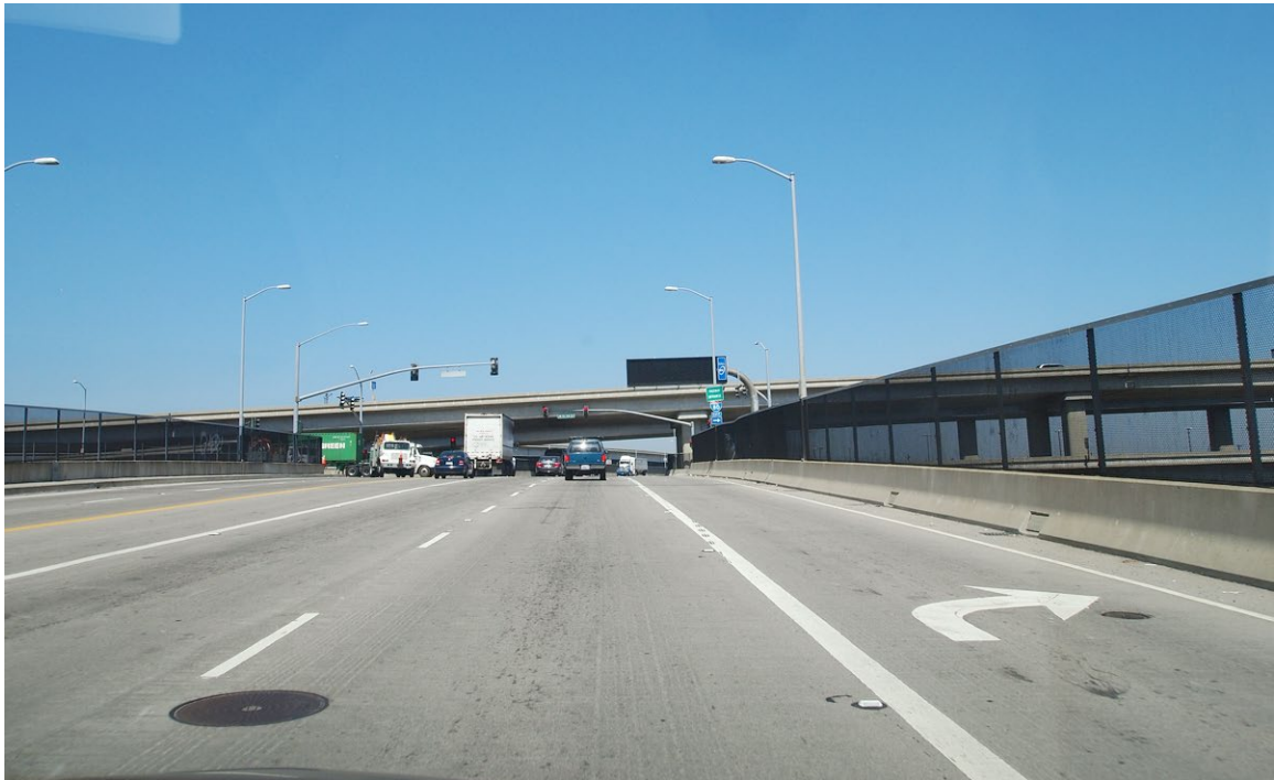
Photo 4. Looking northwest toward Frontage Road and I-80 connection overpass from West Grand Avenue.
