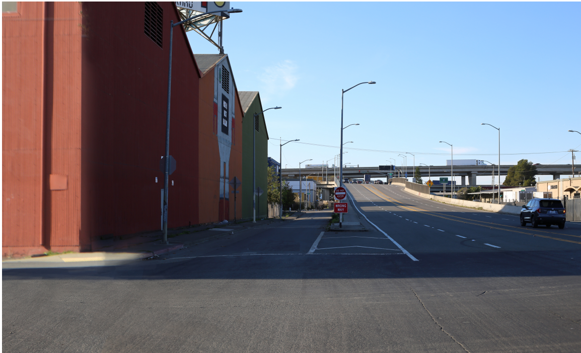
Existing Conditions. View of warehouse on West Grand Avenue alley.
