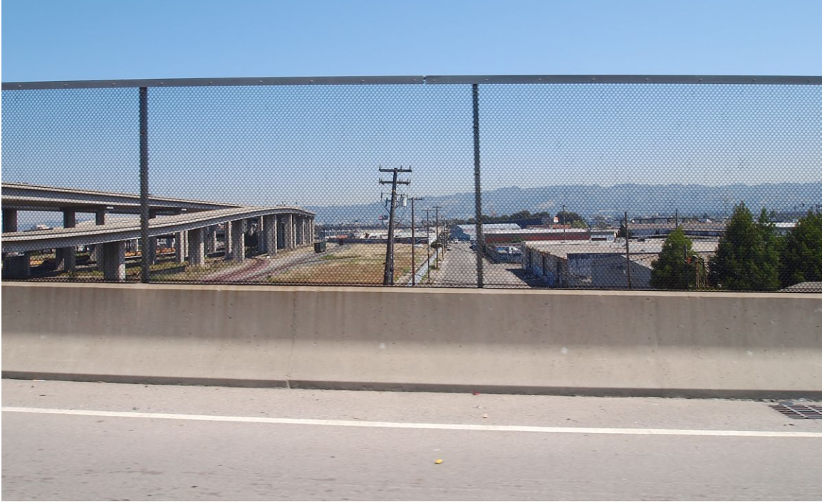
Photo 7. Looking northeast toward elevated freeway connectors, the rail line, western edge of Oakland, and Berkeley Hills from West Grand Avenue.
