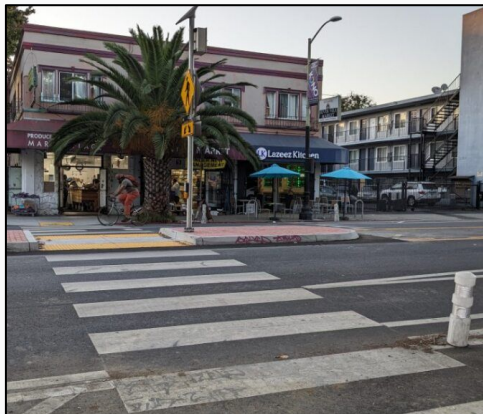
Pedestrian Refuge Island and High Viz Crosswalk
