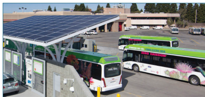
AC Transit’s on-site energy stations enable zero-emission buses to be refueled at rates comparable to refueling diesel buses. (Photo: courtesy of AC Transit)
