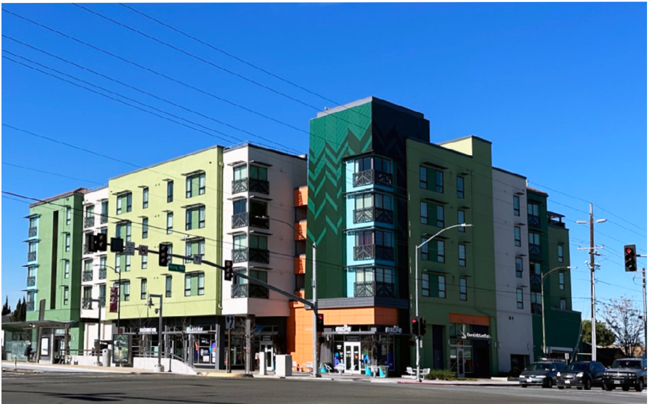
Affordable housing apartment building, Santa Clara County
