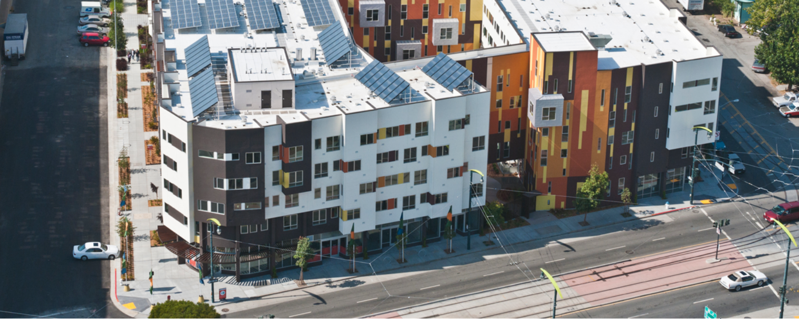
Armstrong Place Senior Housing and Armstrong Townhomes in San Francisco Photo by Steve Proehl, courtesy of BRIDGE Housing
