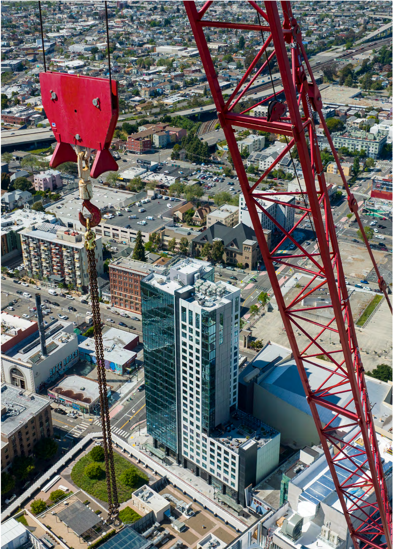
High-rise apartment, Oakland Photo: Karl Nielsen
